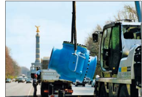
Fig. 7.4.3-05: DN 1000 ball valve for a wastewater pressure pipeline
