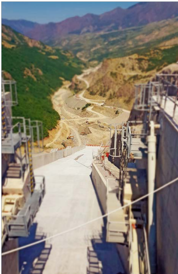
A view from the dam down to the emergency spillway.
