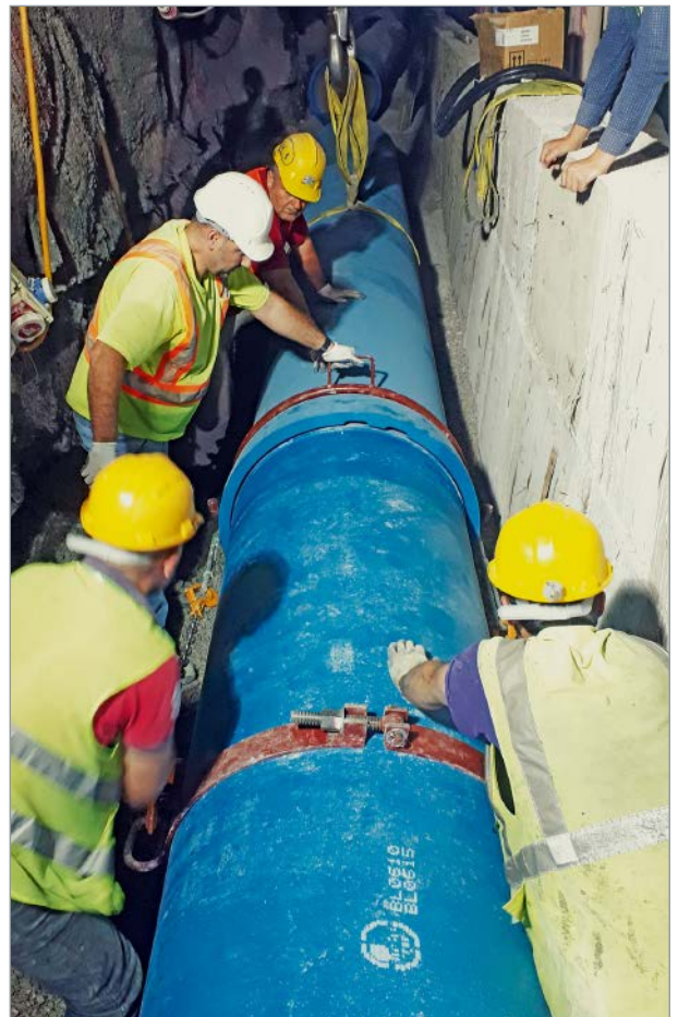
An assembly team installing a DN 800 pipe.
