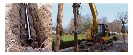
♦ In the Vorarlberg district of Hard am Bodensee the development of a construction area has necessitated the installation of a new sewage pipeline. The unfavourable subsoil conditions consisting of clay, fen and peat determined the choice of pipe material. Because of the flatness of the land the pipeline was able to be laid in nominal diameters DN 150,
