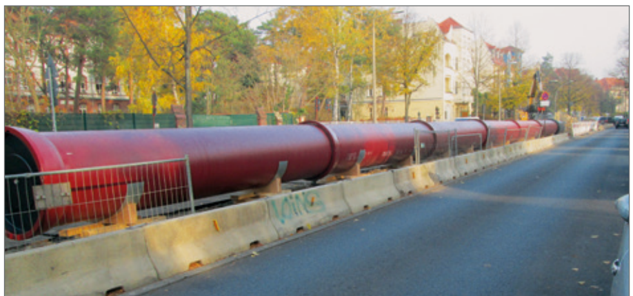
Interim pipeline in Hermann-Hesse-Straße
