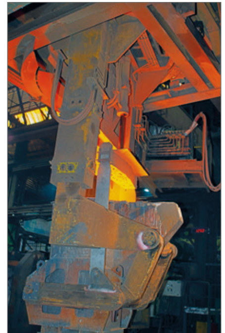
Casting ladle on the overhead crane.
