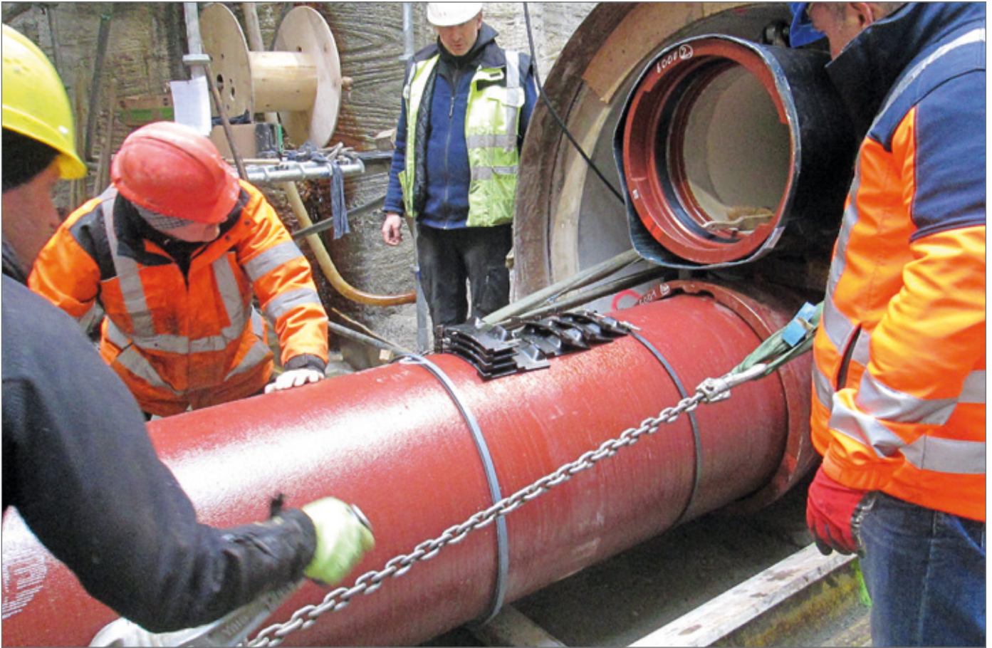
Installation of ductile iron pipes with restrained joints.
