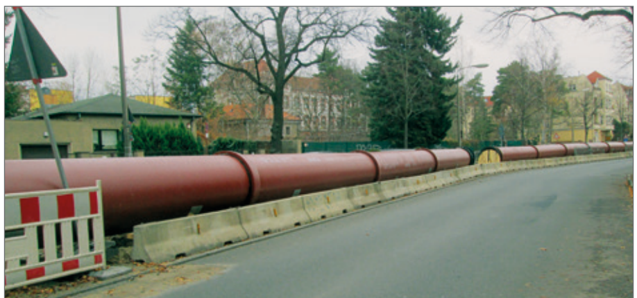
Section-by-section tightness testing of the interim pipeline.
