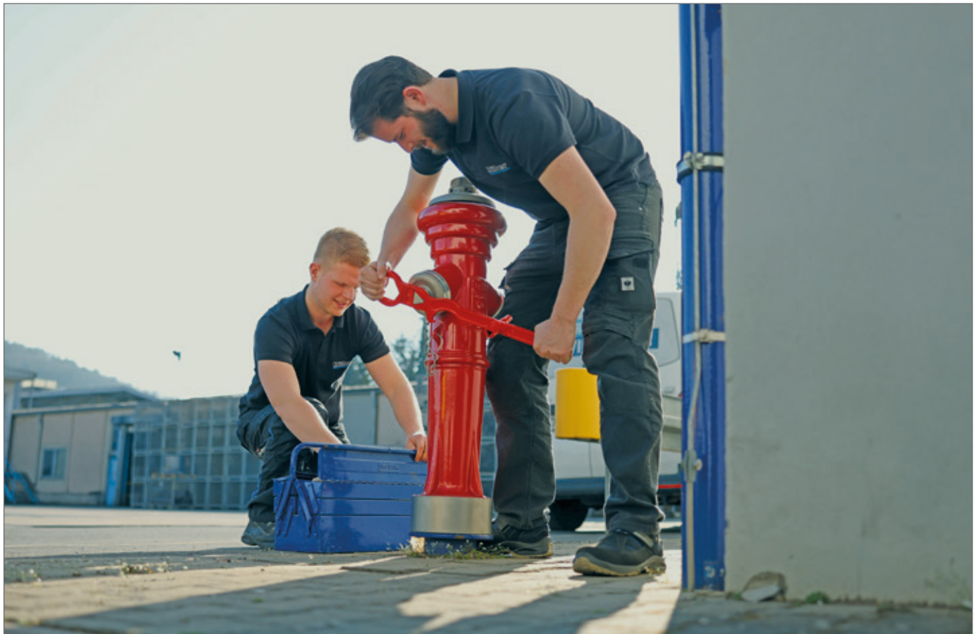
Support for the installation company by expert service teams.
