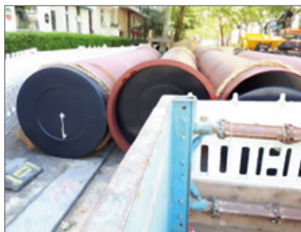
DN 1000 pipe with BLS®-joint in Bergstraße (Steglitz district of Berlin).
