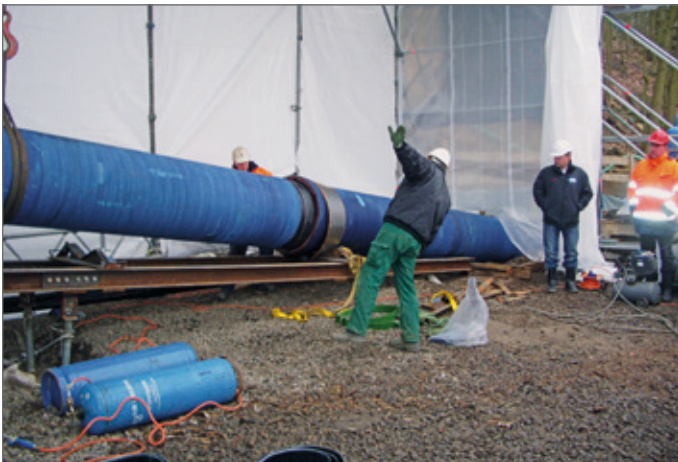
Replacement of the raw water pipeline at the "Schildhorn" wells.
