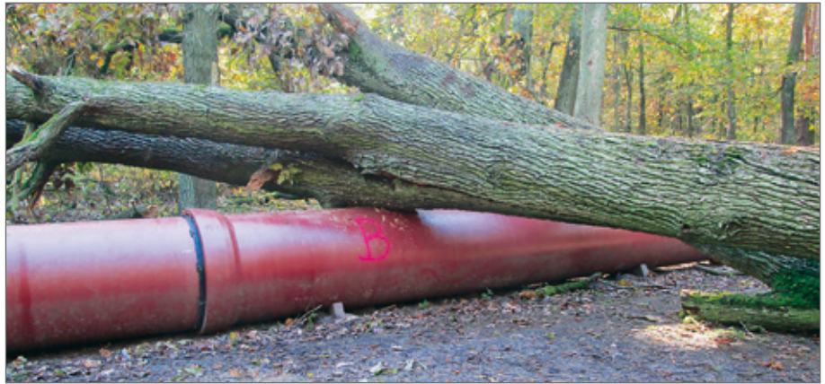
An uprooted oak tree caused no damage to the interim pipeline.
