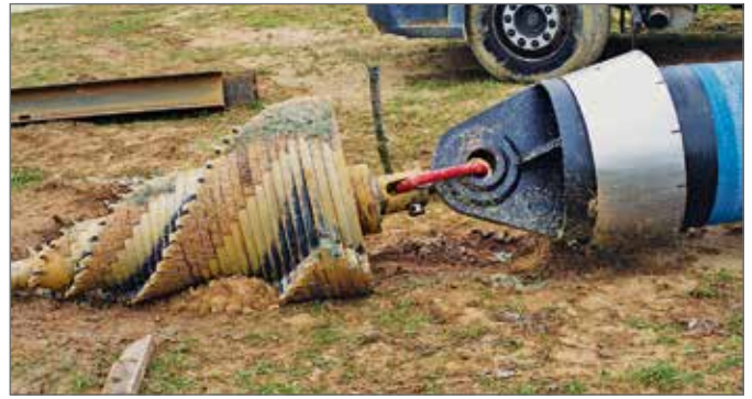
Connection of the upsizing head to the DN 600 pipe pull-in head.
