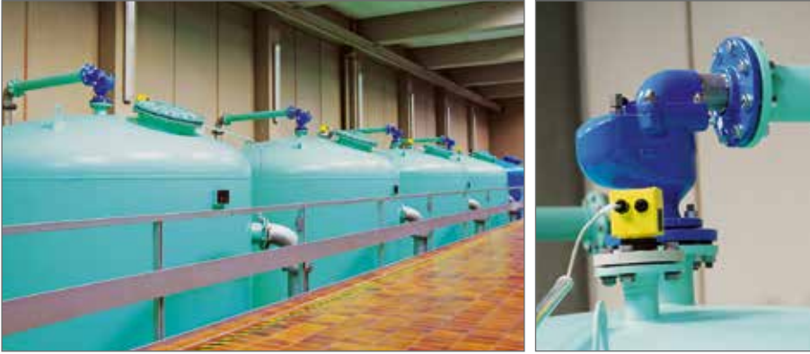
Single-layer filter vessels with TWIN-AIR admission and release valve in position.
