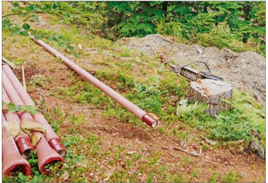
Ductile iron pipes with the VRS®-T restrained push-in joint earn extra points with the abrasion resistance of cement mortar lining, which is guaranteed even at the high flow speeds which occur on steep slopes.
