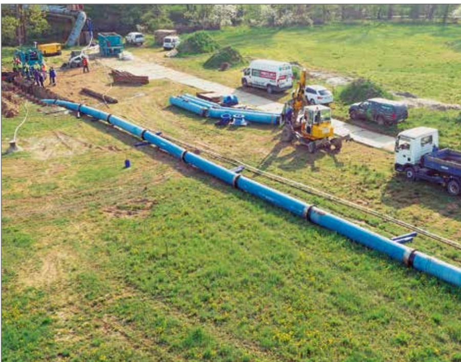
The pipe string was pulled through in one piece.
