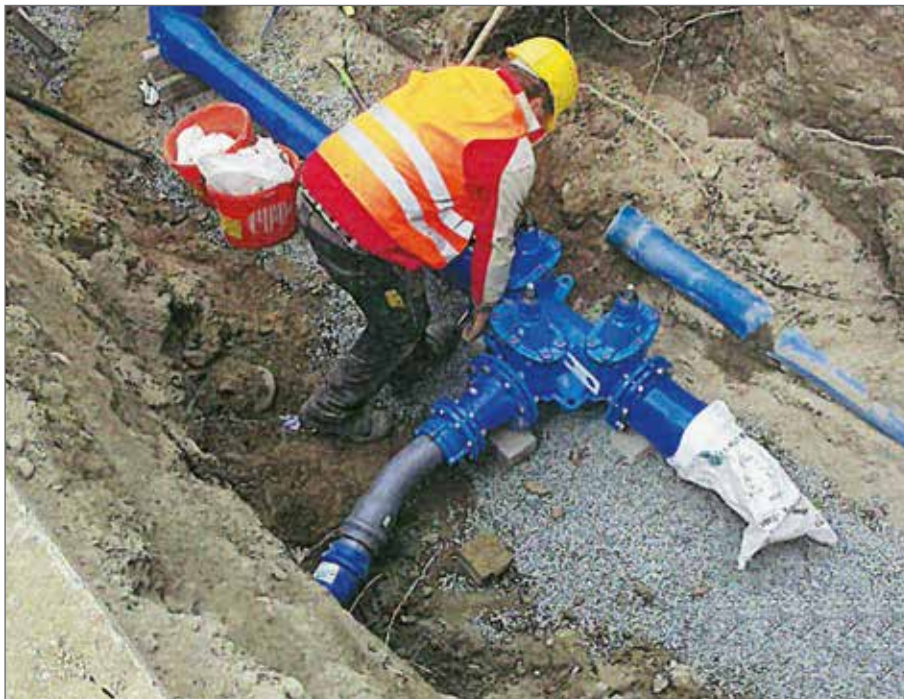
Installation of various valves and hydrants in the piping network.
