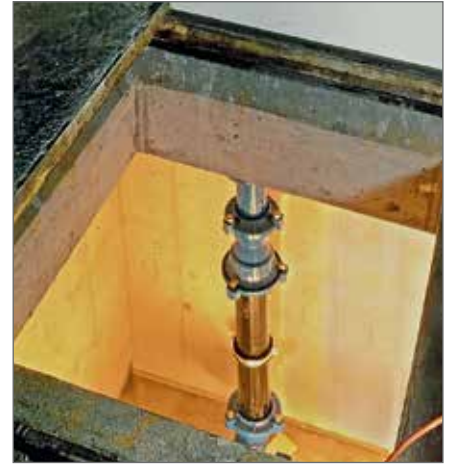
A view from the road area into the hydrant chamber.
