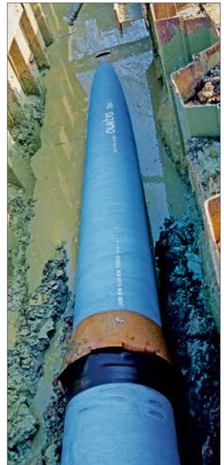
Pulling the pipes into the borehole.
