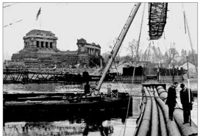
Securing the pipes with steel frames and lowering them to the riverbed.
