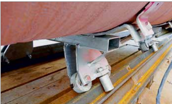
On pre-assembled rails the pipe clamps pulled from the other side roll slowly through the tunnel.
