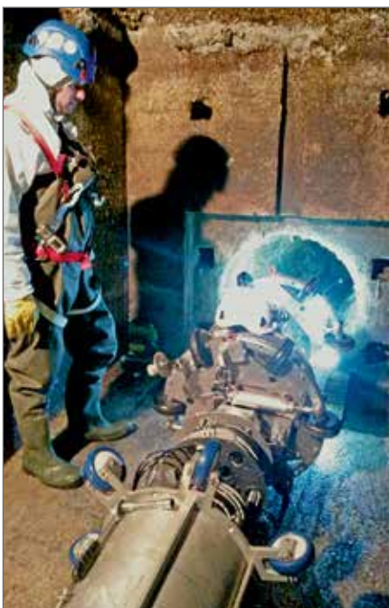
Positioning the scanners at the culvert opening.
