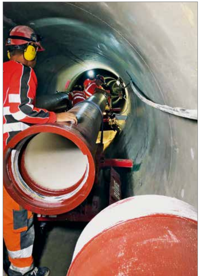
Pipe assembly DN 400 with protective epoxy finishing layer at Industriestraße
