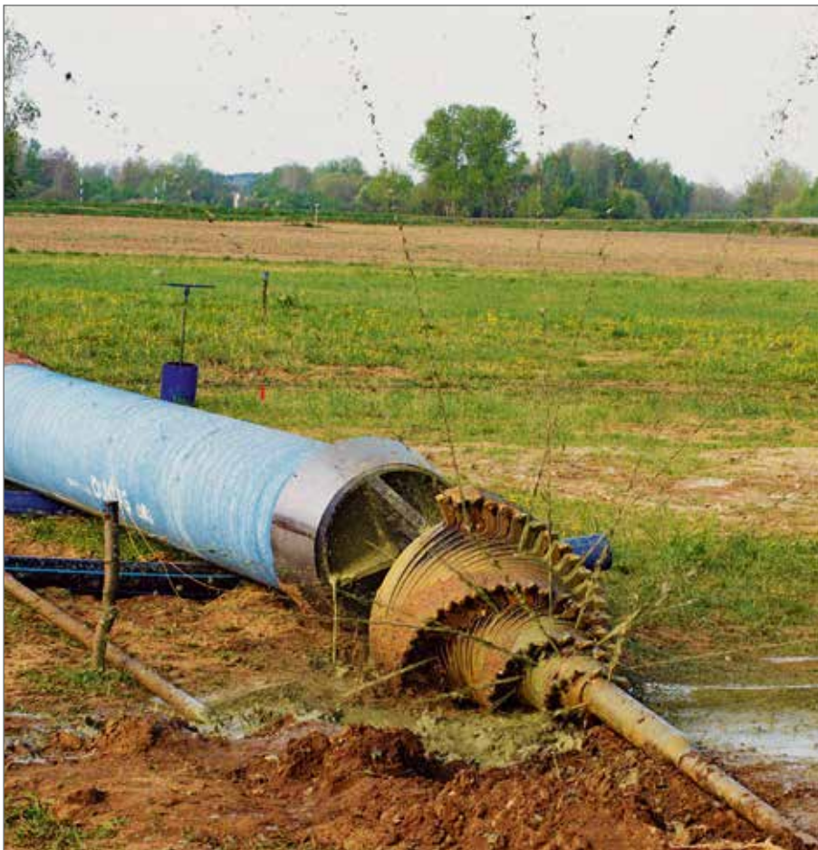
Function testing of the drilling head before pulling in the pipes.
