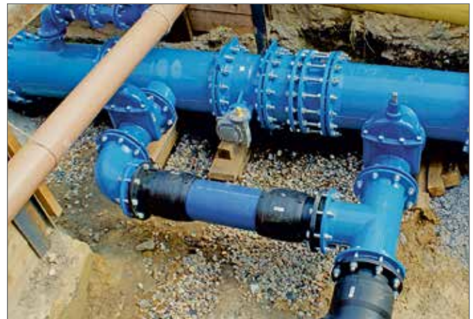
... as well as branches and connections by open-trench installation.
