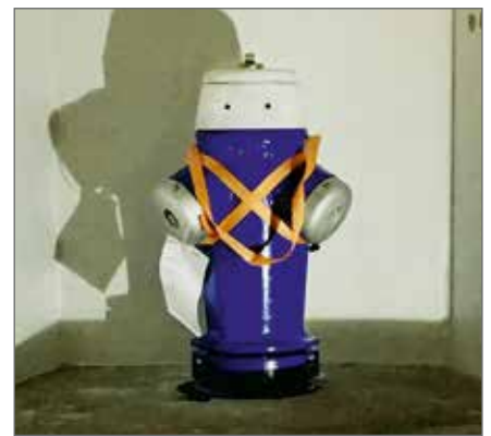
Hydrant recess with HYPLUS hydrant top part installed.
