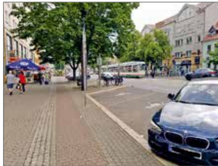
The 2 to 4-lane Halberstädter Straße with its wide pavement area, cycle way, parking strip, trees, tramway and bus traffic before the start of the renovation work.
