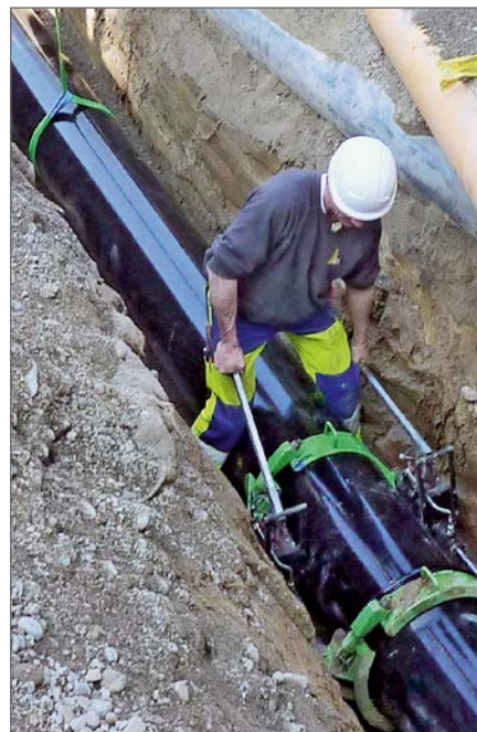
Installation under difficult conditions where pipelines cross
