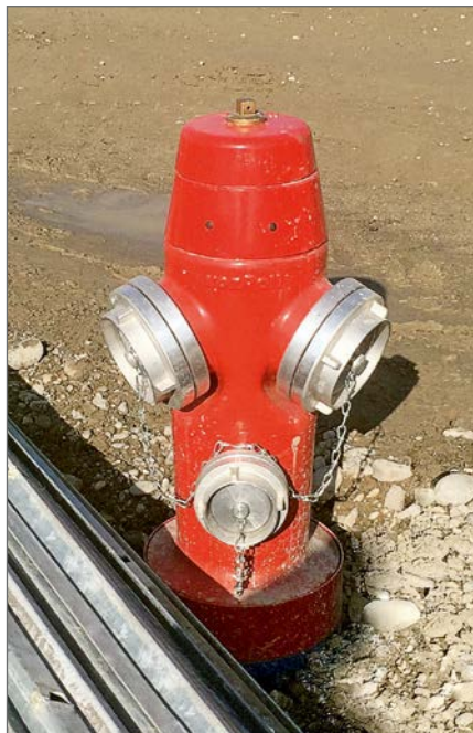
vonRoll high-performance industrial hydrants (Fig. 5530) with Storz 110 mm lateral outlets and Storz 75 mm central outlet
