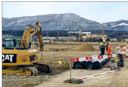
A view northwards across the Luterbach Biogen construction area
