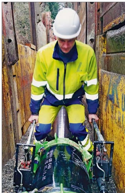
Assembling a HYDROTIGHT push-in joint with hydraulic pipe-laying equipment
