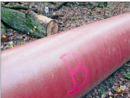
After the oak had been removed there was no sign of damage or even any alteration in the coating
