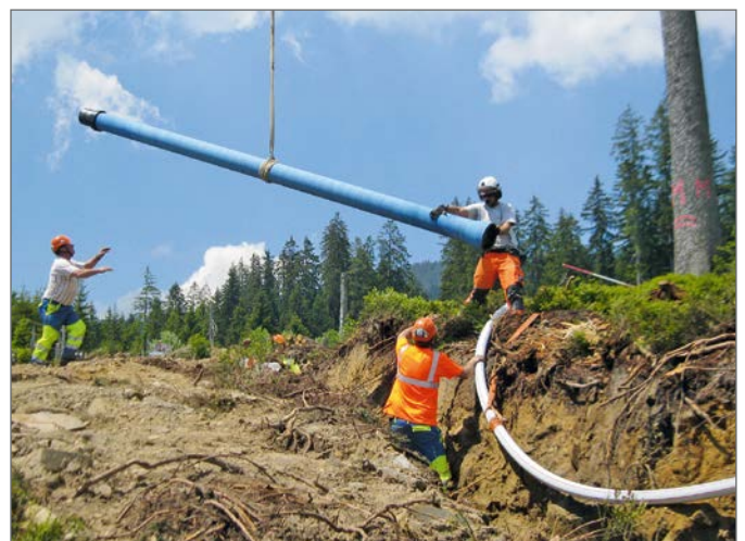
DN 200 iron pipes were flown in where the terrain was steep
