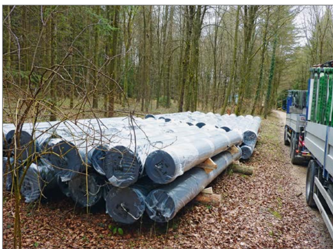
Pipe store in the Gönhard Forest
