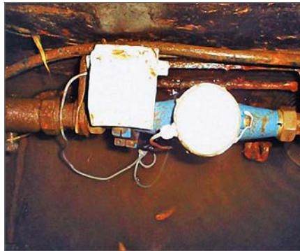
Remotely readable water meter with a two-way 433 MHz short-range radio module
