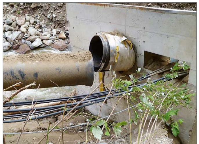
Non-restrained push-in joint which was torn out during the catastrophic bad weather event
