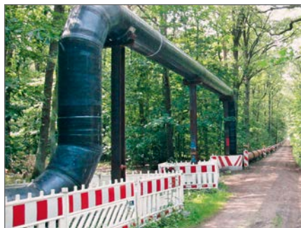
A bridge of steel pipes to maintain access to the forest
