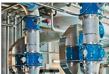
Loose-flanged ROCO wave installed vertically or as an element in a pipeline system
