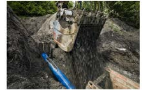
Backfilling the pipe trench with the soil previously excavated
