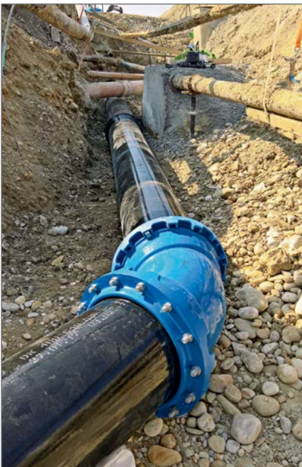
DN 400 double-socket bend before the pipeline runs beneath existing works pipelines
