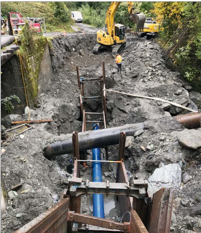
Culverting beneath the stream represented a challenge.
