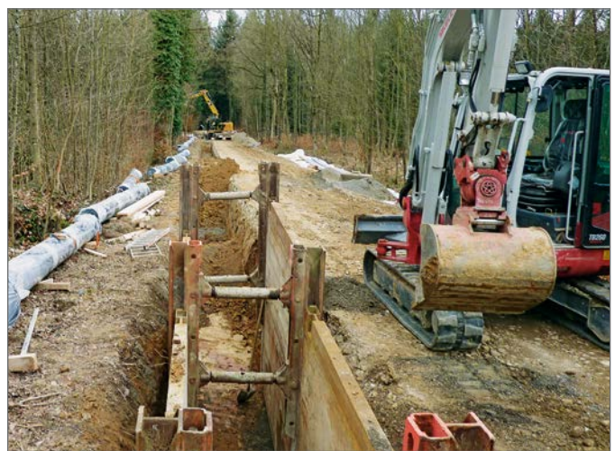
The route of the pipeline alongside a field track
