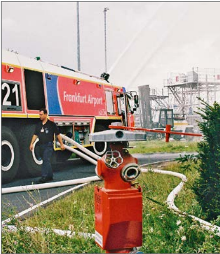
Industrial hydrant for extinguishing water supply at airports
