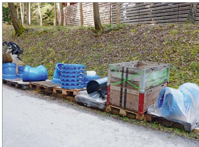
Stock of fittings at the construction site
