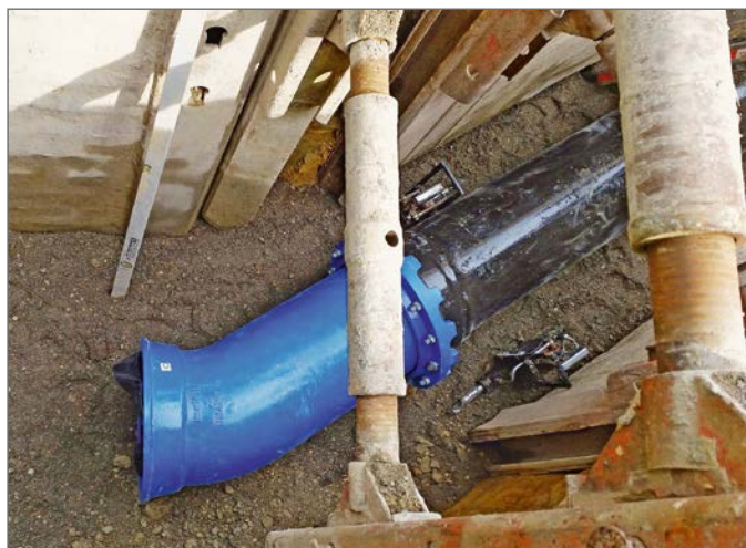
MK 45° bend installed
