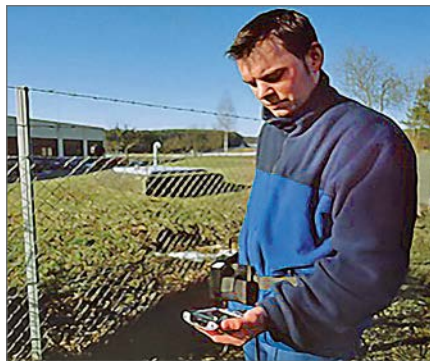
Reading a remote read-out water meter; no more need to climb into the shaft
