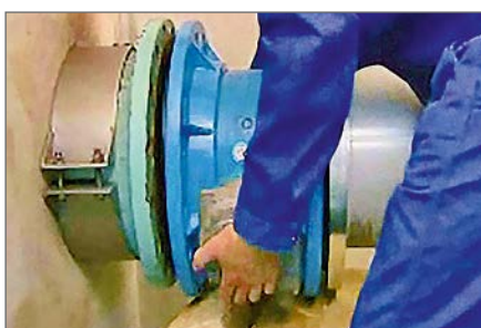
Easier assembly using the single-side loose flange
