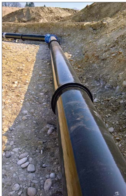
ECOPUR DN 400 restrained pipe with thrust protection (Fig. 2807A)
