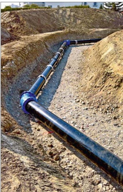
Relocation of a DN 400 transport pipeline because of a new roundabout
