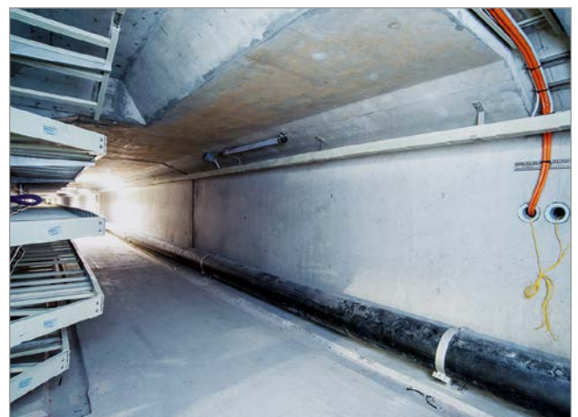
Figure 5: DUCPUR heat-insulated ductile iron pipes in the service conduit
