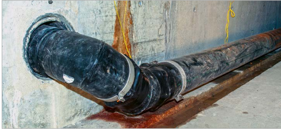
Figure 7: Post-insulation with shrink-on sleeves at the sockets of the push-in joints
