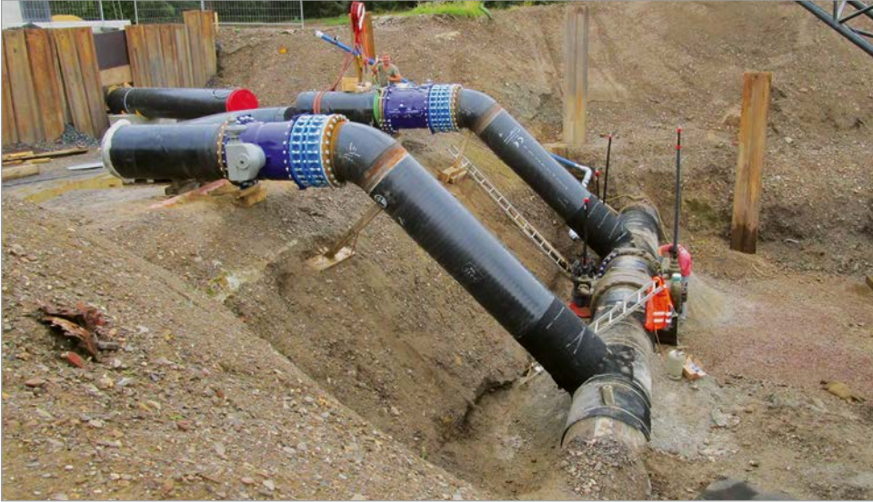
Figure 1: DN 800 feed and discharge line with enamelled DN 800 butterfly valves in ductile cast iron for the UV plant at the WWWW waterworks in Halingen
