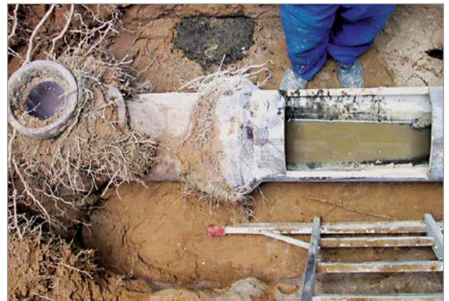
Figure 6: Roots at a depth of 7 m, which have grown down to this depth because of the good oxygen supply Source: Schmiedener, H.
