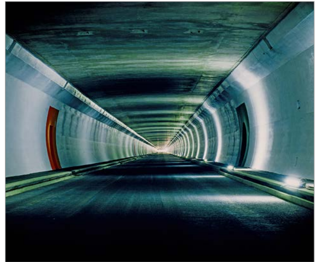
Figure 3: A perspective of the Längholz road tunnel with lateral refuges/hydrant recesses
