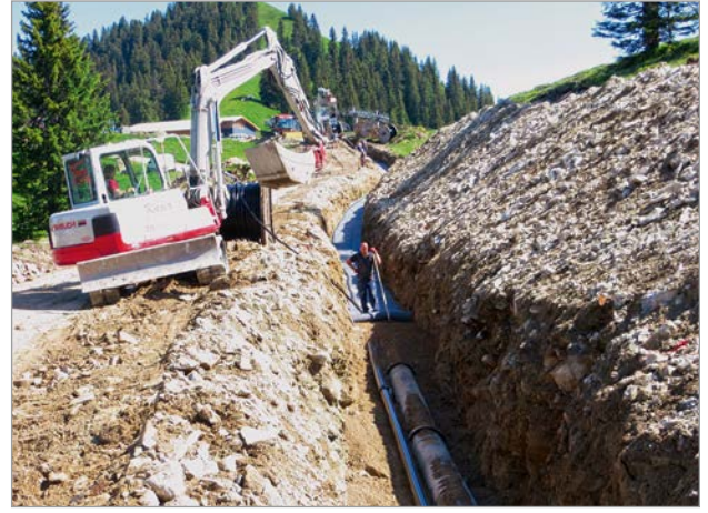
Figure 3: Field pipeline installation – DN 500 transport pipeline
