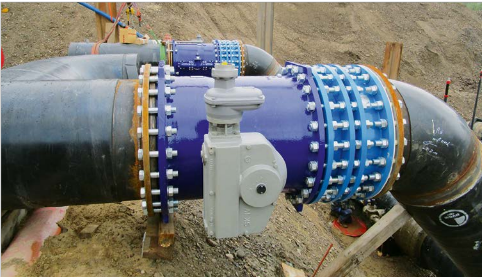
Figure 2: Detailed view of an enamelled DN 800 butterfly valve with lateral bypass and dismantling joint for the UV plant at the WWWW waterworks in Halingen
