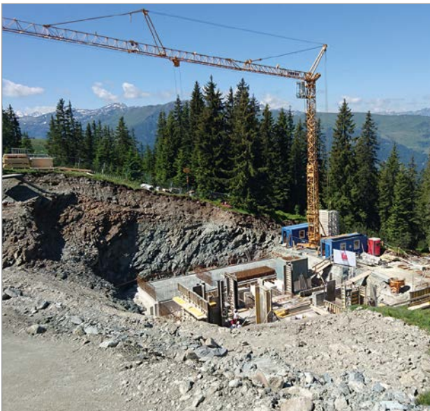
Figure 2: Construction of the new pumping station
