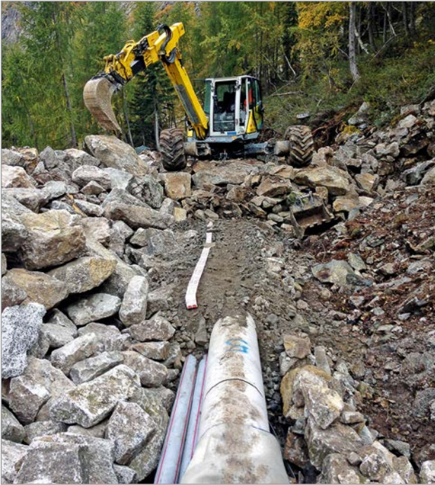
Figure 12: ECOPUR pressure pipeline with parallel-running empty pipes for supply and control cables
