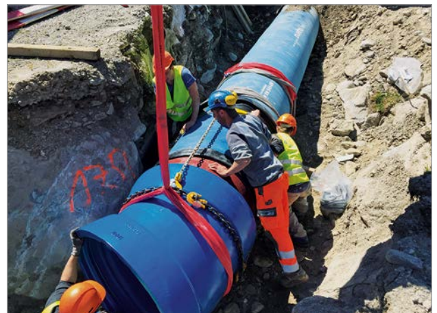
Figure 3: Installation of a 22° double socket bend (MMK 22) and an adapter pipe for a change of direction
