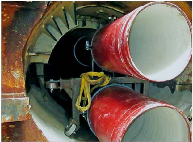
Figure 7: Pulling in the prepared pipe bundle
