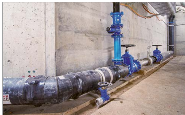
Figure 15: vonRoll valves in use – section valves, shutoff valves for branch pipelines and a tapping saddle for drainage
