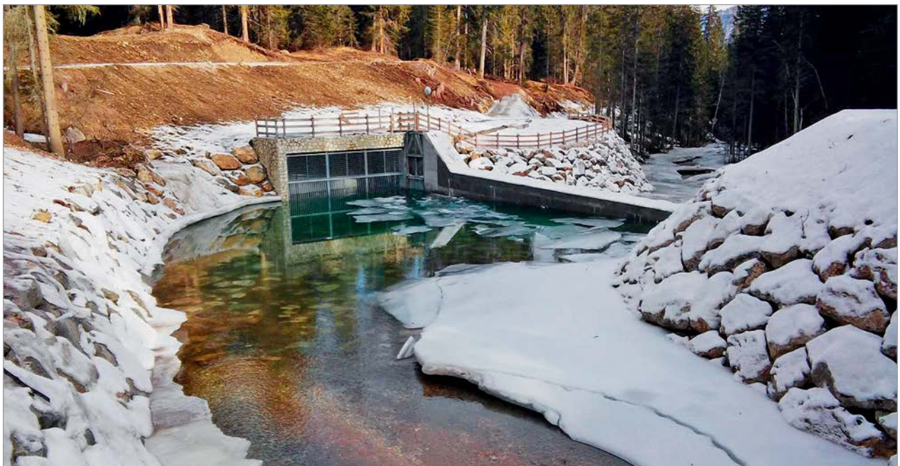
Figure 1: Costeana small hydropower station
