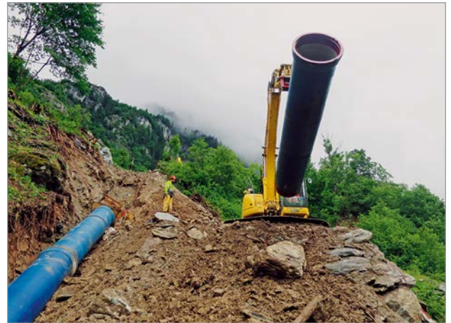
Figure 2: Assembling a ductile iron pipe “upside-down”
