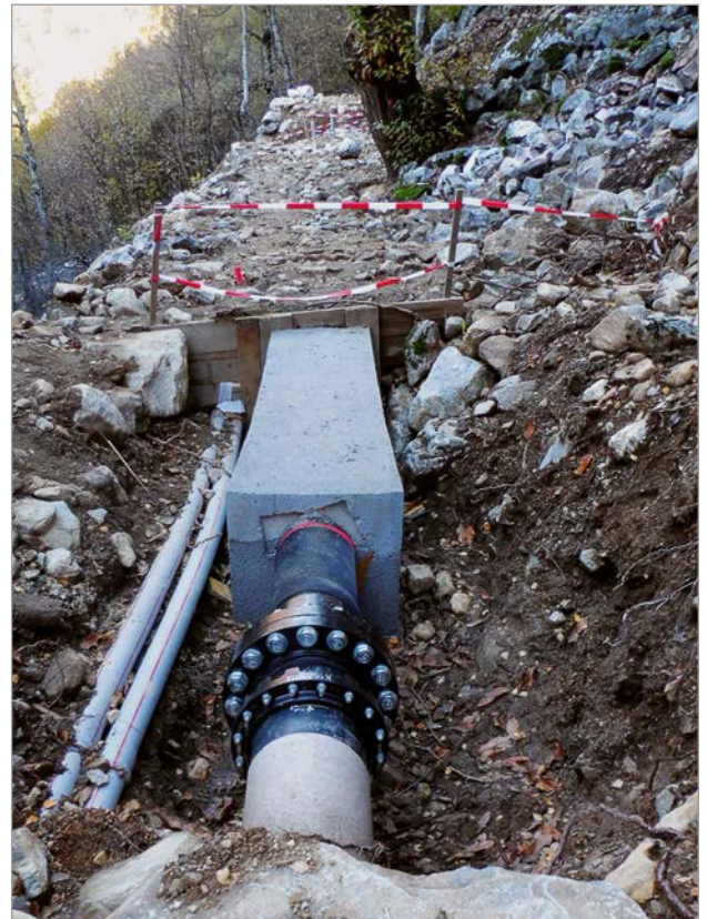
Figure 11: Transition from ductile cast iron to steel, special fitting, flanged socket (E), with PN 100 bar flange
