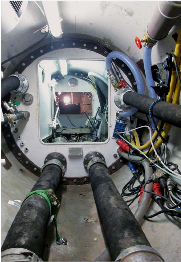
Figure 4: View inside the lock chamber
