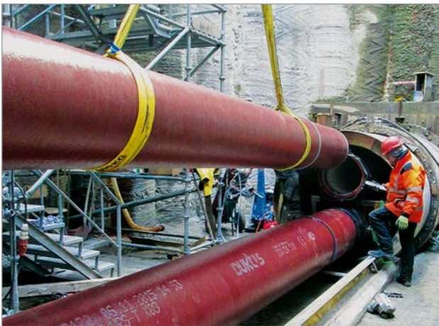
Figure 6: Assembling the ductile iron pipes in the launch shaft
