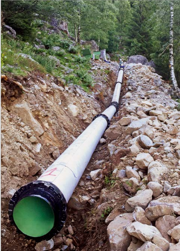
Figure 9: ECOPUR full-protection pipes with ROCK protective cover and external HYRDOTIGHT thrust protection Fig. 2805
