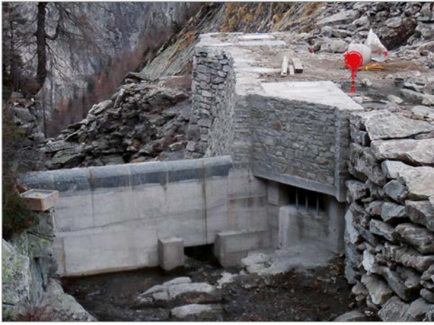
Figure 2: Water supply into the inlet structure
