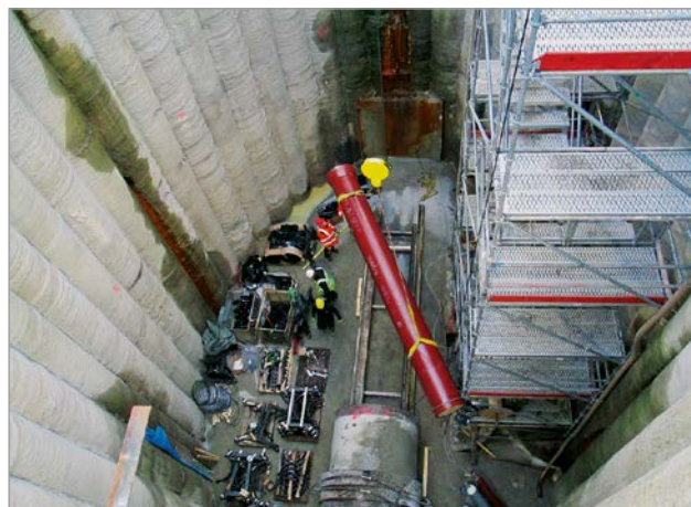
Figure 2: Lowering a ductile iron pipe ready for assembly
