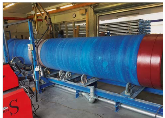
Figure 4: An adapter pipe being put together at the Hagenbucher centre of competence in Eglisau
