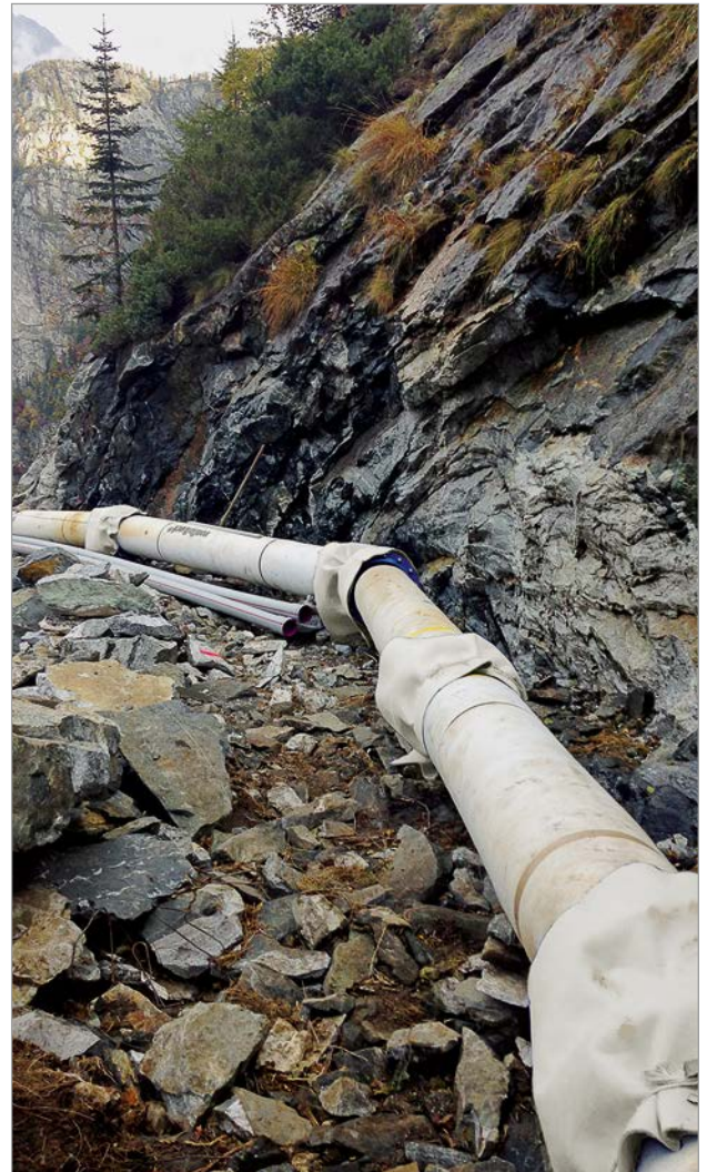
Figure 5: Deflectible HYDROTIGHT push-in joint
