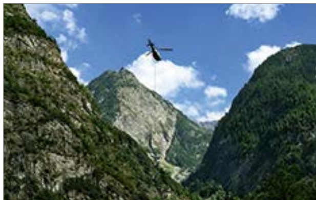
Figure 6: Transport and installation of ECOPUR pipes by helicopter
