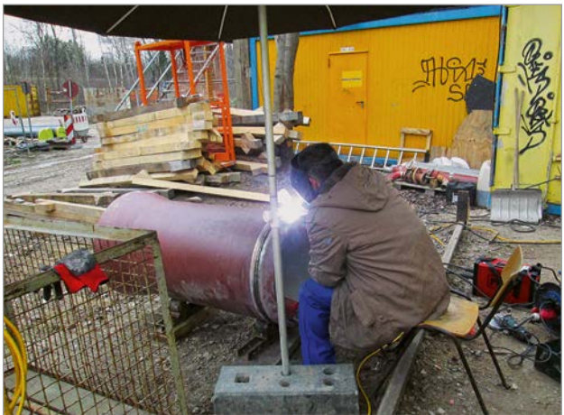
Figure 8: An application engineer from the pipe manufacturer applying a welding bead
