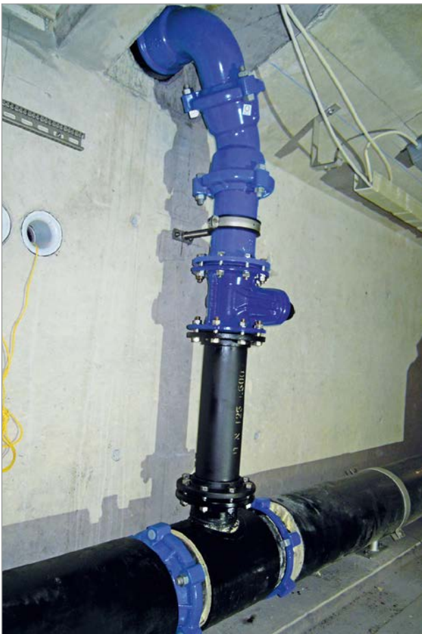
Figure 11: DN 125 branch pipeline, easily aligned fittings with external thrust protection Fig. 2806
