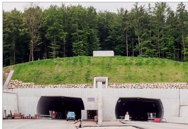
Figure 1: A view of the portal area of the Längholz tunnel
