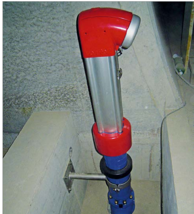
Figure 14: vonRoll VARIO 2.0 hydrant lower section and vonRoll HYTEC hydrant upper section after final assembly
