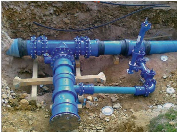
Figure 10: DN 400 valve intersection with DN 100 bypass
