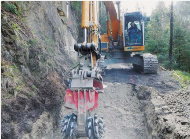
Figure 9: Using the cutter-head excavator
