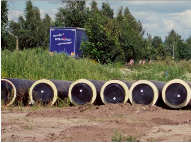
Figure 5: Pipes for installation underground with PE outer casing
