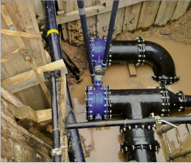
Figure 3: Ready-assembled DN 400 vonRoll shut-off butterfly valves
