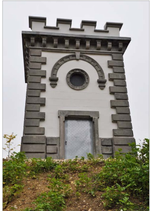
Figure 4: Restored tower of the valve chamber
