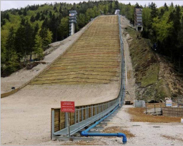
Figure 8: Snow-making equipment on the ski jumping hill in Planica, Slovenia [11]
