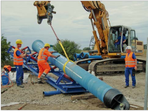
Figure 2: Assembly ramp for single pipe assembly
