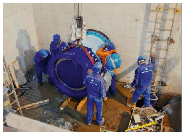
Figure 2: Installing the double eccentric, fully enamelled DN 1200, PN 10 butterfly valve
