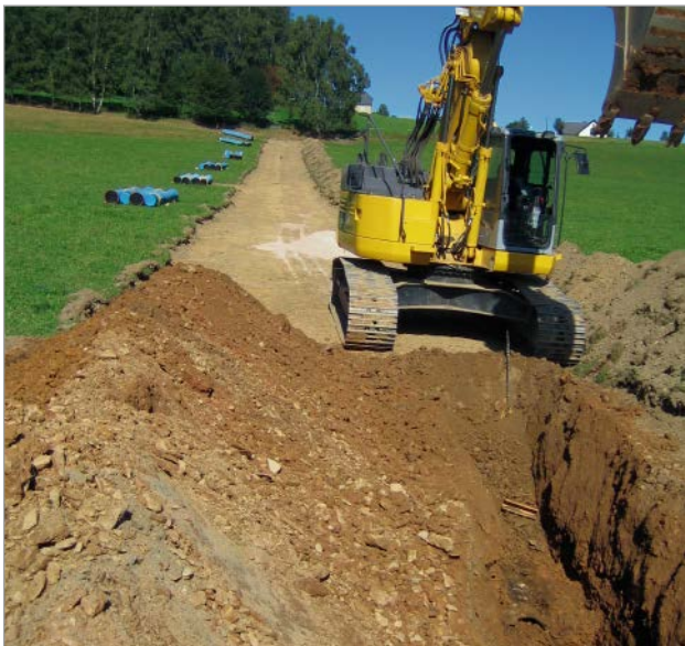
Figure 6: The route of the cement mortar coated DN 400 BLS® pipes
