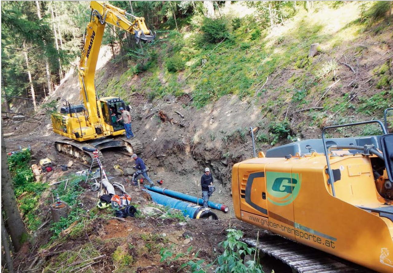
Figure 10: Parallel installation of DN 200 and DN 600 ductile iron pipes
