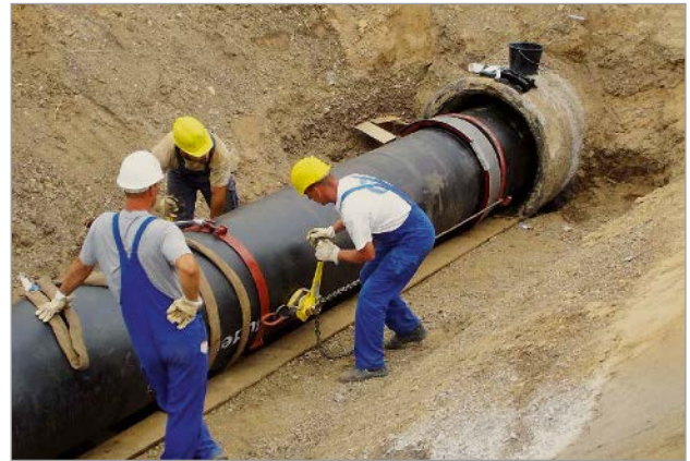
Figure 10: Pipe relining with DN 800 pipes
