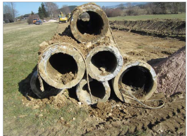
Figure 4: DN 450 concrete pipes removed from the old pipeline
