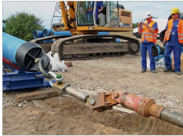
Figure 3: Traction head with tensile force gauge
