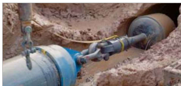
Figure 9: DN 900 installation with the HDD technique in Valencia, 2007
