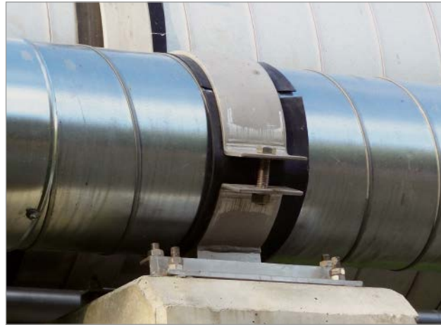
Figure 9: Rubber interfaces between folded spiral-seam outer tube and bearing
