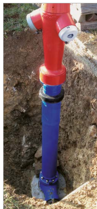
Figure 5: The polymer concrete base offers an ideal foundation for the entire hydrant combination – pillar hydrant design
