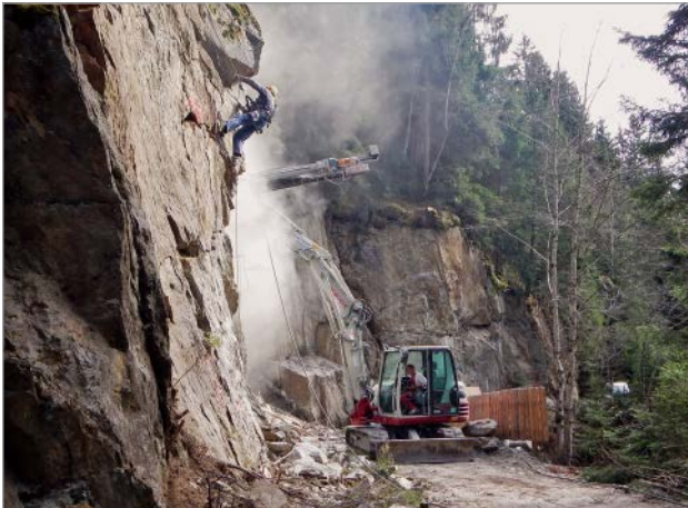
Figure 8: Construction work in the rock
