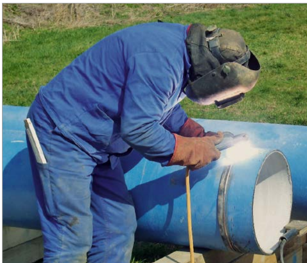
Figure 11: Applying the welding bead for the BLS® system
