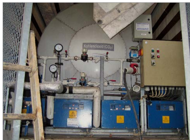
Figure 13: Vaporiser system as the source of CO 2
