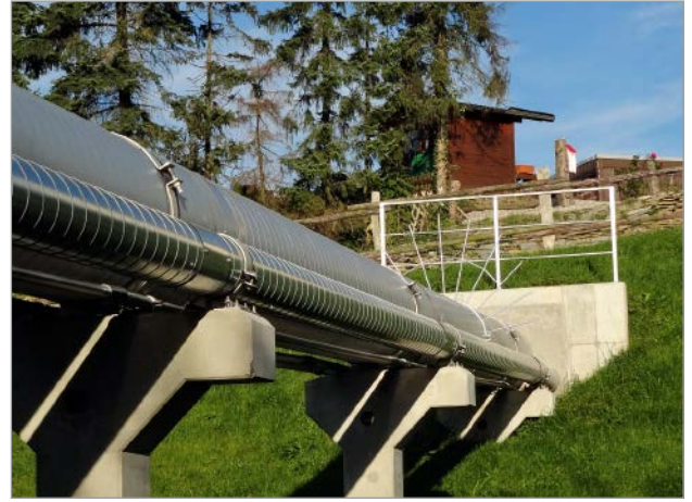
Figure 6: Support distance = pipe length = 6 m
