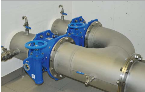
Figure 2: ROCO wave butterfly valves, DN 150, PN 16
