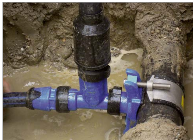
Figure 4: Tapping under mains pressure
