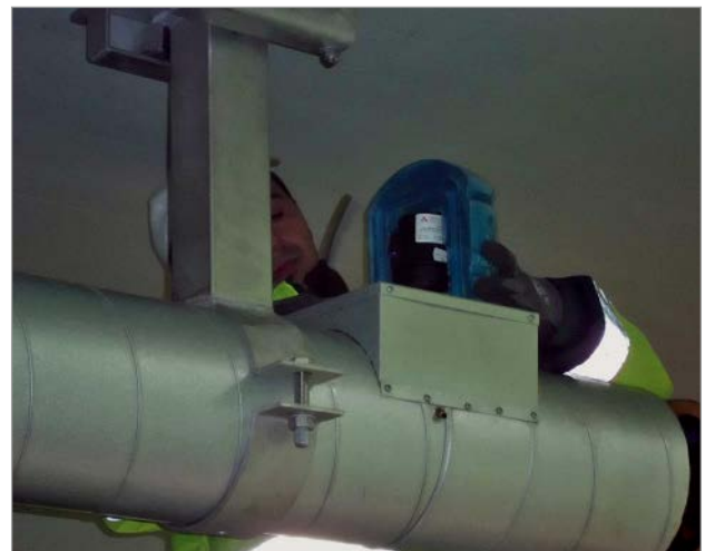
Figure 10: 1.5" threaded female outlet insulated in the factory with shut off capability and ventilation valve with thermal insulation
