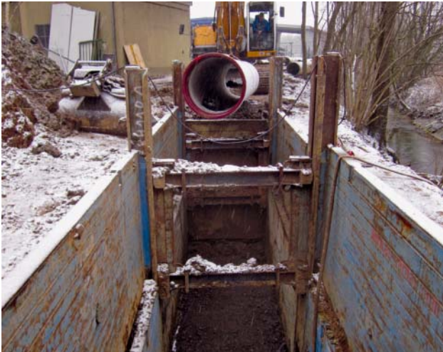
Fig. 5: Securing the trench with shoring equipment
