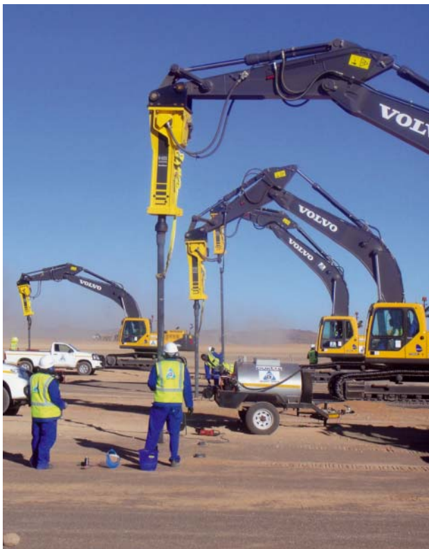
Fig. 2: Four machines for sinking the ductile iron driven piles
