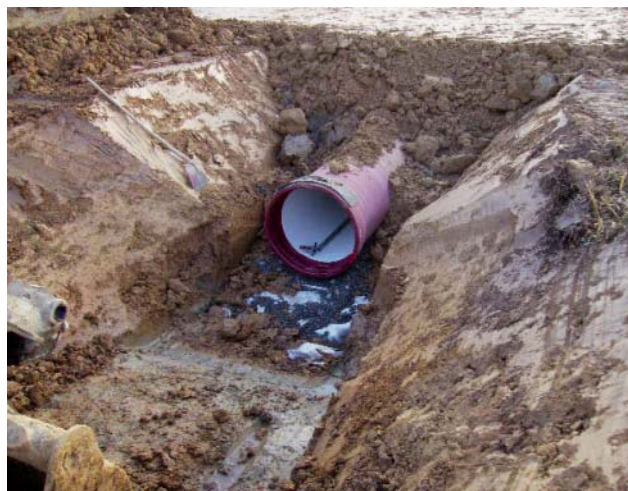
Fig. 10: Pipe trench backfilled with excavation material
