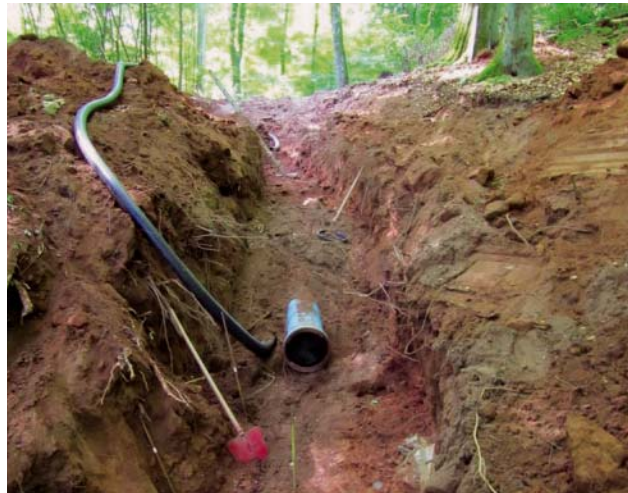
Fig. 7: DN 300 ductile iron pipes – installation in the trench
