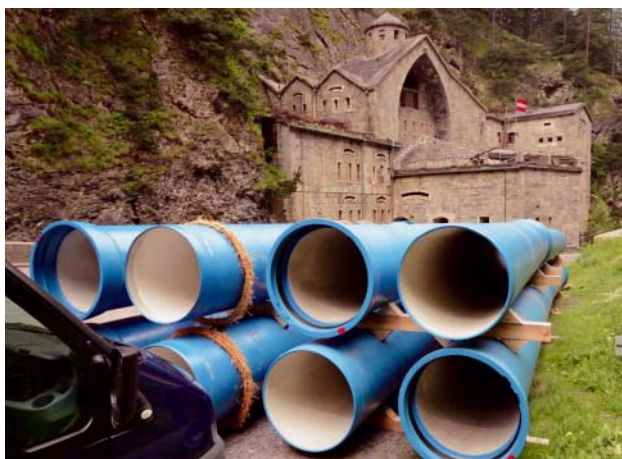
Fig. 1: Ductile iron pipes – pipe store for the construction of the pressure pipeline for the Stiller Bach hydroelectric power station in Nauders.
