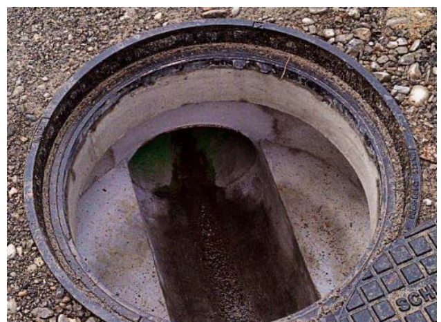
Fig. 5: In-situ concrete manhole with flow channel and shoulder
