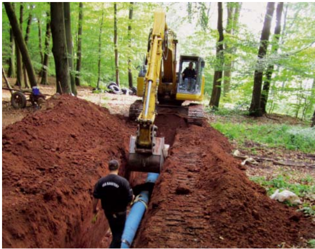
Fig. 2: Installation of the pipes in a narrow track through the wood
