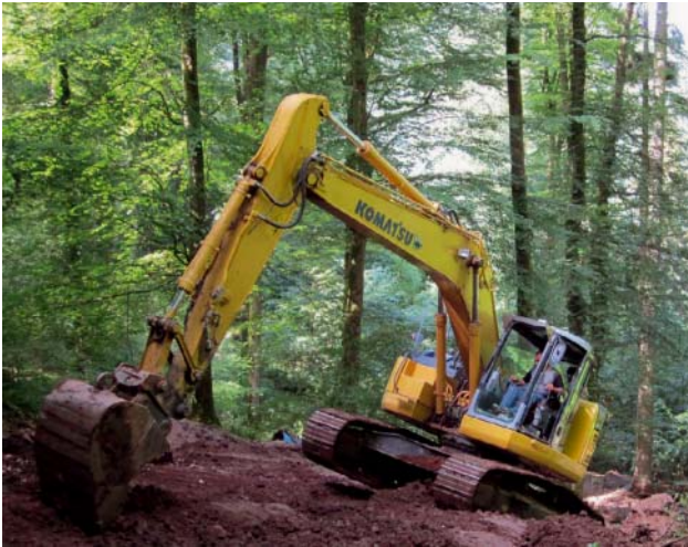
Fig. 4: Civil engineering work in the rocky terrain of the wooded slope
