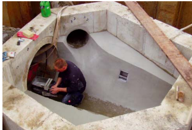
Fig. 3: Reinforced concrete structure
