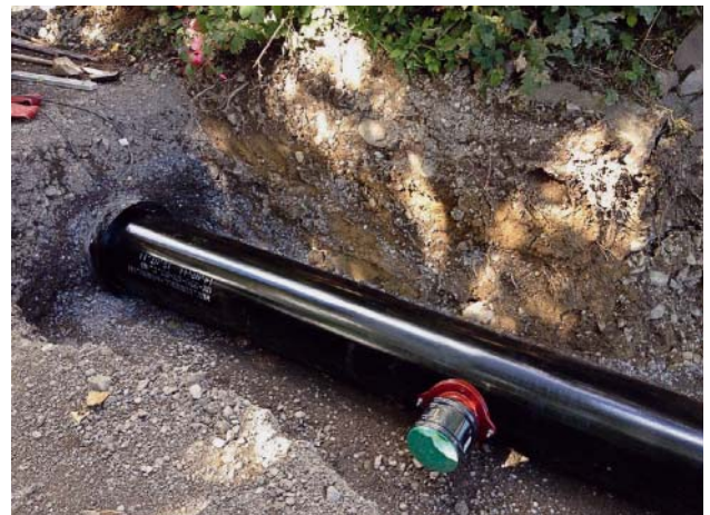
Fig. 4: Tapping saddle assembled after treatment of the cutting edge with epoxy resin and transition sleeve assembled on a plastic pipe
