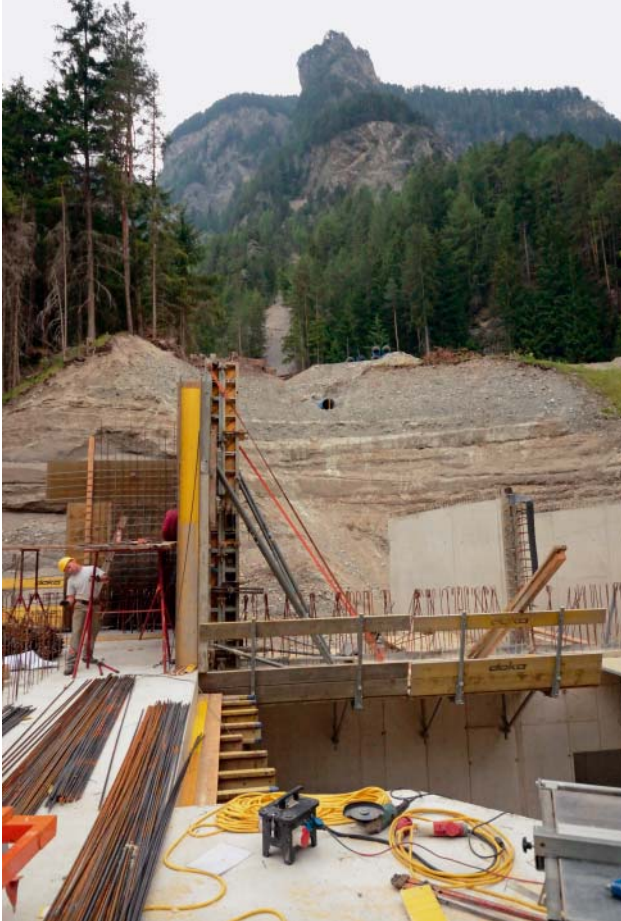
Fig. 10: Construction of the machine hall of a considerable dimension
