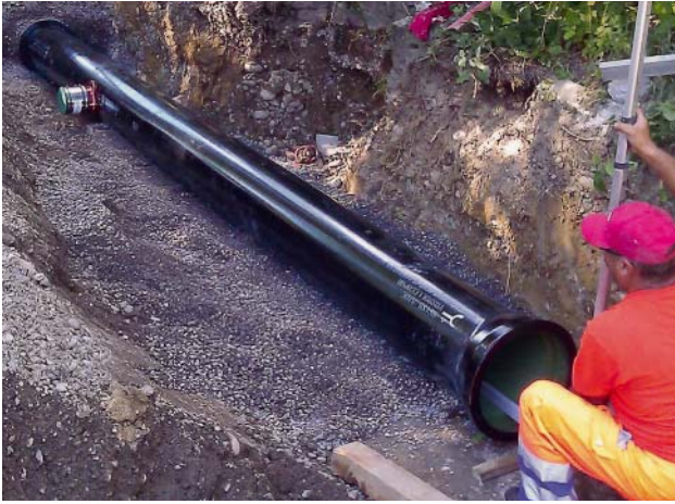
Fig. 6: Checking the gradient of the installed vonRoll ECOPUR pipes
