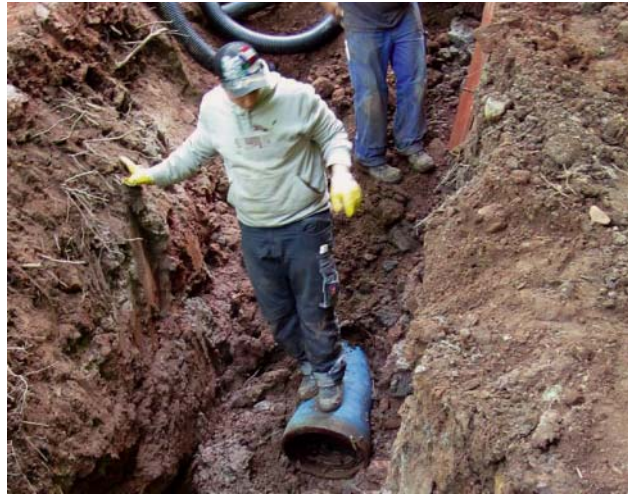
Fig. 6: Assembling the push-in joint with the socket against the direction of flow
