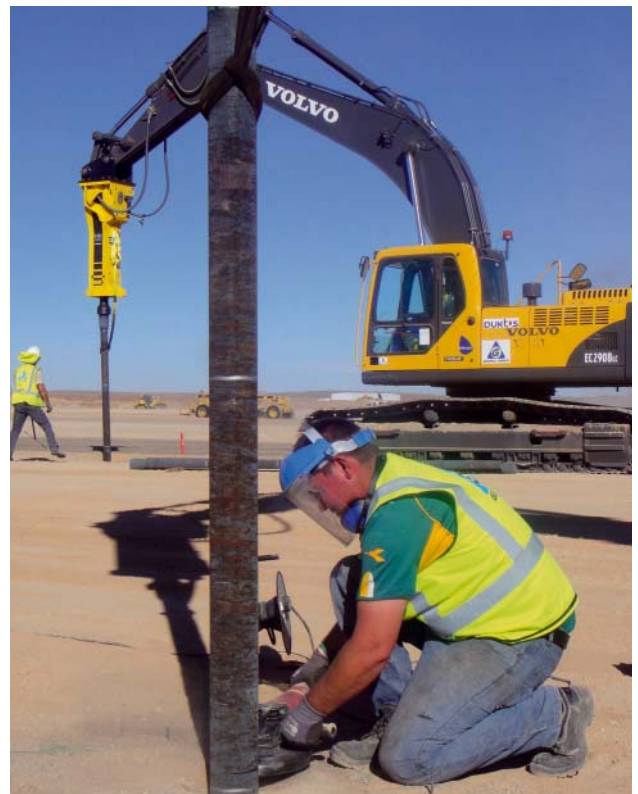
Fig. 3: Cutting off the surplus length of a driven iron pile
