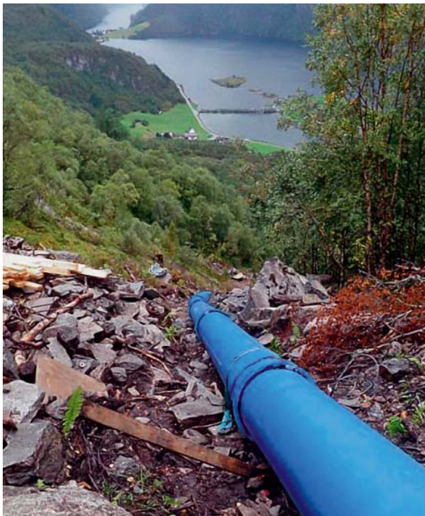
Fig. 10: Completed steep-gradient pipeline with restrained BLS® push-in joints
