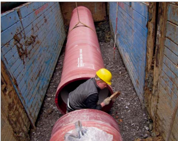
Fig. 6: Pipe laying in a shored pipe trench
