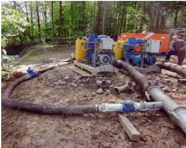
Fig. 12: Waste water retention during the switchover to the new sewer
