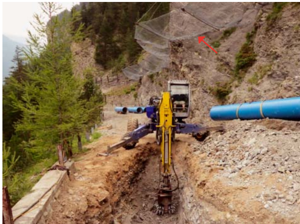
Fig. 5: Rock fall protection measures along the pipeline route
