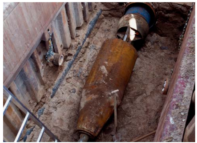
Fig. 8: Upsizing head, traction gauge and traction head
