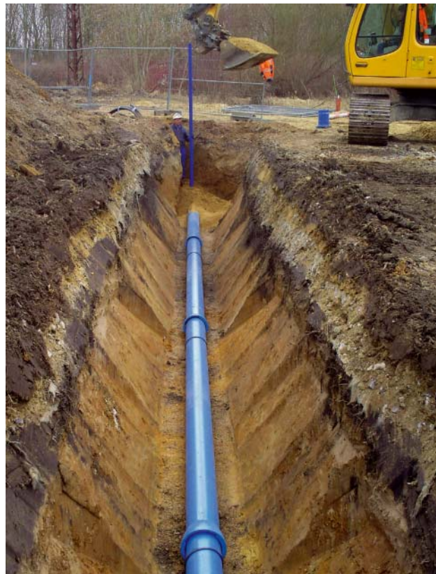
Fig. 4: Installation of DN 250 ductile iron pipes in the sloped trench
