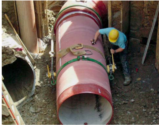
Fig. 8: Lower bedding layer with 0/45 mm mineral aggregate
