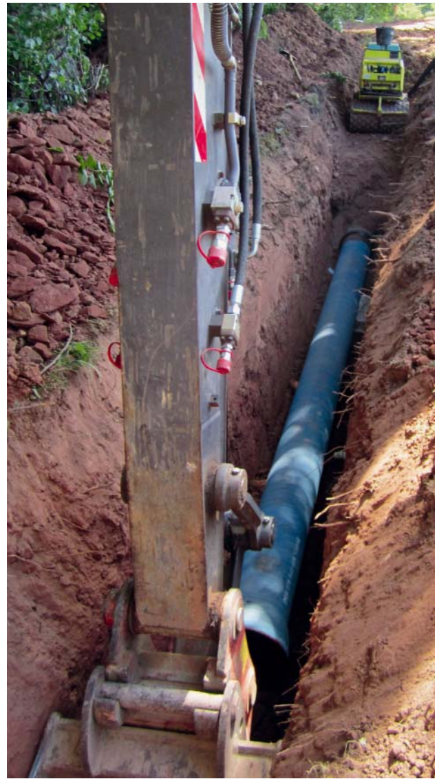
Fig. 3: Installation of the DN 300 ductile iron pipes in the flat area
