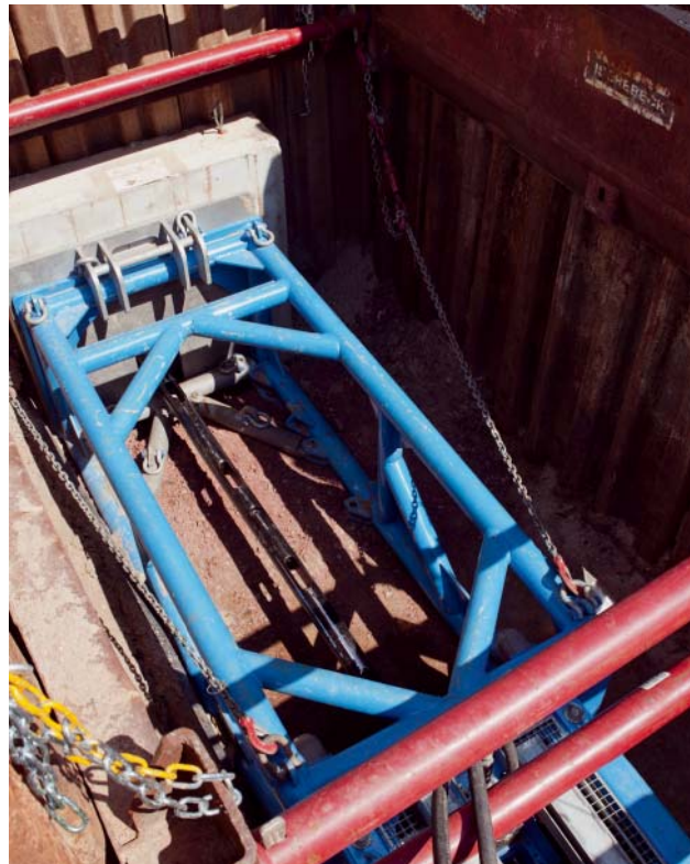
Fig. 6: Reusable reinforced concrete thrust block Source: BASF SE, Ludwigshafen
