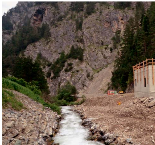
Fig. 4: Double-chamber sand trap at the catchment structure
