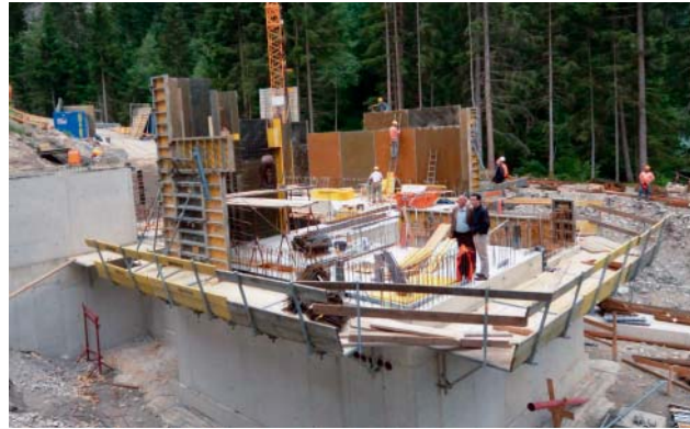
Fig. 11: New machine hall at the mouth of the Inn
