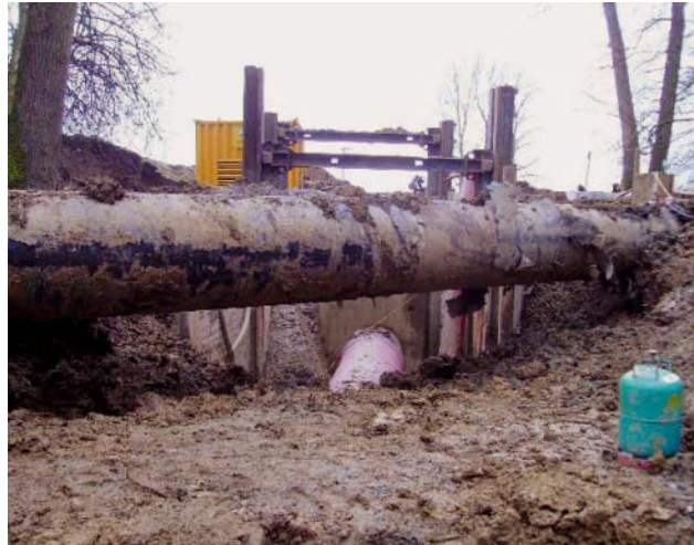
Fig. 9: Krebsbach intersection with raised base profile
