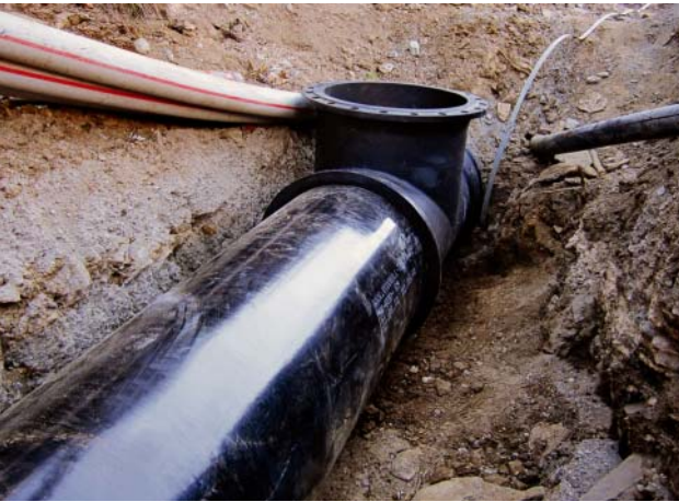
Fig. 2: Manhole for maintenance and overhaul work in construction, designed with DN 600/600 double-socket tee with flanged 90° branch, coated with epoxy resin. In the final version, equipped with DN 600 black flange incl. baffle plate
