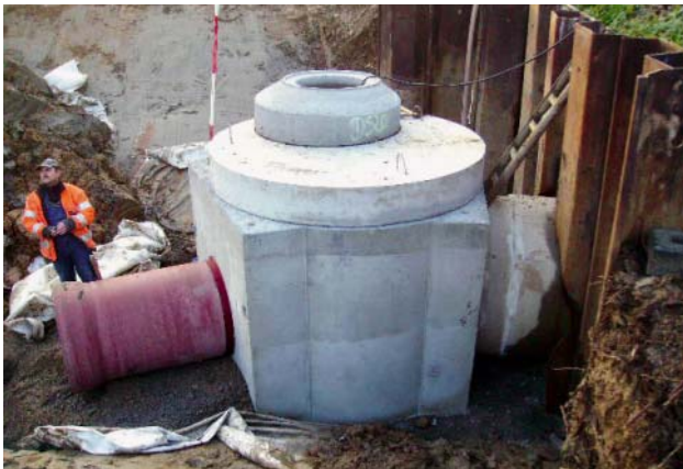
Fig. 2: Prefabricated manhole
