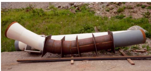
Fig. 9: Eccentric steel cone – transition from the pressure chamber of the sand trap to the pressure pipeline
