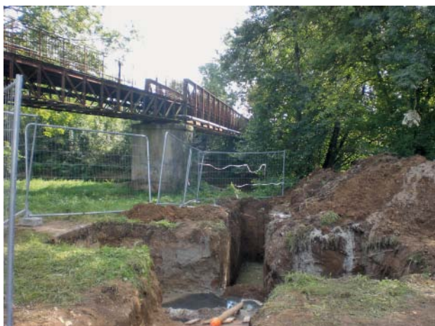
Fig. 1: The footbridge over the river Marne
