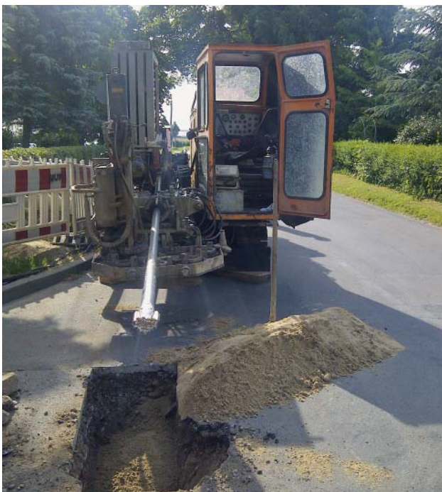
Fig. 2: Preparing for the pilot bore
