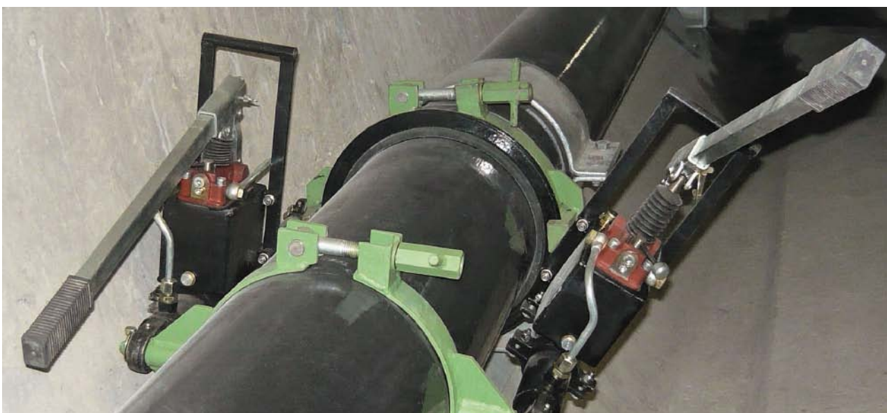
Fig. 8: Assembling a pipe in the utility gallery
