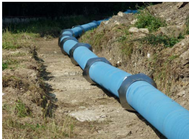
Fig. 4: A pre-assembled pipe string with sheet-metal cones slid over the joints
