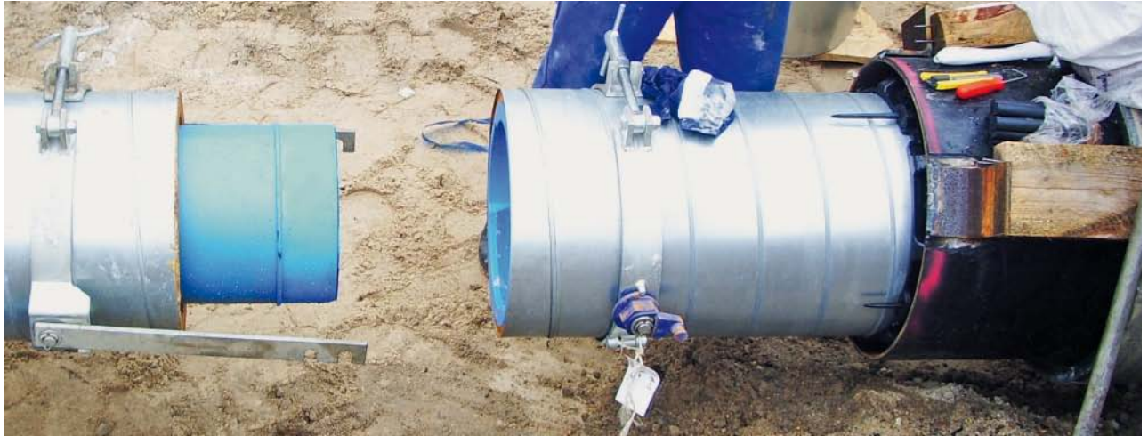
Fig. 6: Preparing to assemble WKG pipes with BLS® push-in joints
