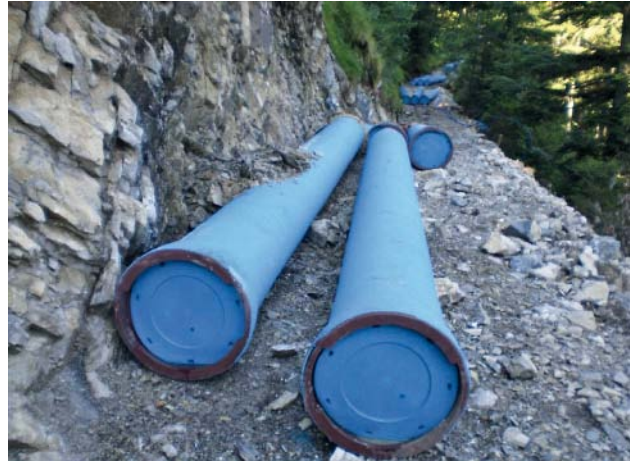
Fig. 4: Installation of ductile iron penstock pipes in rocky terrain
