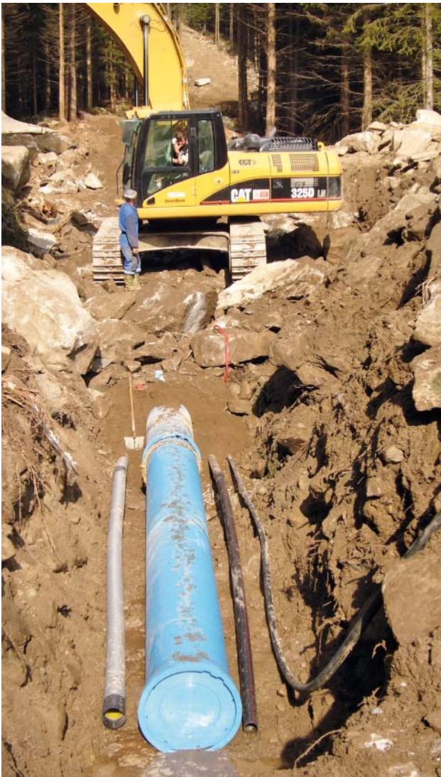
Fig. 3: Installing the DN 600 ductile iron pipes together with empty tubes
