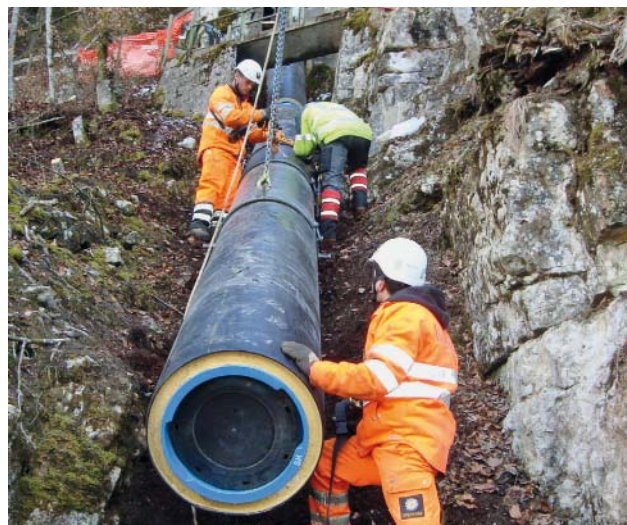
Fig. 3: Ductile iron pipes with additional insulation of rigid polyurethane foam and a casing tube of HDPE
