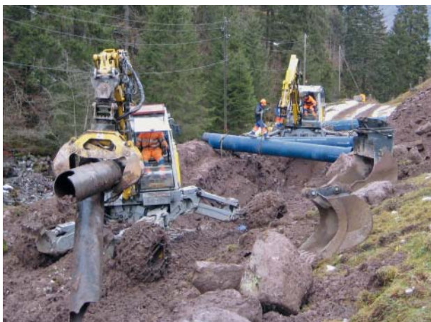
Fig. 9: The “Niedererbach” penstock pipeline: demolishing the old pressure pipeline
