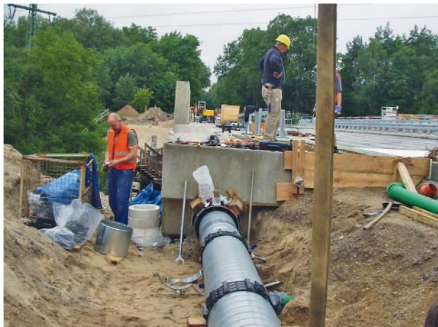
Fig. 18: DN 300 WKG pipes being pulled in on the Nesselgrund bridge
