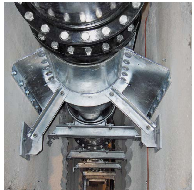
Fig. 17: Pipeline run through between closely spaced compartment walls
