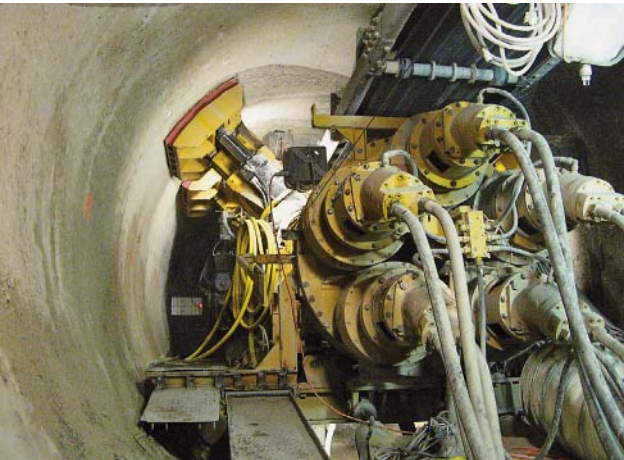
Fig. 5: The tunnel boring machine – in operation
