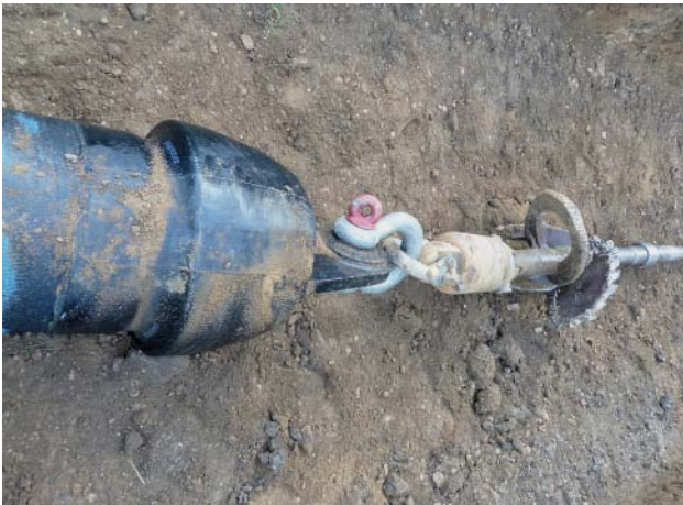
Fig. 5: Traction head plus swivel assembled to pipes
