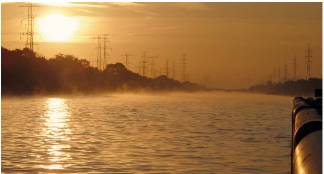
Fig. 1: The Albert Canal near Geel in Belgium, awaiting the installation of a DN 500 ductile iron culvert pipeline
