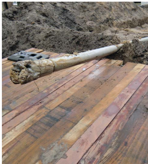
Fig. 3: Arrival at the end of the pilot bore
