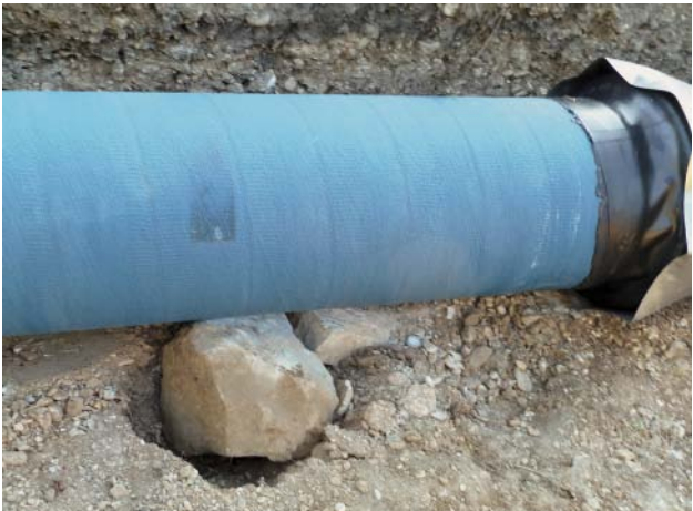
Fig. 8: A stone causing the stress
