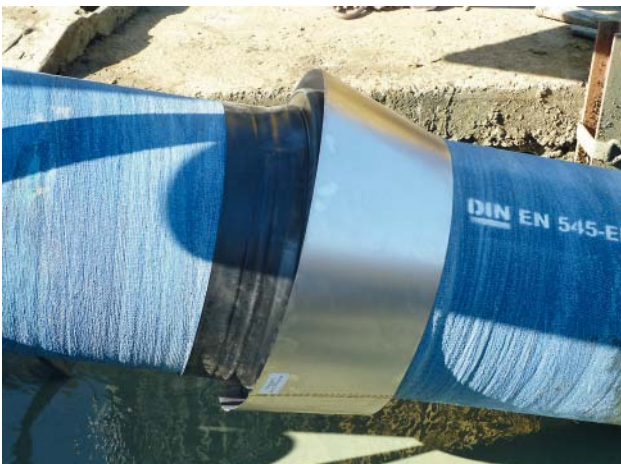
Fig. 7: Socket protection by a rubber protective sleeve
