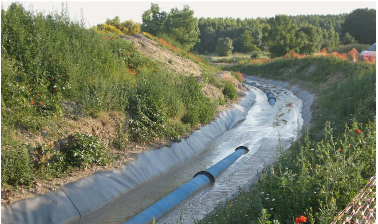
Fig. 8: A pre-assembled pipe string floating in bentonite suspension
