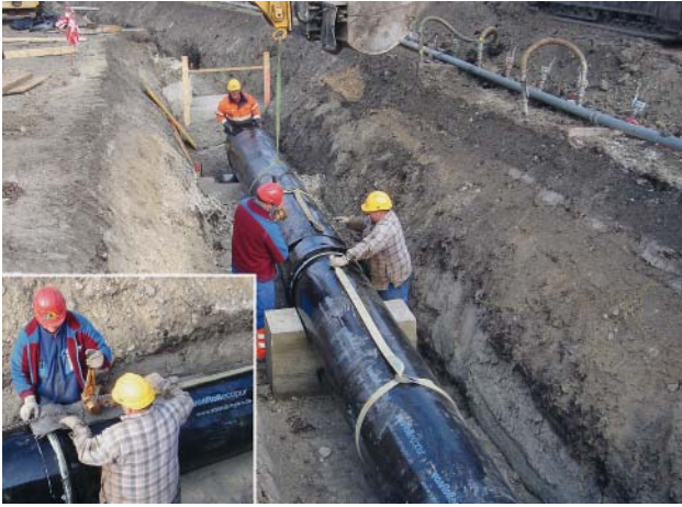
Fig. 3: Pipes being assembled on the heads of piles
