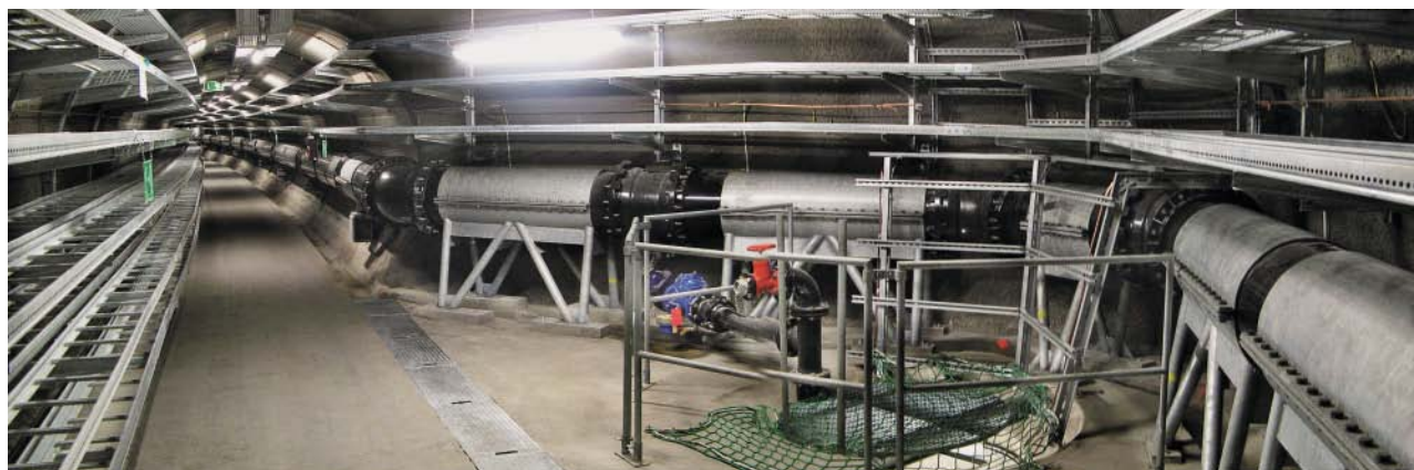
Fig. 13: Widened area containing steel stands – completed state
