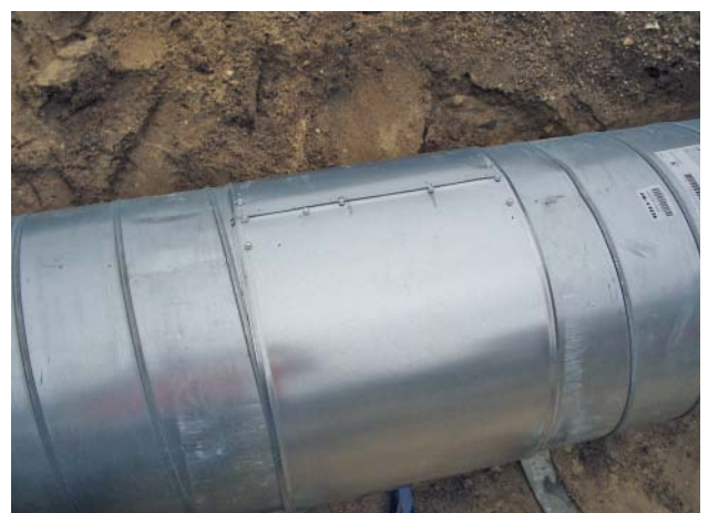
Fig. 9: Fully assembled sheet metal sleeve in the region of the socket joint
