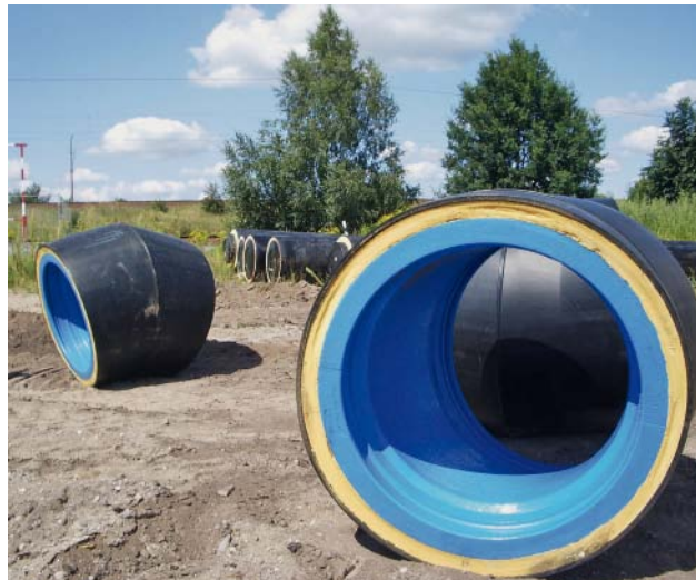
Fig. 4: DN 500 WKG bends for burying
