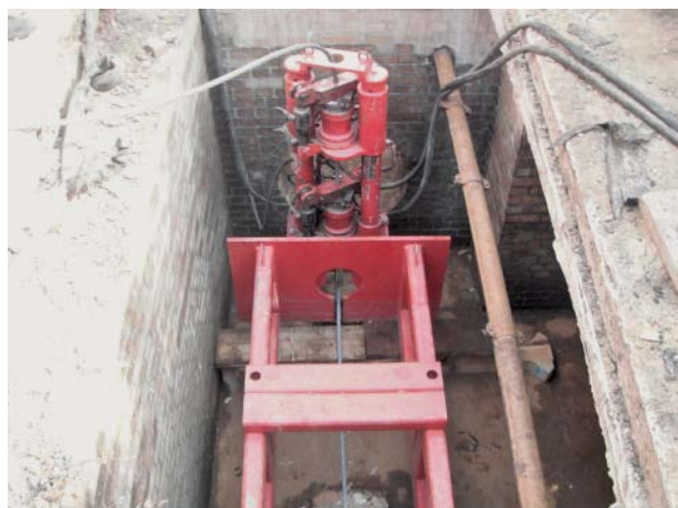
Fig. 5: The hydraulic traction rig [Source: NRM]
