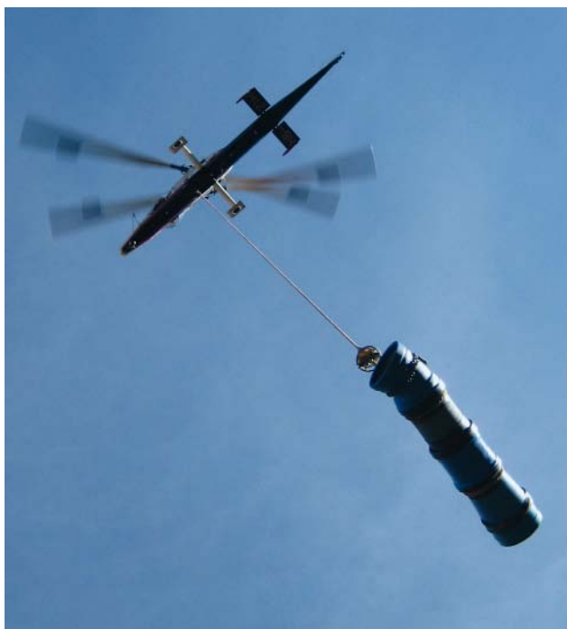
Fig. 4: The “Sagenbach” penstock pipeline: pipe transport by a K-Max helicopter
