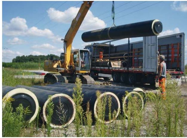
Fig. 10: The Sedlitz project – unloading the DN 500 WKG pipes on site
