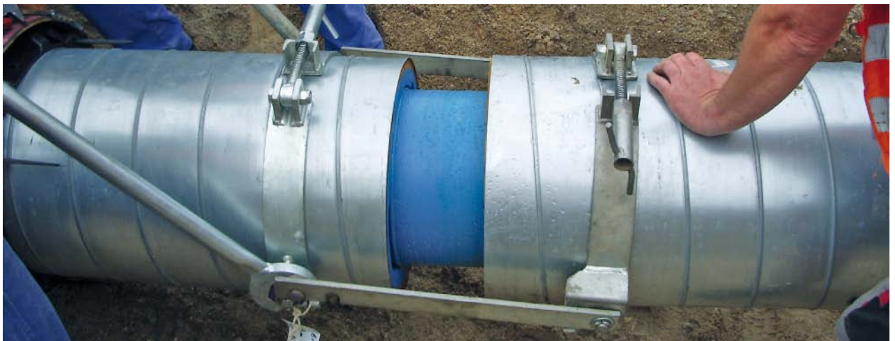
Fig. 7: Pulling the BLS® push-in joint together with an assembly tool
