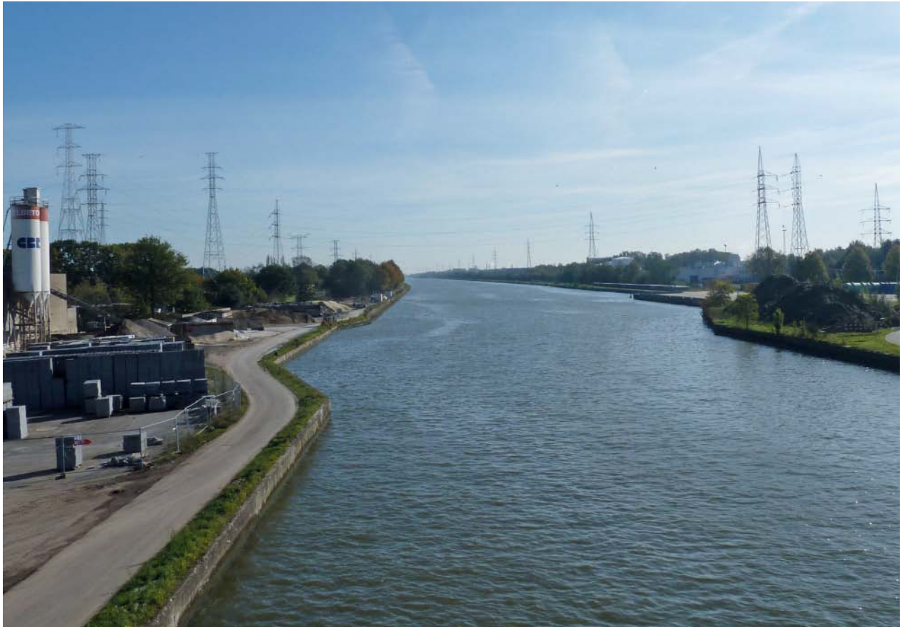
Fig. 10: The Albert Canal near Geel in Belgium after a culvert pipeline of DN 500 ductile iron pipes was installed
