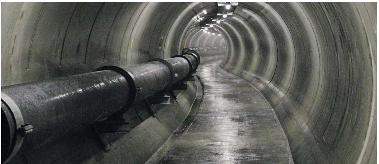
Fig. 10: An assembled run at radiuses up to R = 200 m
