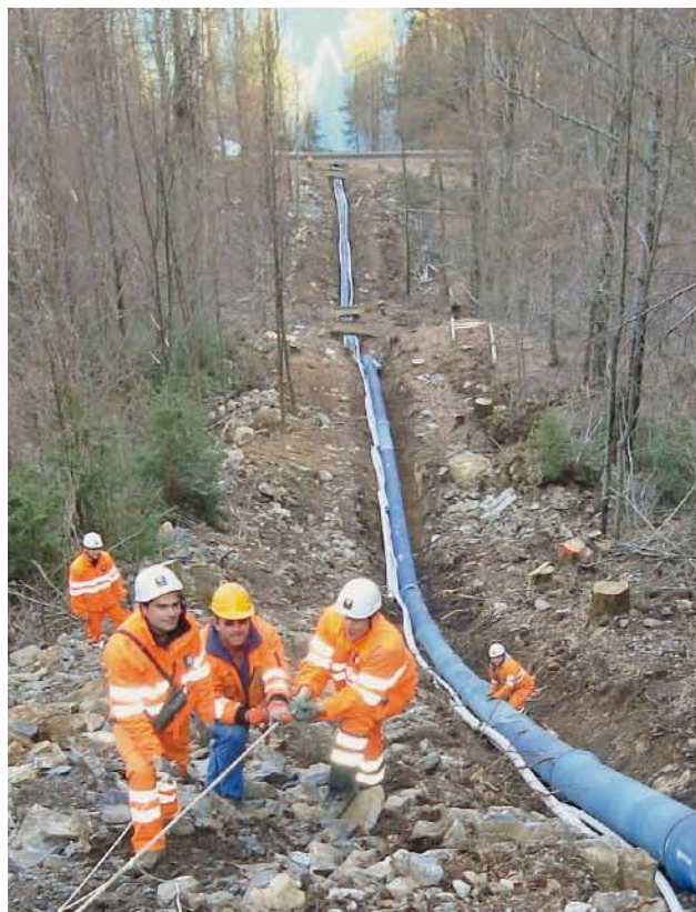
Fig. 7: Path followed by the DN 400 pressure pipeline
