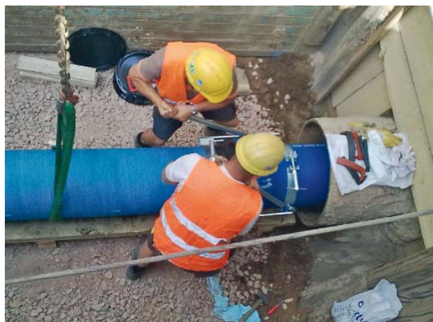
Fig. 4: Assembling a BLS®/VRS®-T push-in joint [Source: NRM]
