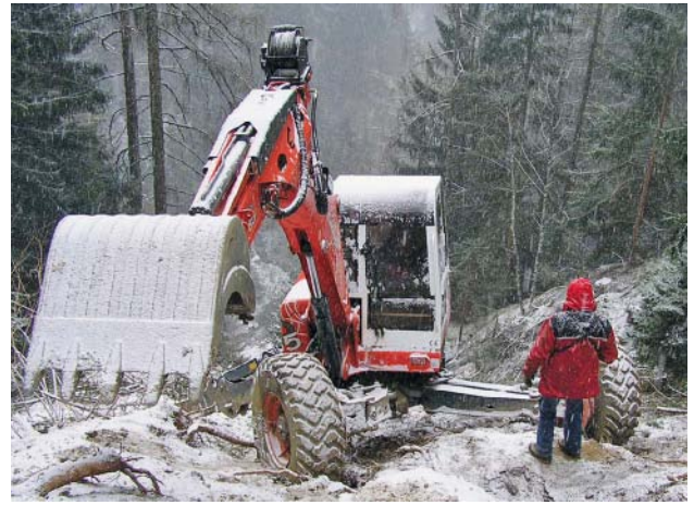
Fig. 6: Bad weather conditions making installation very difficult
