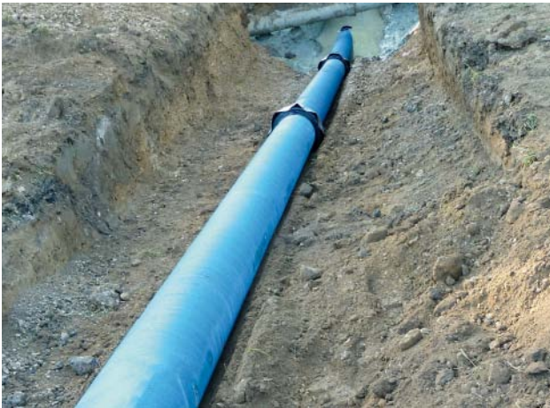
Fig. 6: Pulling in the pipe string
