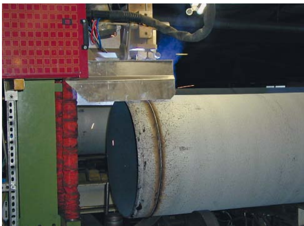
Fig. 4: The welded bead applied in the factory
