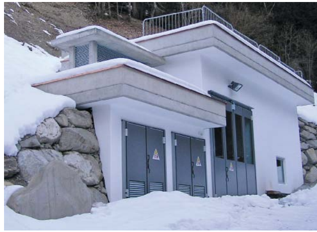
Fig. 10: The turbine house built into the steep slope
