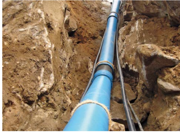
Fig. 2: Very cramped conditions for Installing the ductile iron pipes
