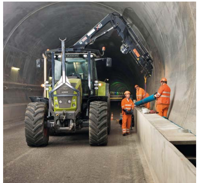
Fig. 10: Towing tractor and crane boom
