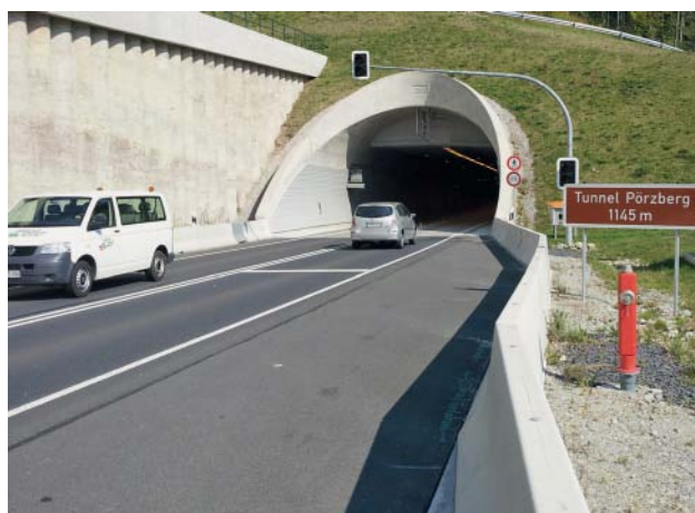
Fig. 5: The Porzberg tunnel near Schaala
