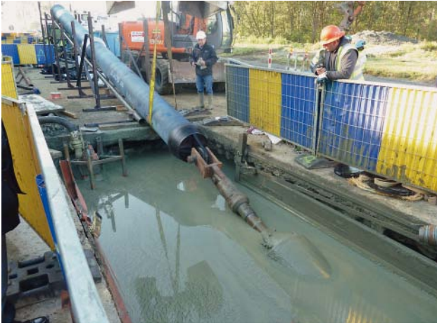
Fig. 9: Assembly on a ramp
