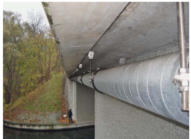
Fig. 22: The Hohenauen bridge: a suspended WKG pipeline with no bridge skirt
