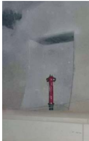
Fig. 2: DN 80 pillar hydrant with two outlets
