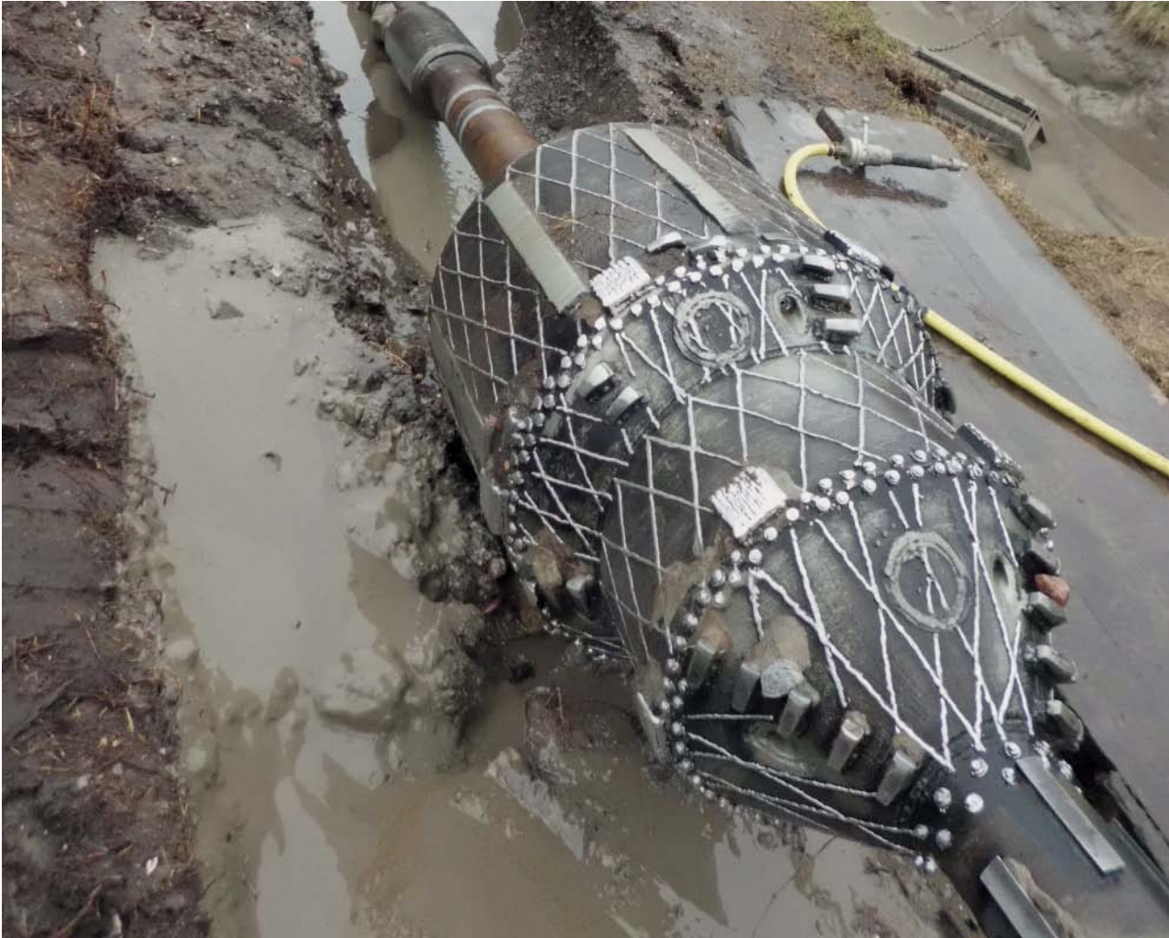
Fig. 5: Arrival of the upsizing head in the target pit
