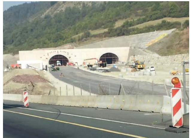
Fig. 1: Eastern portal of the Jagdberg tunnel
