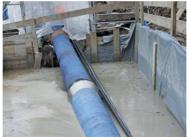
Fig. 11: The DN 700 ductile iron pipeline dipping into the drilling fluid
