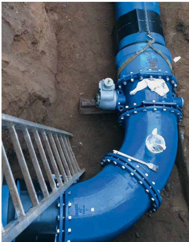
Fig. 8: Ductile iron fittings and a butterfly valve which were installed
