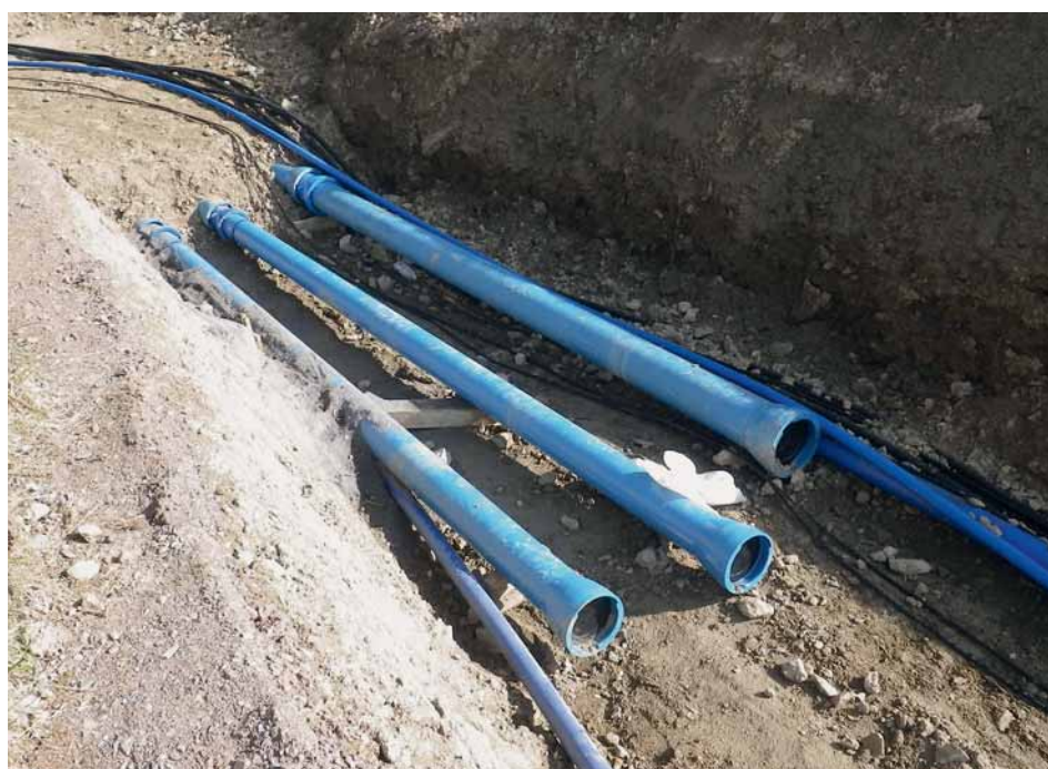
Fig. 6: Ductile iron pipes with restrained push-in joints
