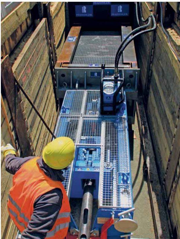
Fig. 4: Groundoburst 2500 G with a front frame
