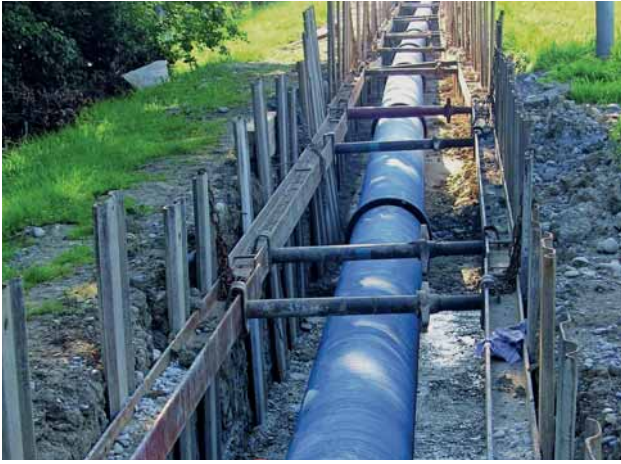
Fig. 1 Ductile iron pipes do not require a sand bedding
