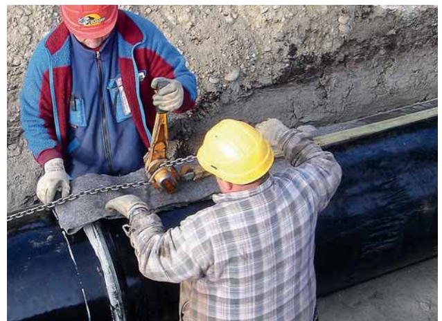
Fig. 8: DN 700 ductile iron pipes – easy, time-saving assembly
