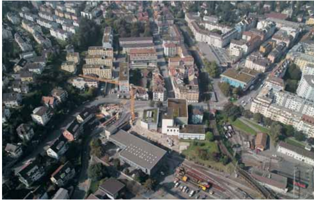
Fig. 4: Aerial photo of the area of the “Lowering of level of the Lucerne Zentralbahn” site, where ductile iron piles were used for the first phase of the work
