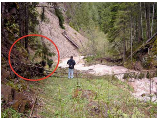
Fig. 1: The turbine pipeline was installed straight through the mountain at the point indicated by the red circle
