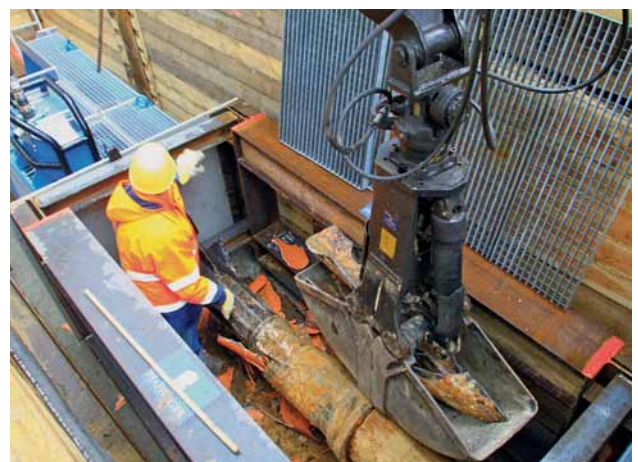
Fig. 11: Bursting mandrel and removal of the fragments of old pipe
