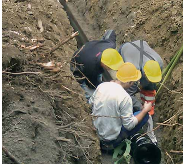
Fig. 2: Installing a vonRollecopur DN 200, PFA 40, wall-thickness class K 9 pipe
