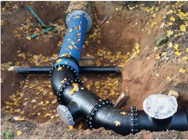
Fig. 3: Installation above an existing pipeline
