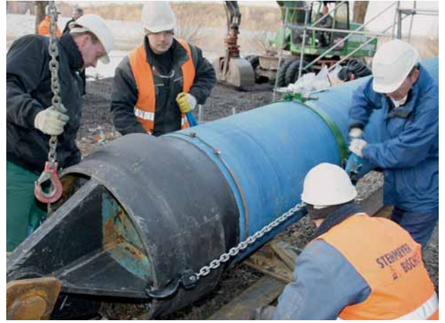
Fig. 10: Fitting the traction head
