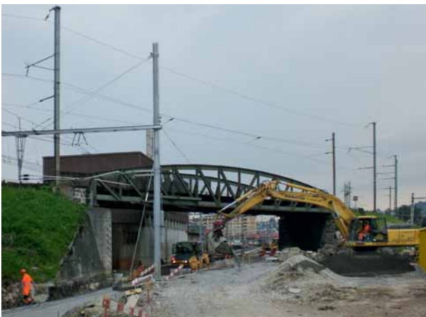
Fig. 9: New masts erected for overhead lines
