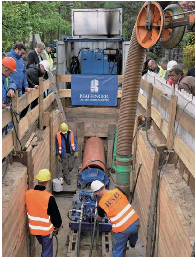
Fig. 8: The launch or assembly pit
