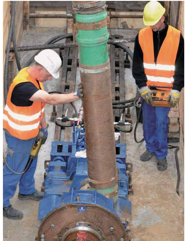
Fig. 10: Extraction by suction of the fed spoil
