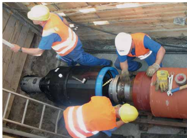
Fig. 9: Assembly of the first pipe to the reamer
