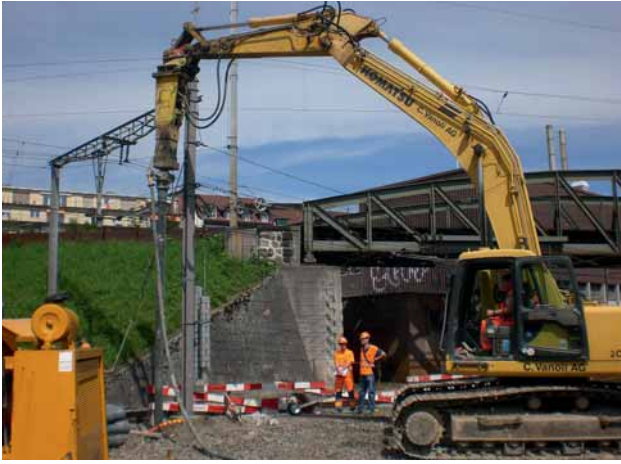
Fig. 7: The driven ductile iron piles being driven
