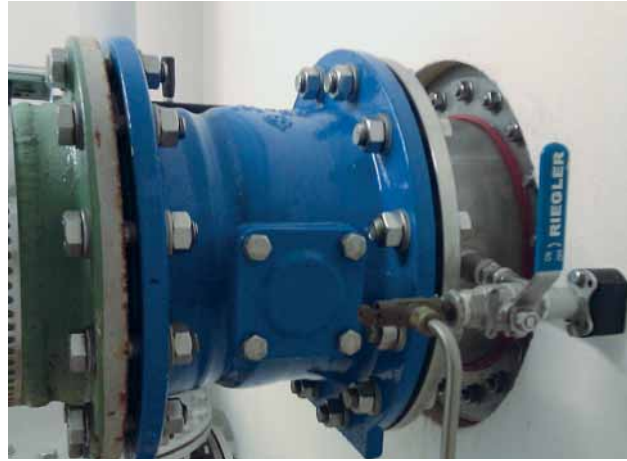
Fig. 2: Settling chamber outlet with sampling equipment
