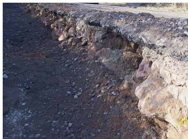
Fig. 4: Non-cohesive soil in the pipeline zone
