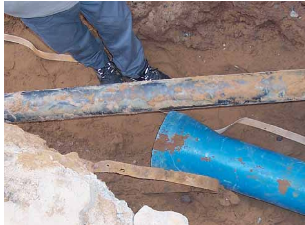
Fig. 3: A third-party pipeline along the route of the new pipeline
