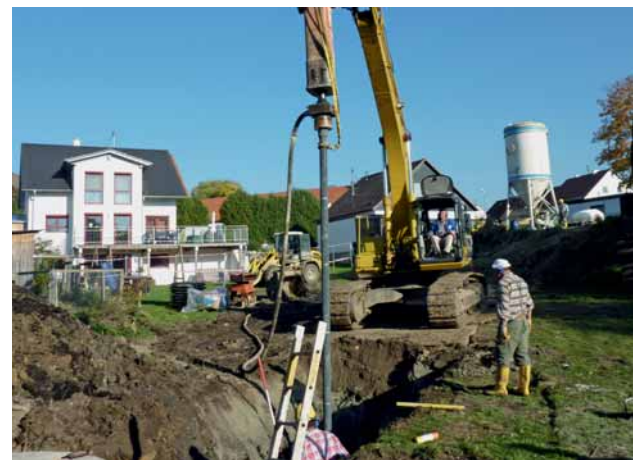
Fig. 8: Driving the 118 mm x 7.5 mm ductile iron piles
