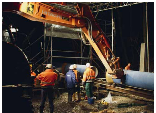
Fig. 12: Three-shift work – Work on the night shift
