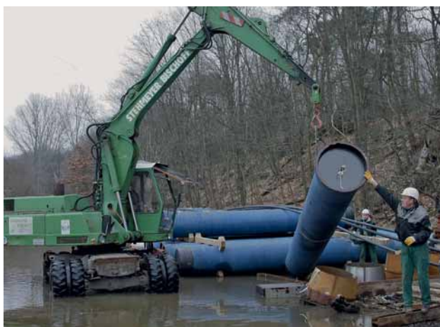
Fig. 5: High water on the Havel – Work in the flooded site area
