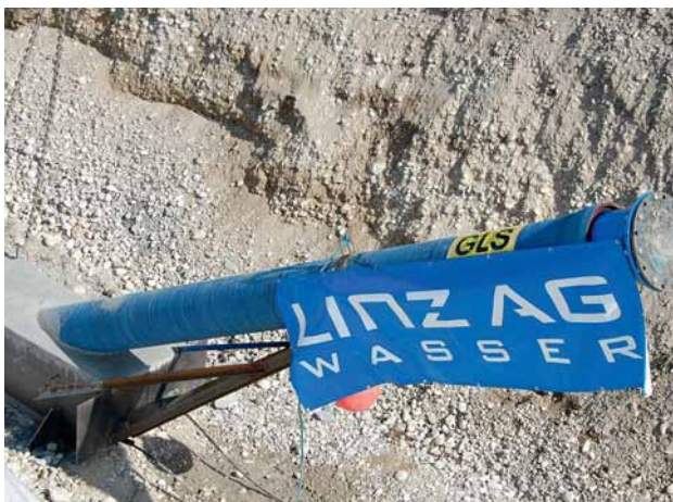
Fig. 3: The fully assembled culvert pipeline end section
