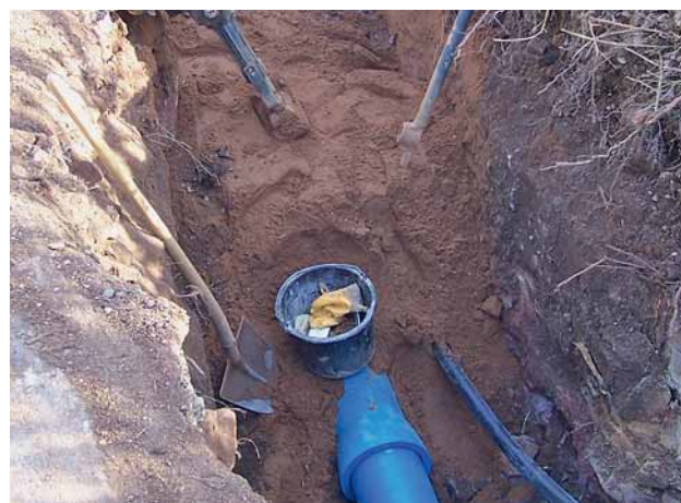
Fig. 5: Additional corrosion protection by a sand bedding
