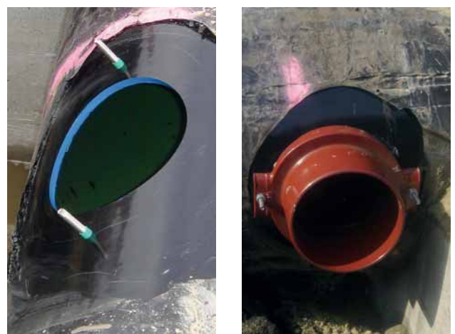
Fig. 9: Lateral connections are child's play to connect: On left: bored hole coated with epoxy paint On right: fully connected 90° tapping saddle
