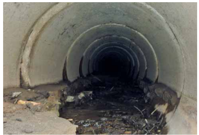
Fig. 1: The old concrete pipeline – the duct for the Schüttgraben stream
