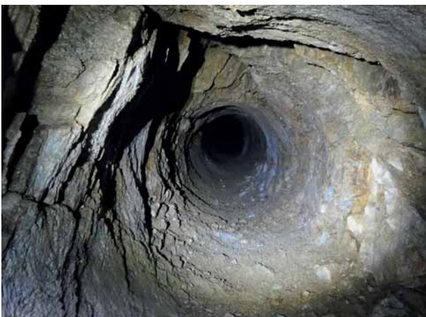
Fig. 5: The pipeline tunnel when bored, showing the sometimes friable rock
