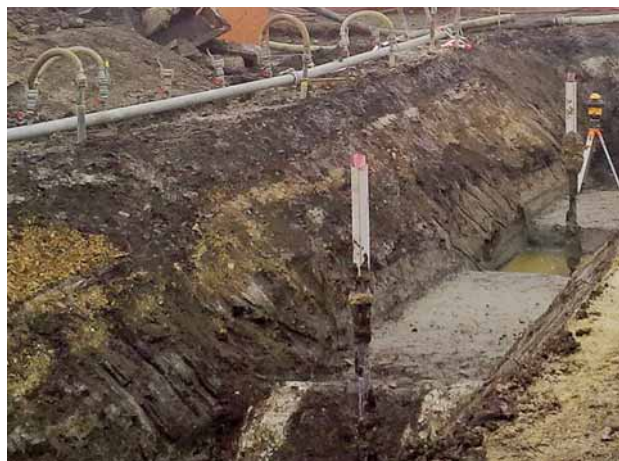
Fig. 3: Heads of piles projecting from the ground
