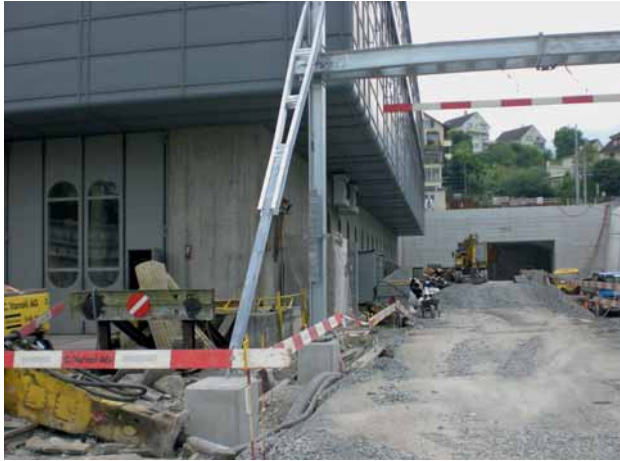
Fig. 12: Laying overhead line and anchorage footings
