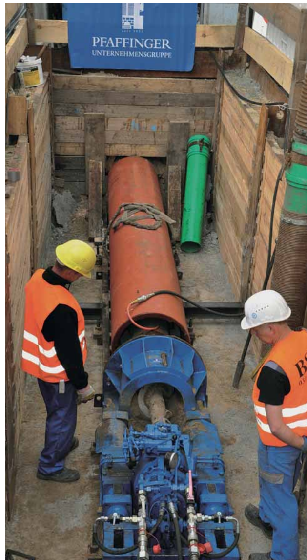
Fig. 2: The DN 300/DN 500 press-pull technique with soil removal
