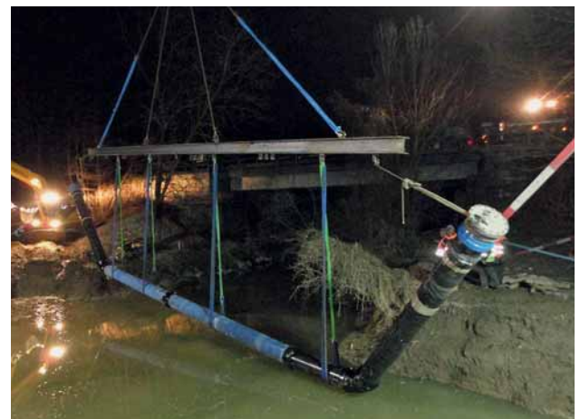
Fig. 4: A fully assembled culvert pipeline being lifted in – done under floodlights
