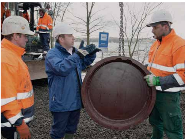
Fig. 9: Instruction by the pipe supplier's applications engineering department
