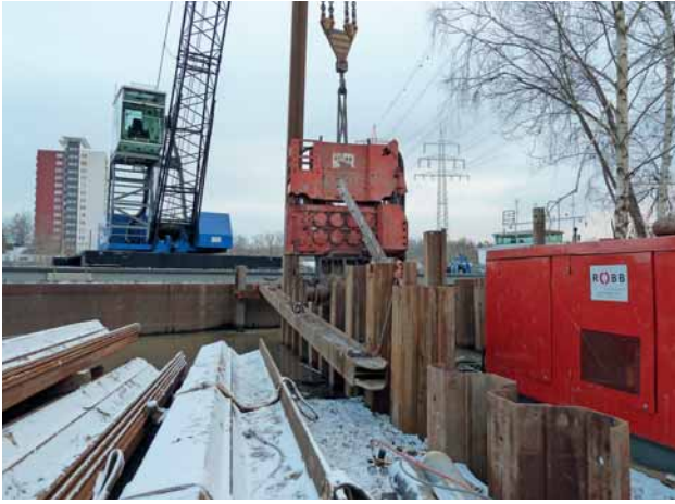
Fig. 3: Driving the sheet piling
