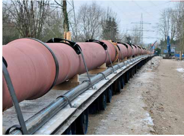
Fig. 5: The supporting structure on rollers
