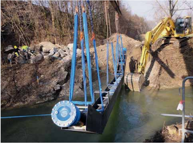
Fig. 5: A culvert pipeline combination comprising ductile iron pipes and a cradle of steel plate
