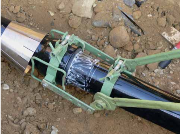
Fig. 3 A DN 125 push-in joint being connected on a burst lining project
