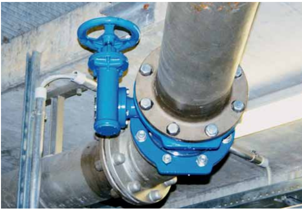
Fig. 4 Easier valve replacement due to the pulling tight of the loose flange – there is no need for the valve flange and pipe flange to be spread apart to fit the seal.
