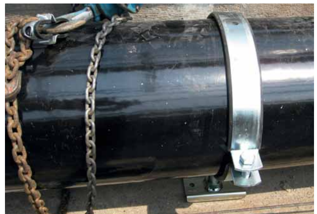
Fig. 6: A fixing point for the ecopur ductile iron pipe using a pipe clip with integral base plate
