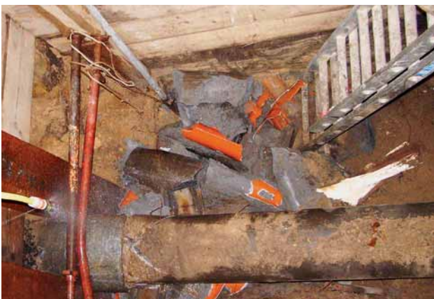
Fig. 5: The bursting process combined with the press-pull process
