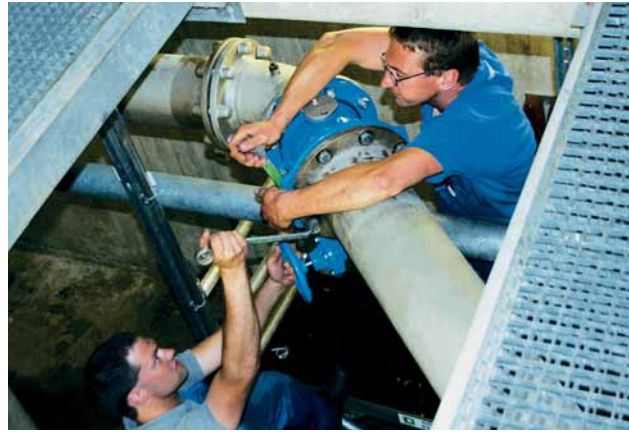
Fig. 5 Perfect positioning of the valve ensures excellent accessibility in all installation situations. It is even possible to subsequently turn the valve when it is installed.
