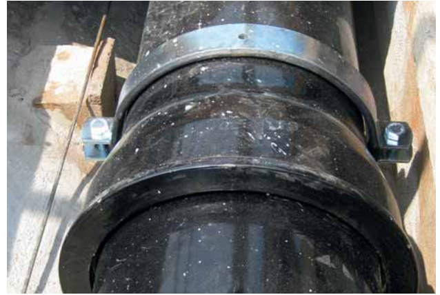
Fig. 5: Detail view of the hydrotight push-in joint in the narrow duct for the works pipeline
