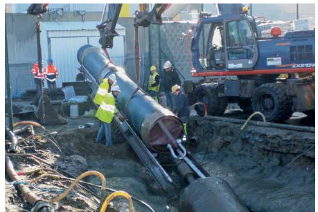
Fig. 6: Pipes being connected on a connecting ramp
