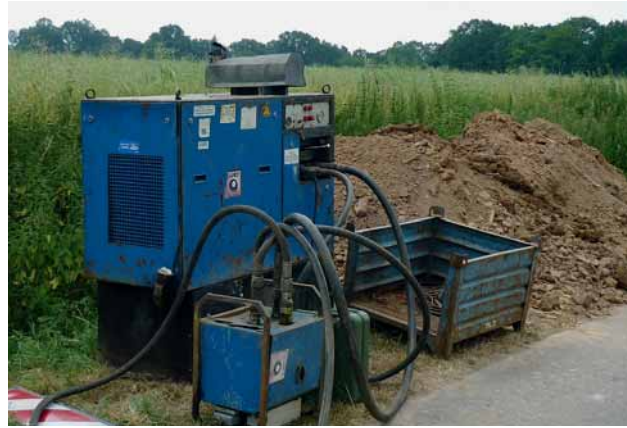
Fig. 3: The bursting system – the hydraulic unit to control the bursting rig
