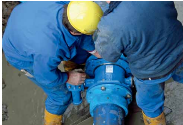
Fig. 6 Whether in plant construction or in a pipe trench – the dismantling type butterfly valve is the right solution everywhere.
