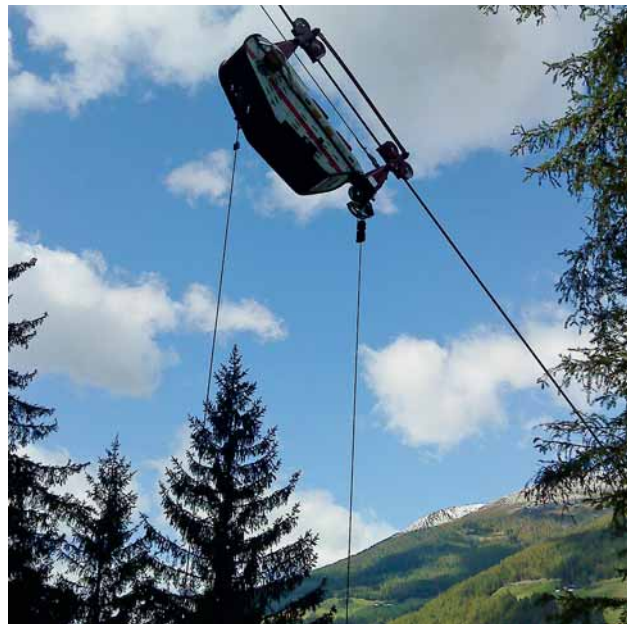
Fig. 6: Project 3 – The Furkelbach power station in South Tyrol: cable car with movable track cable
