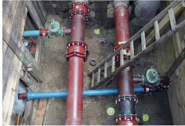
Fig. 7: Twin DN 250 ductile iron pipelines – open trench installation
