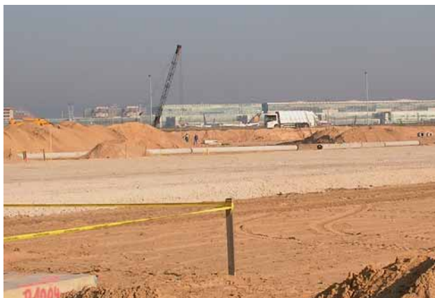
Fig. 1: The aprons of Terminal 3 under construction
