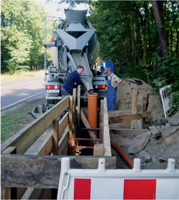
Fig. 4: Pouring in special mortar to fill the annular space
