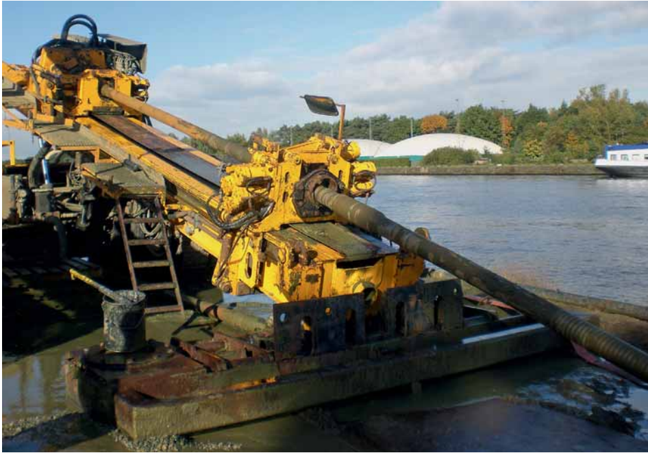
Fig. 4: 1000 kN drilling rig
