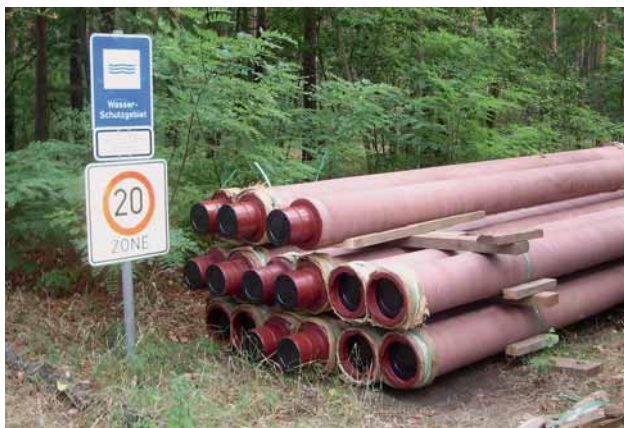
Fig. 1: Prepared for installation: special ZMU-PLUS ductile iron pipes with BLS® push-in joints
