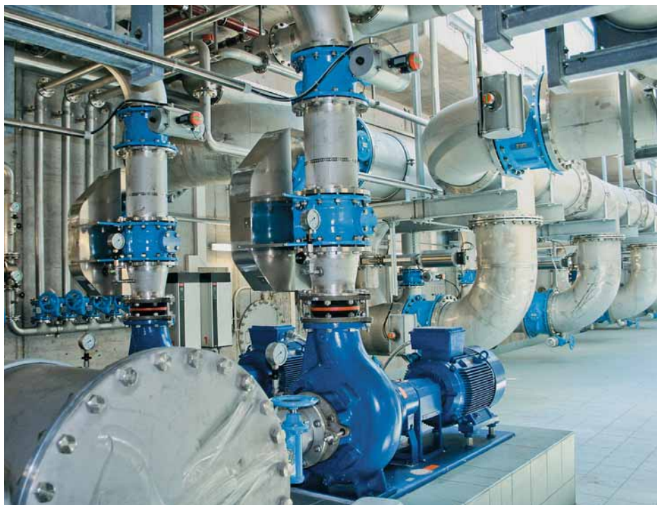
Fig. 2: DN 400 dismantling type butterfly valves – no problem to install in vertical pipes; no complicated supporting of the valve from below during installation because it is first fastened in place by its fixed flange when being installed.
