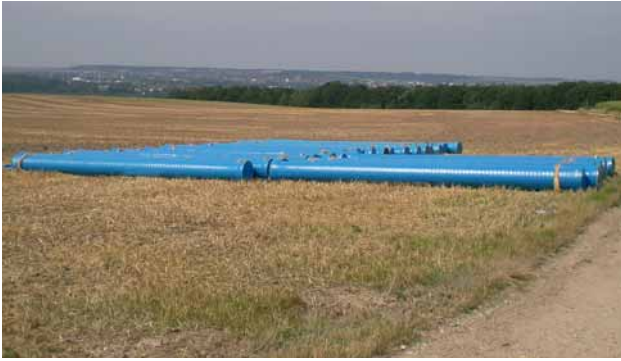
Fig. 2: DN 400 ductile iron pipes on the route
