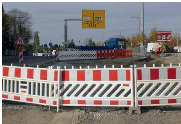
Fig. 1: Road building work on the “Mittlerer Ring Nord” ring-road in Leipzig
