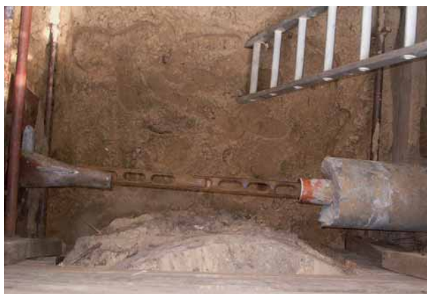
Fig. 3: Traction string guided in a plastic pipe
