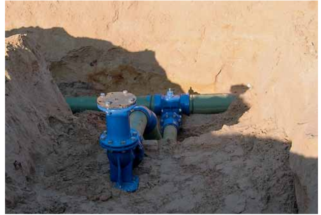
Fig. 5: Ductile iron fittings for making a connection to an underground hydrant
