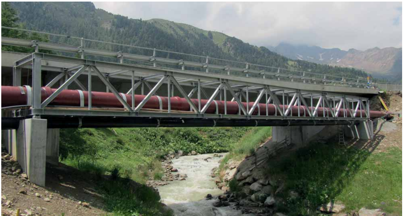
Fig. 3: Project 1 – The Vernagtsee power station in South Tyrol: a pipe bridge some 25 m long carrying a DN 700 penstock pipeline
