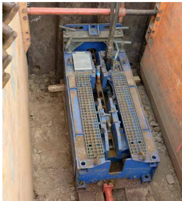
Fig. 4: A target pit containing a hydraulic bursting rig
