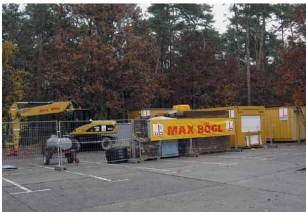
Fig. 1: The Max Bögl company's site equipment
