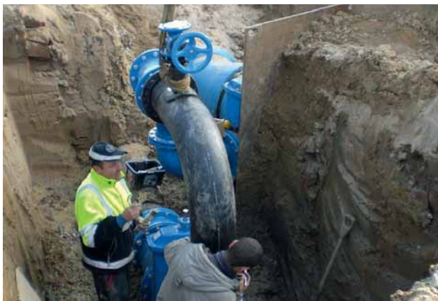
Fig. 3: Connecting up an interim pipeline
