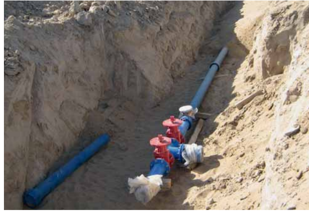
Fig. 6: Buried ring pipeline partially covered
