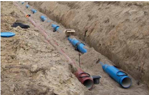
Fig. 4: Ductile iron drinking water and sewer pipes being installed in parallel
