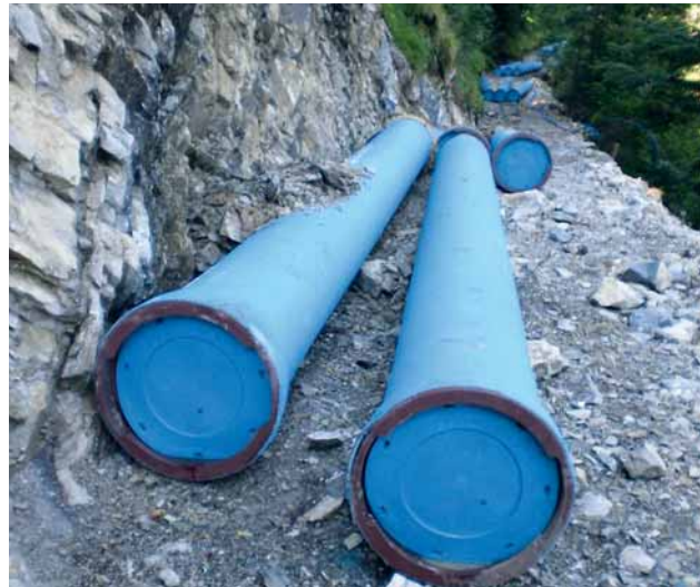
Fig. 16: DN 400 ductile iron pipes – on the cleared route across the slope
