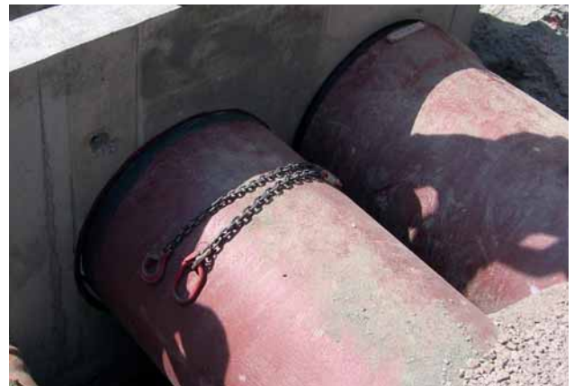
Fig. 11: Pre-cast reinforced concrete manhole with ductile iron manhole connections
