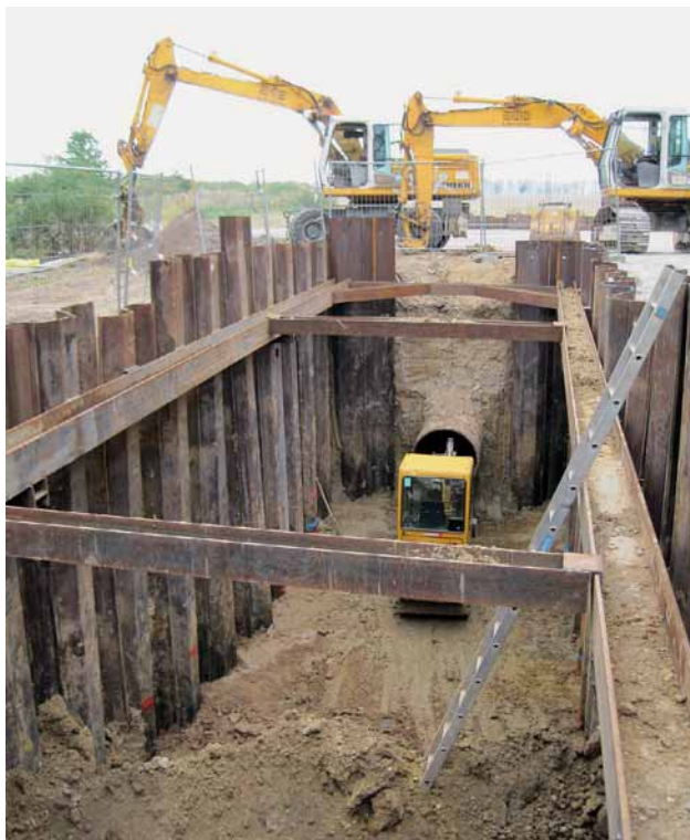
Fig. 1: Shoring of a trench with sheet pile shoring
