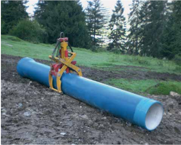
Fig. 18: A shortened ductile iron pipe with a welded bead applied by the layers
