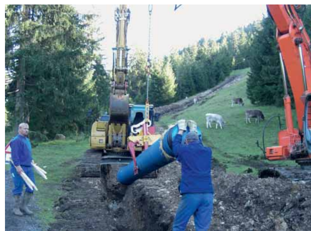
Fig. 6: Ductile iron pipes being laid on the ski slope at Kuhweide
