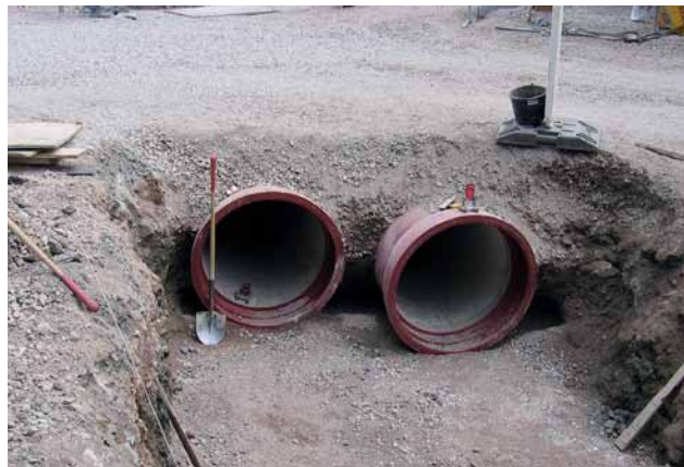
Fig. 7: The relief sewer (twin DN 1000 pipelines) covered with earth
