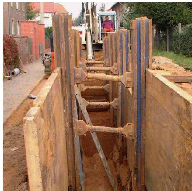
Fig. 6: Installation trench with slide rail shoring
