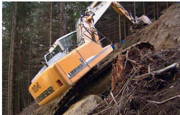
Fig. 2: The pipe trench being dug on a steep slope
