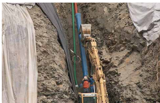
Fig. 4: Work being done on the turbine pipeline
