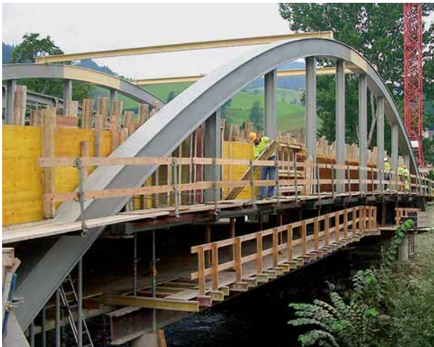
Fig. 1: The Rietwis bridge under construction
