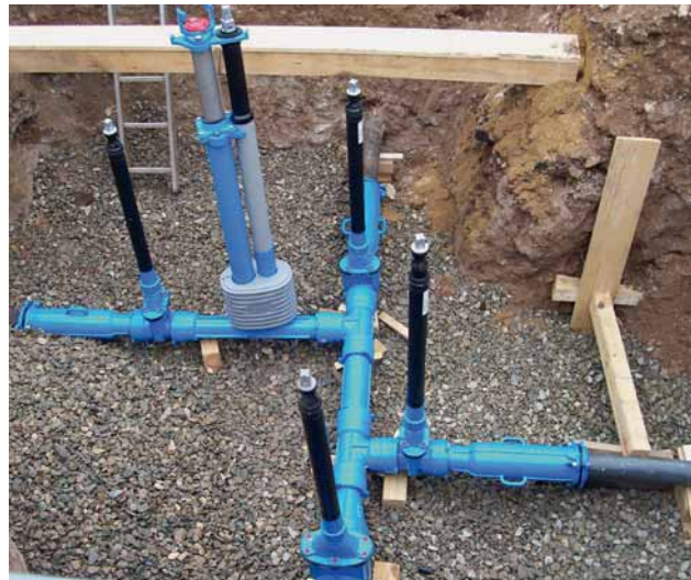
Fig. 5: The gate-valve equipped intersection after renovation
