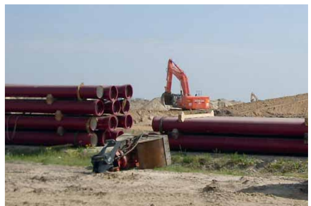
Fig. 2: Pipeline re-laying to prepare the construction site
