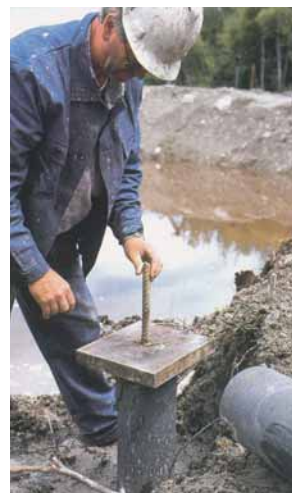
Fig. 6: The pressure distributing plate being fitted
