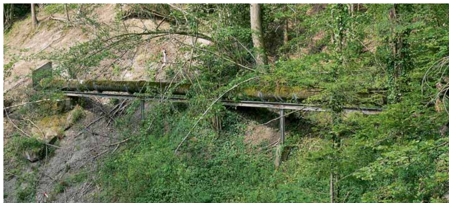
Fig. 1: The old “Gämpi” viaduct
