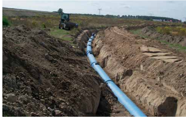
Fig. 5: A DN 600 drinking water pipeline in the Kienberg area
