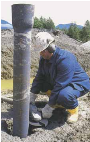
Fig. 2: Cutting off the projecting section of the pile
