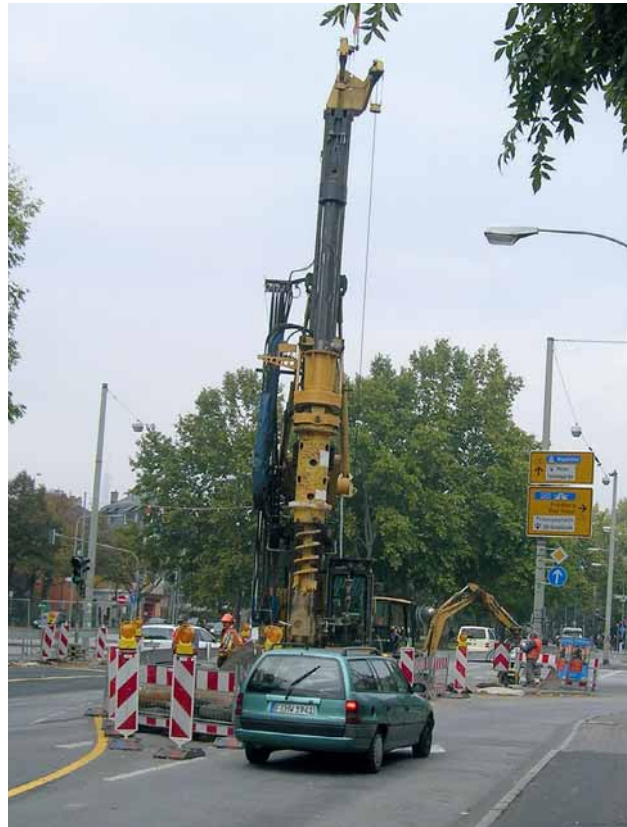
Fig. 3: Putting in the bore joist sheeting on the Nibelungenplatz
