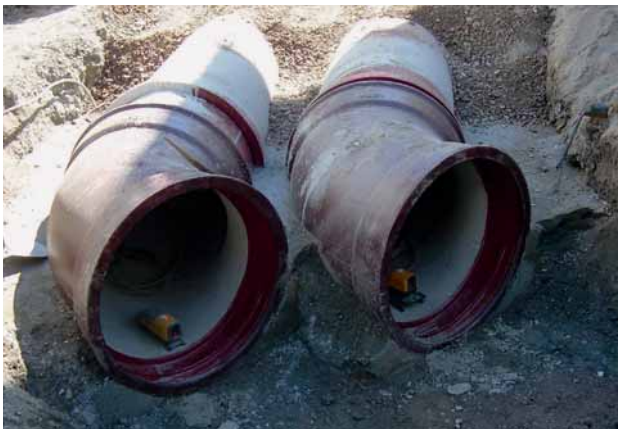
Fig. 9: Twin DN 1000 socket bends when installed
