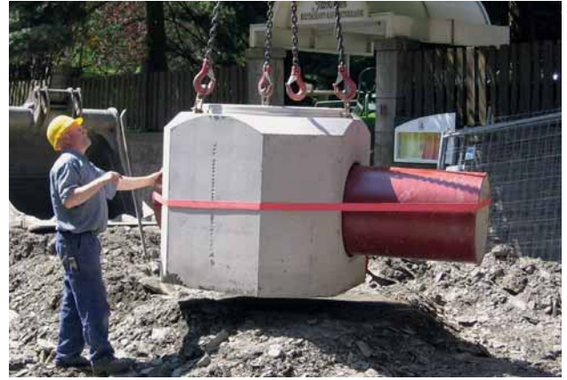
Fig. 10: Pre-cast reinforced concrete component with pre-fitted DN 500 ductile iron connector
