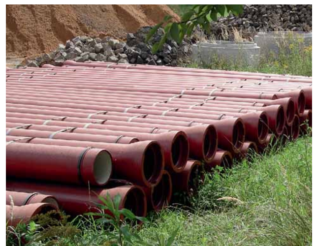
Fig. 3: Ductile iron pipes to EN 598 with TYTON® push-in joints
