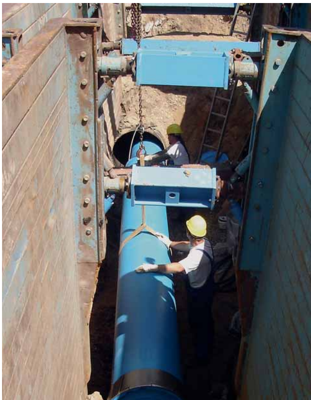
Fig. 4: Assembling of a DN 600 BLS® pipe
