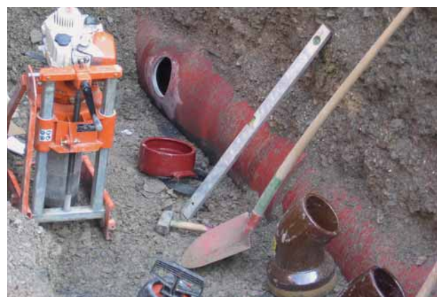
Fig. 12: House connections being made from the sewer with ductile iron saddles
