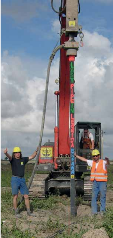
Fig 9: The last pile being driven at the Lebrija solar energy park
