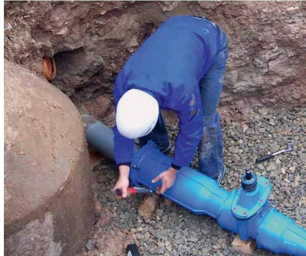
Fig. 4: A restrained connection to a pipe end
