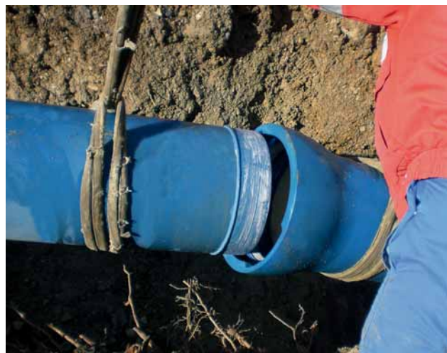
Fig. 17: Pipe ends being swung together
