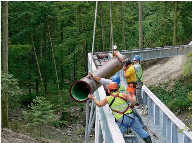
Fig. 5: The ductile sewer pipes being swayed in
