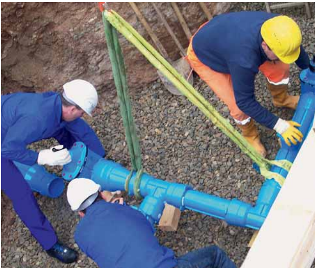
Fig. 3: Positioning the new gate-valve equipped intersection
