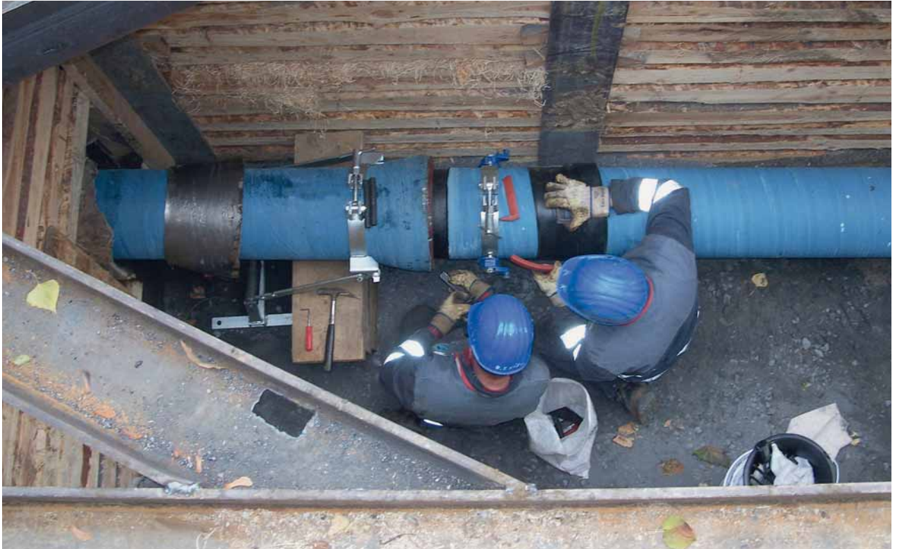
Fig. 4: Connecting a BLS® push-in joint
