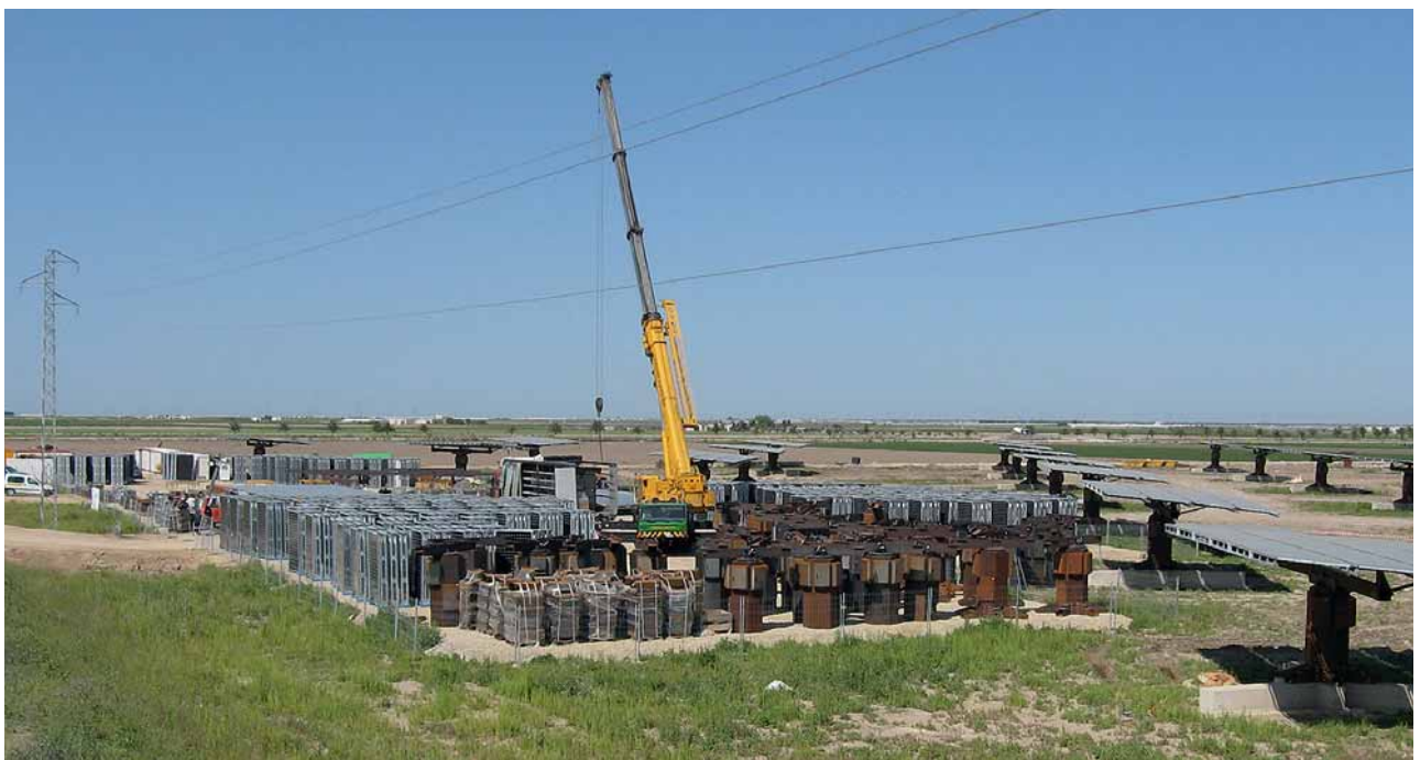
Fig. 8: Construction of the solar energy park in Lebrija
