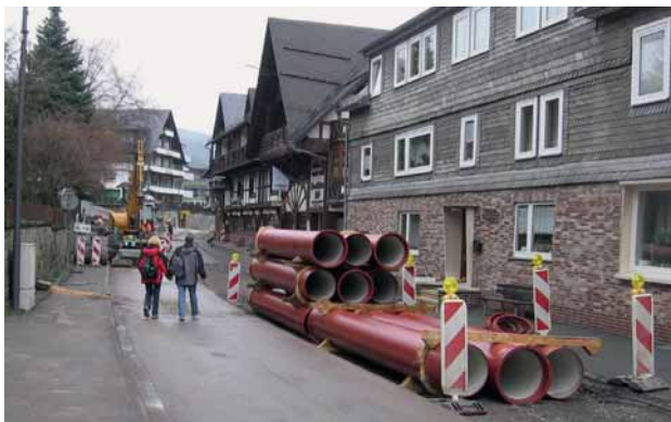
Fig. 2: Ductile sewer pipes lined with high-alumina cement mortar for internal protection and with a zinc coat and a top coating as external protection
