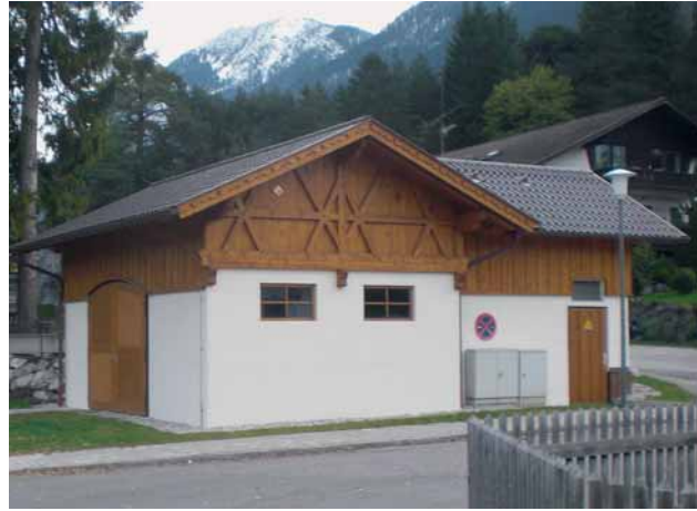
Fig. 4: The turbine house
