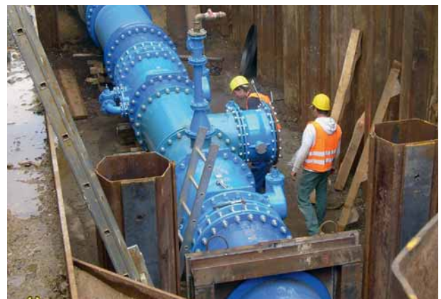
Fig. 3: Installation of a butterfly-valve-equipped cross
