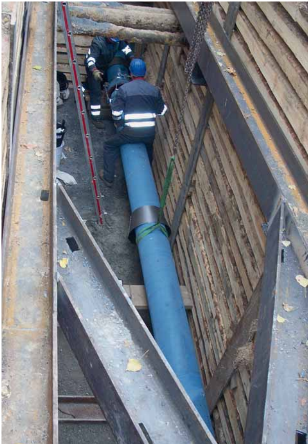
Fig. 5: Inserting the DN 300 ductile iron pipes
