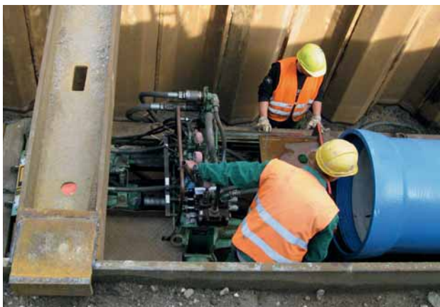
Fig. 2: A DN 900 TYTON®-pipe being pushed in
