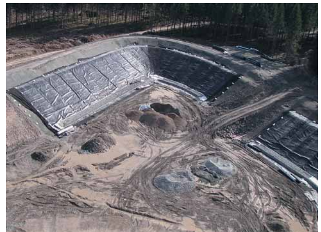
Fig. 3: The central reservoir being excavated
