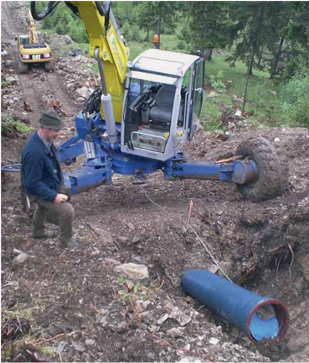
Fig. 14: A walking excavator in use
