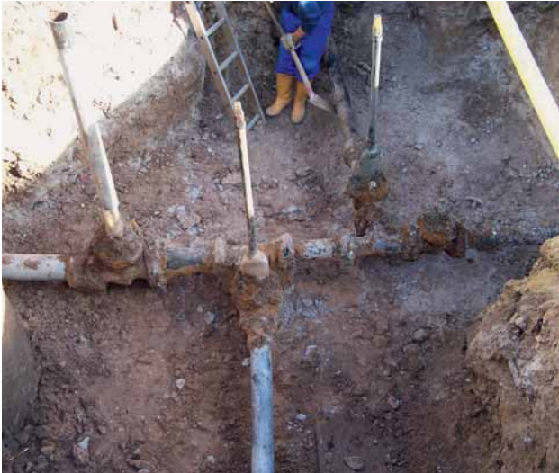
Fig. 2: The existing pipeline intersection
