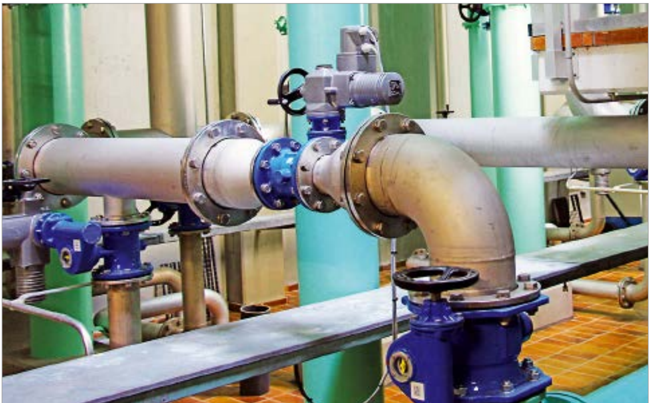
PAS10 dismantling joints, ERHARD ROCO wave butterfly valves with integral electric drive
