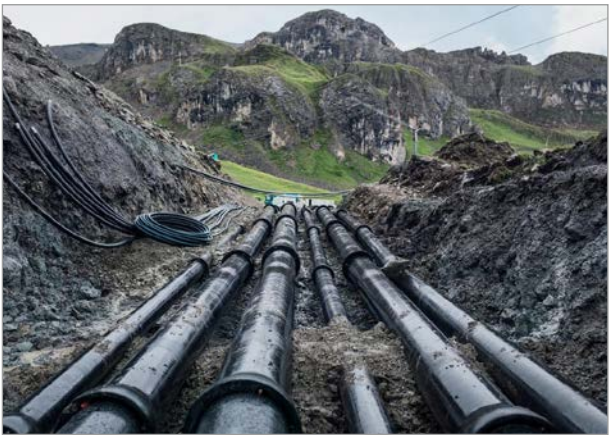
Figure 4: Installation of the filling and take-off pipelines in high-Alpine country
