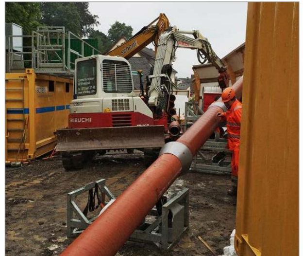
Figure 2: Assembling the pipes with socket guards before pulling in
