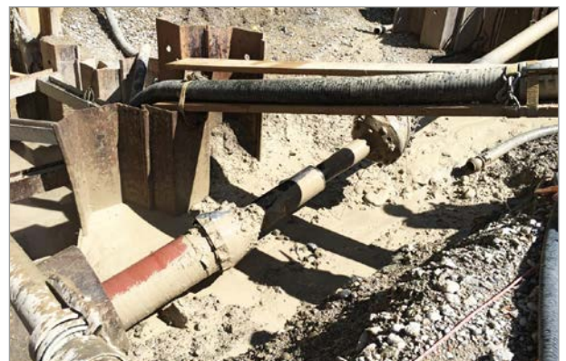
Figure 4: Upsizing head with the first pipe in the target pit
