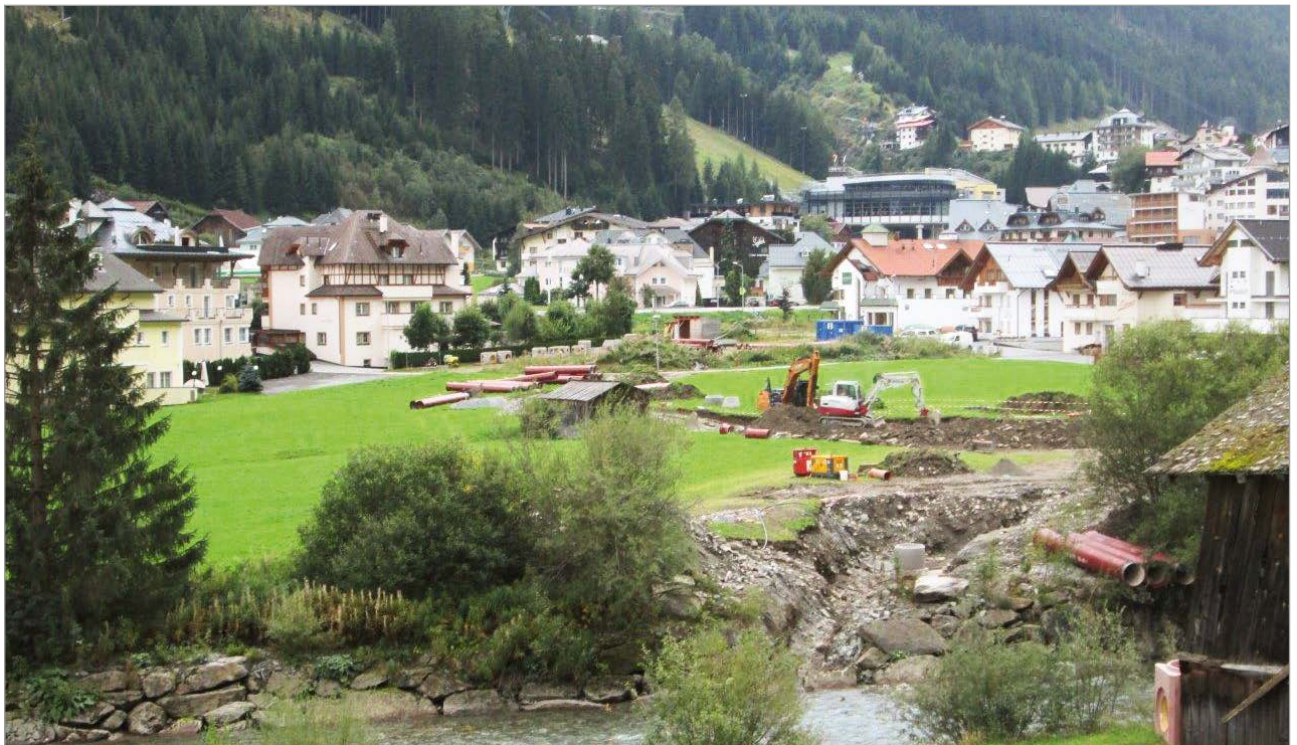
The route taken by the pipeline on the outskirts of Ischgl
