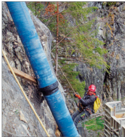
Full physical involvement in the steepest of terrains. The BLS® push-in joint from Hagenbucher can take the vertically acting tractive forces without problem. The pipes were flown in by helicopter.
