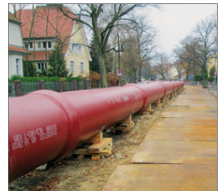
Pipe string with supports and steel plates laid out.
