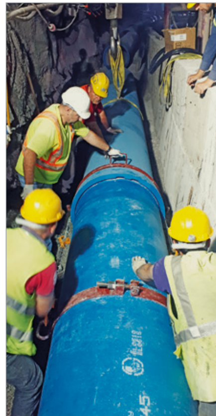
An assembly team installing a DN 800 pipe.
