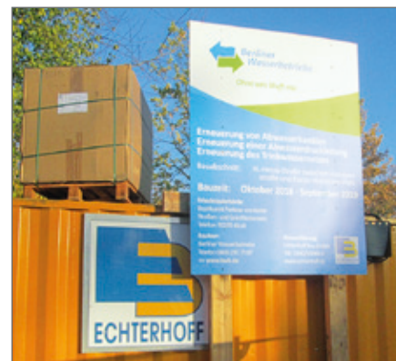
Construction site sign on Hermann-Hesse-Straße in Berlin Pankow.
