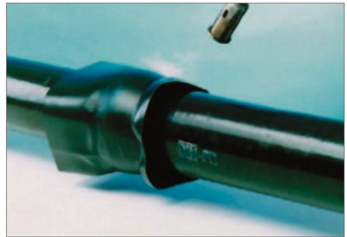
Application of a shrinking sleeve.
