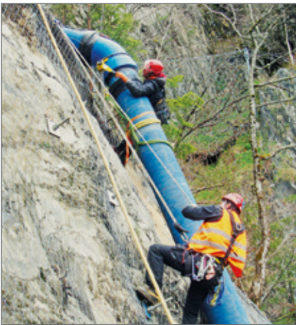
Full physical involvement in the steepest of terrains. The BLS® push-in joint from Hagenbucher can take the vertically acting tractive forces without problem. The pipes were flown in by helicopter.
