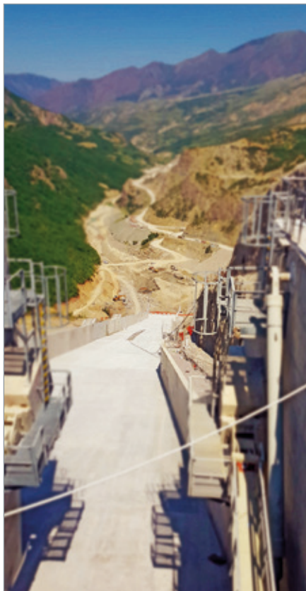
A view from the dam down to the emergency spillway.
