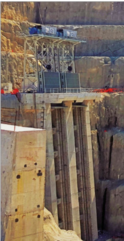
From the barrage wall to the headrace tunnel.
