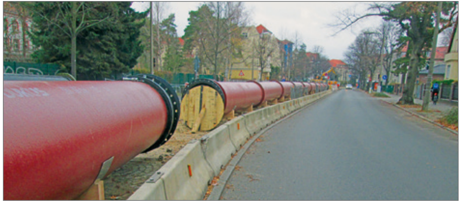
Tightness testing of the interim pipeline section by section.
