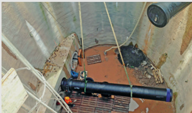
DUCPUR double DN 700 pipeline in the shaft, pulling into the micro-tunnel.
