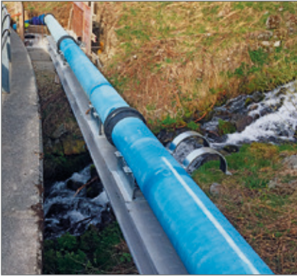
Open stream crossing with thrust blocks on both sides.
