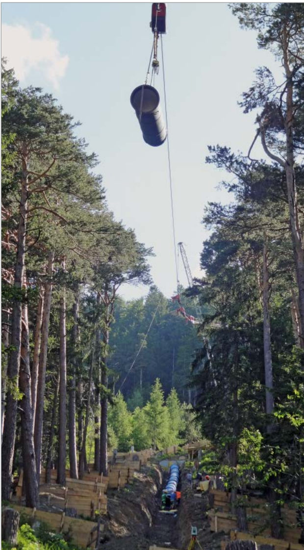
Figure 13: Pipe transport on the steep slope
