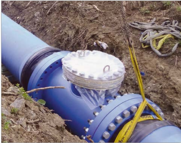
Figure 16: Access for cleaning and inspection
