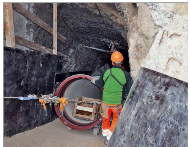
Figure 11: Pipe transport in the tunnel using transport rollers
