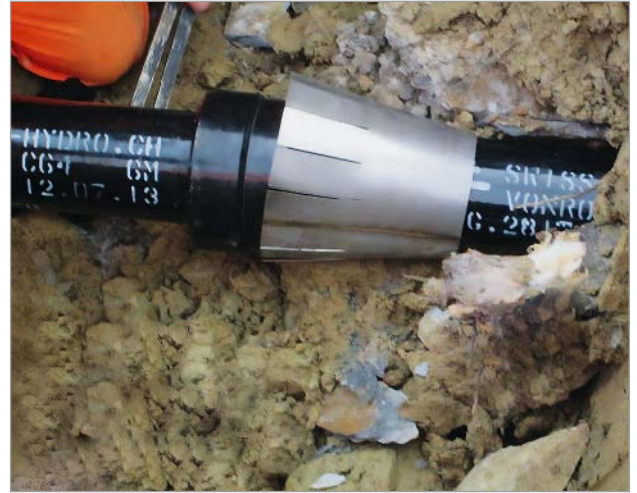
Figure 4: HYDROTIGHT push-in joint – installation using stainless steel sheet protective cones
