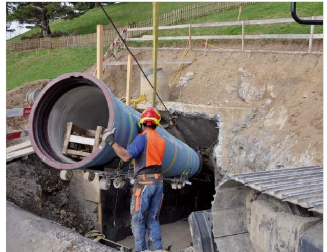
Figure 10: Roller support structure for transporting the pipes in the tunnel
