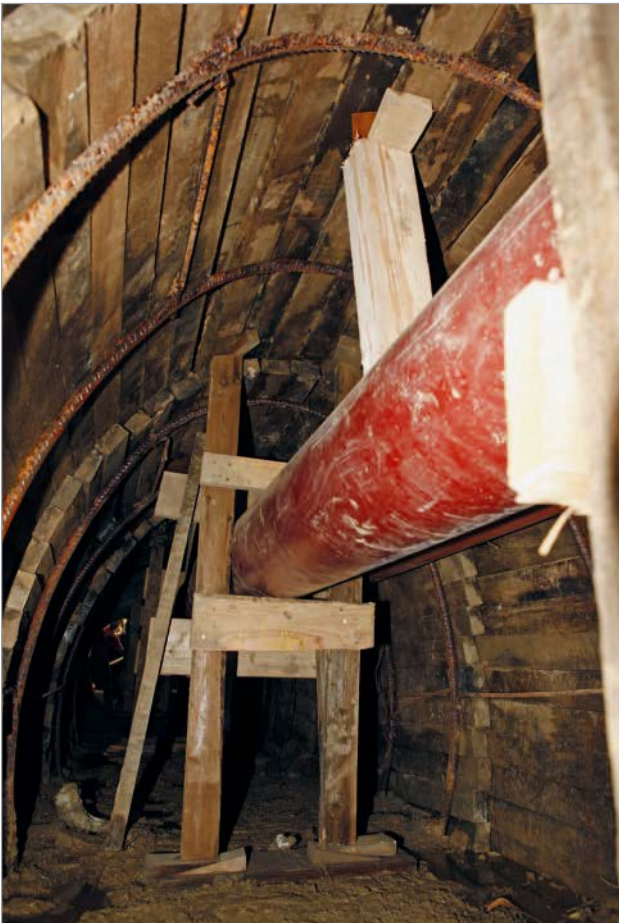
Figure 8: Fixing the assembled pipeline into position
