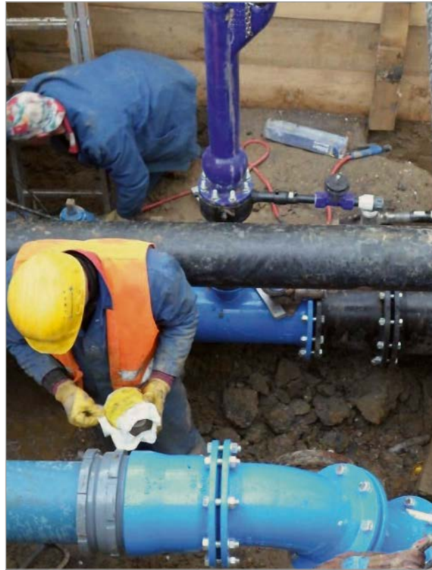
Figure 3: Installed Düker SPEZIAL flanged socket – screwed joint system with special clamping ring
