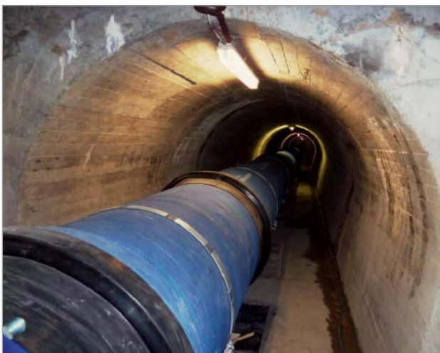
Figure 9: Surge chamber in the pipe tunnel
