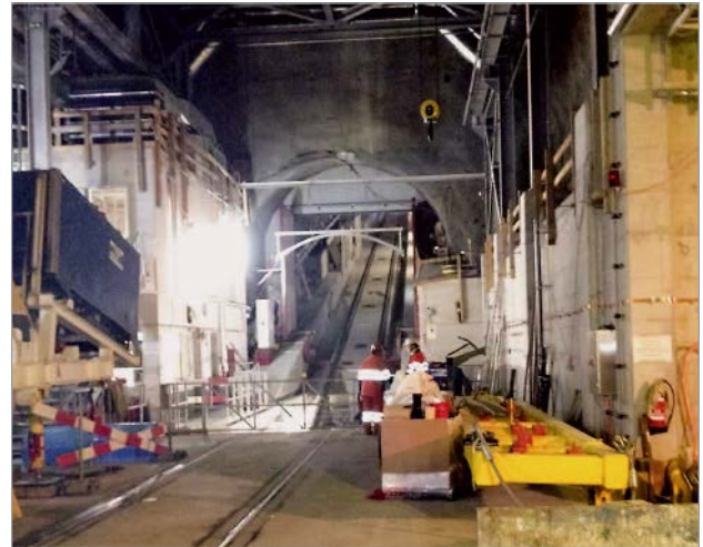
Figure 4: The transition from bottom station cavern to the sloping tunnel
