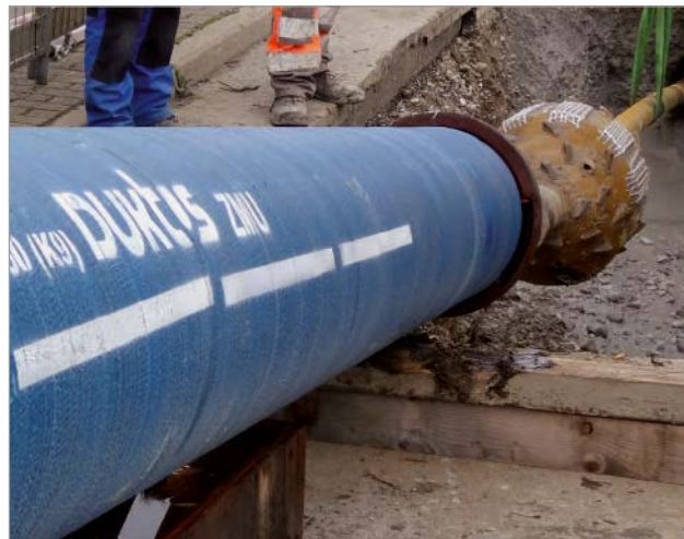
Figure 5: First ductile iron pipe with traction head and pull rods
