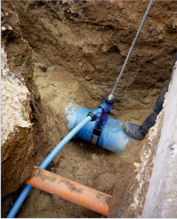
Figure 6: Commissioning a VAG TERRA®lock domestic connection valve in South Germany
