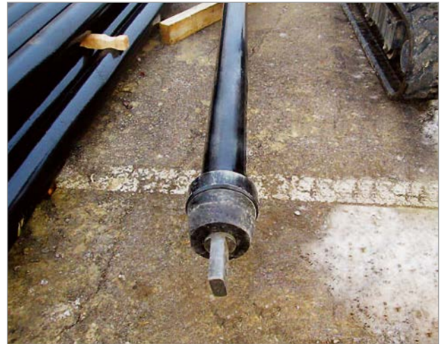
Figure 5: ECOPUR pipe with the traction head fitted and HYDROTIGHT push-in joint
