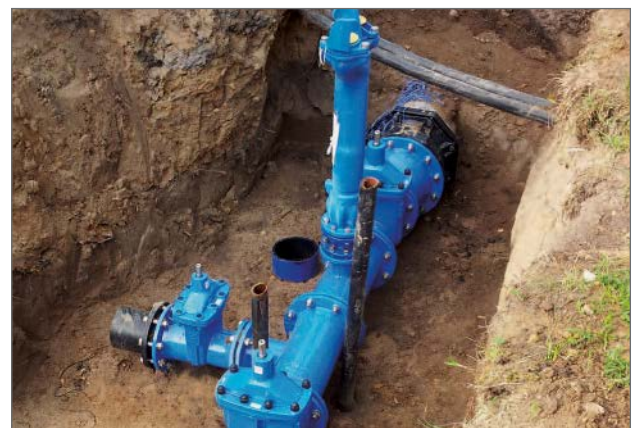
Figure 3: Installation of a new DN 150 drinking water pipeline
