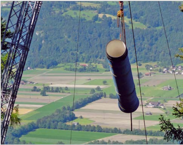
Figure 12: Pipe transport by cableway
