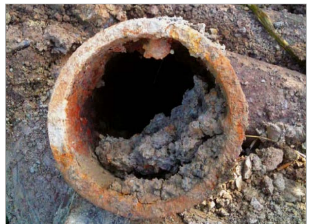
Figure 4: Dismantling the old connection pipeline
