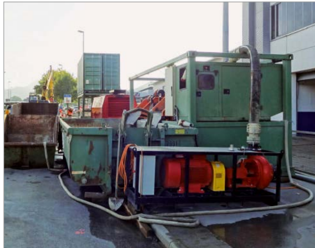
Figure 1: Mobile equipment for processing the drilling mud
