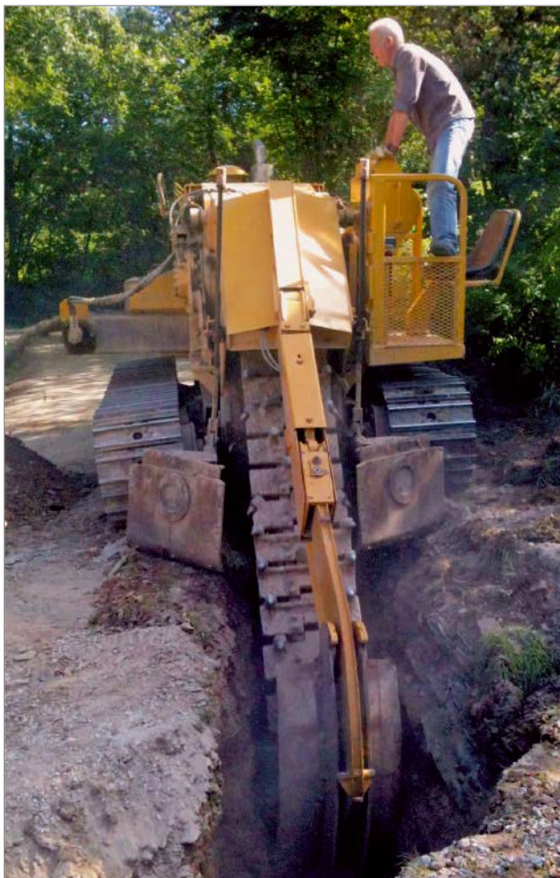
Figure 5: Use of a rock trencher
