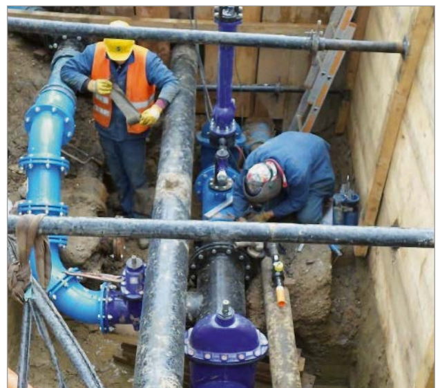
Figure 2: Internally enamelled all flanged tee, DN 300/DN 250/DN 200
