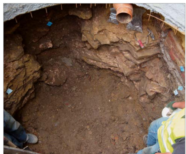
Figure 6: Launch pit with Carolingian brickwork
