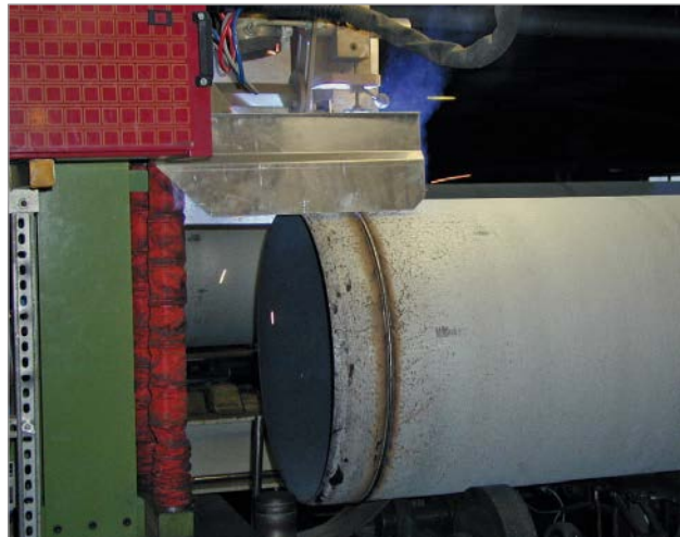
Figure 6: Welded bead applied at the factory
