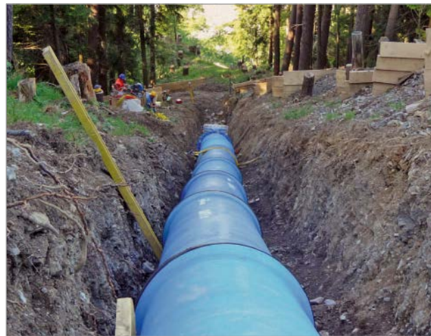
Figure 15: Pipe assembly on the steep slope
