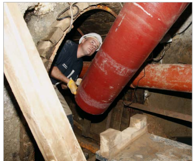
Figure 5: Threading the 3 m pipes into the gallery from the launch pit
