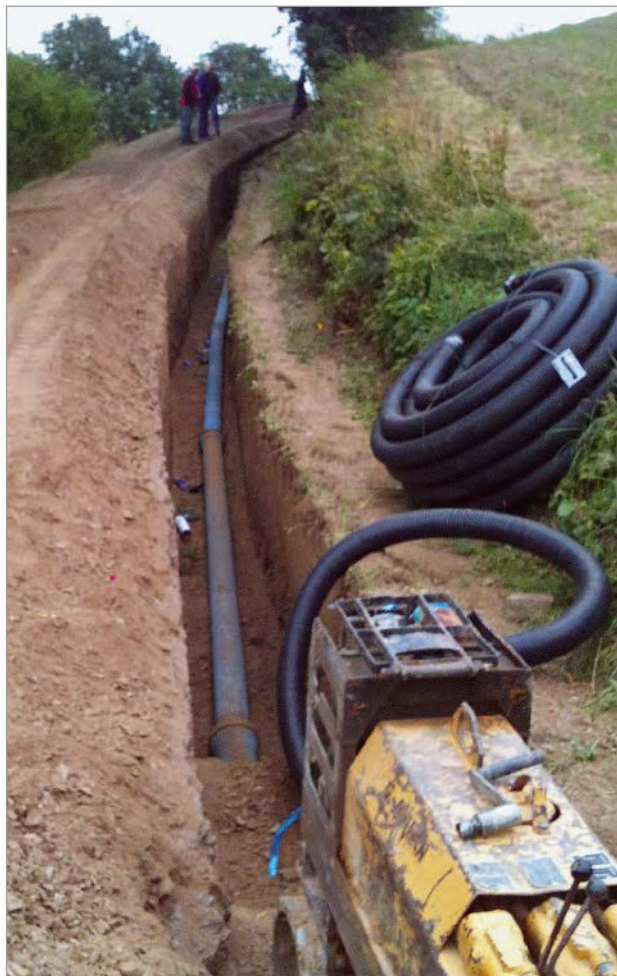
Figure 6: Installation of the reused emergency water pipeline and cable conduit
