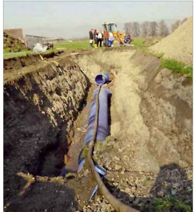
Figure 3: Installation of the DN 600 ductile iron pipes in the open trench
