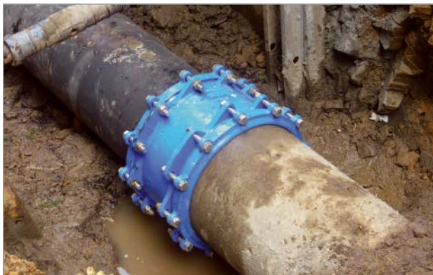
Figure 3: Installed U-Flex DN 500 adapter coupling
