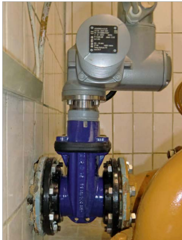
Figure 4: DN 100 replacement/repair valve with loose flange and short overall length to EN 558, basic series 14 [6]
