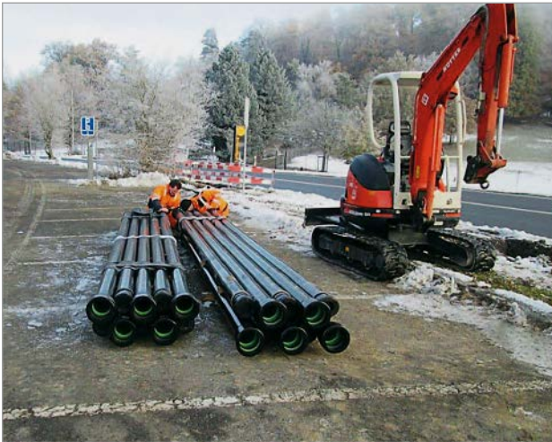
Figure 3: DN 125 vonRoll ECOPUR full-protection pipes – ready for installation on the roadside
