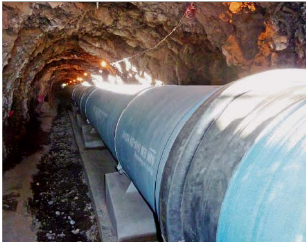
Figure 8: Masescha pipe tunnel
