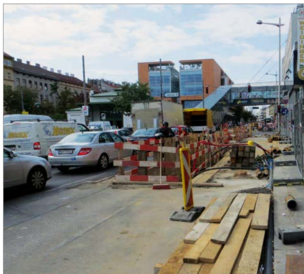
Figure 2: Maintaining the flow of traffic – implementation of the Wiener Wasser traffic concept
