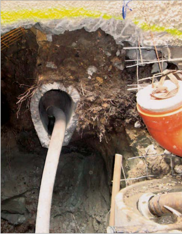
Figure 7: Existing pipeline in the crown of the gallery
