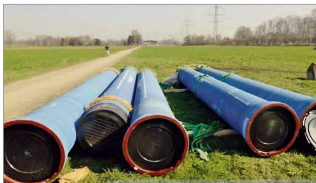
Figure 2: DN 600 ductile iron pipes for installation as a bypass pipeline
