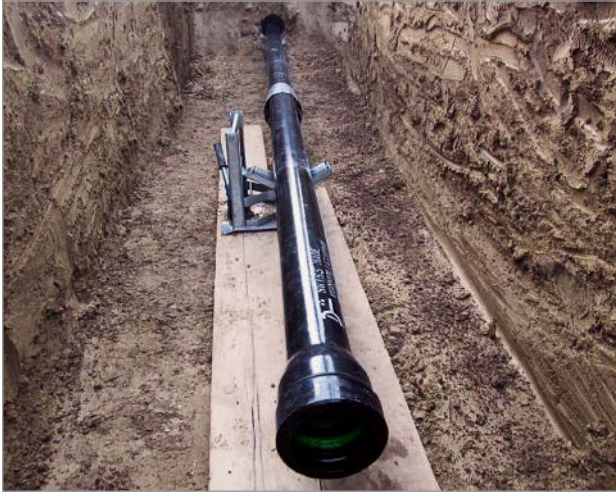
Figure 9: Pulling the ECOPUR pipes in the launch pit
