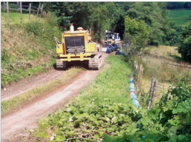
Figure 3: Installation of the DN 150 GGG emergency water pipeline
