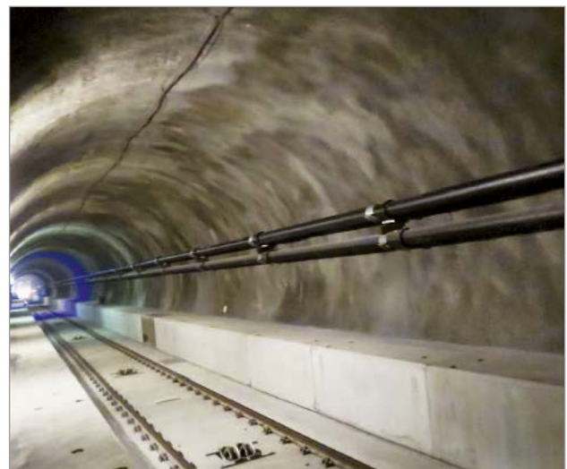
Figure 5: Pressure pipelines installed in the sloping tunnel (with sliding consoles)
