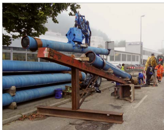
Figure 3: Pipe store, launching ramp, launch pit and intermediate construction pit
