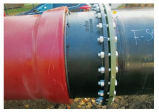
Flanged spigot assembled in the pipe socket using the BLS<sup>®</sup> system.
