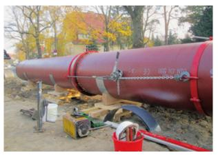
Assembled BLS® joint with pipe supports.
