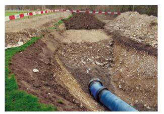
The different types of soil are clearly visible, but the ductile iron pipe with cement mortar coating is up to any situation. Unpolluted excavation material can also be used again for backfilling the trench.
