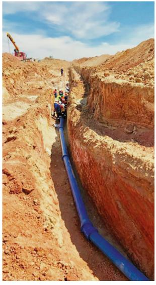
Temperatures as low as -40°C, which prevail in the Mongolian winter and cause the ground to freeze to a depth of up to 3.5 m, make it necessary to lay the pipes 4 m deep.
