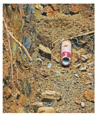
The geological and tectonic conditions in this region make it prone to landslides. The use of ductile iron pipes with cement mortar coating was therefore a "must".
