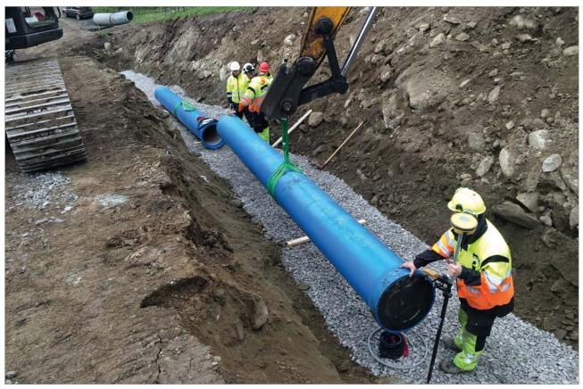
Installation of ductile iron pipes as the turbine pipeline for the Storelvi hydropower station
