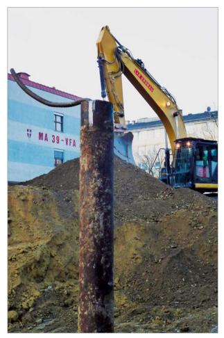
Cast iron driven pile revealed after 30 years
