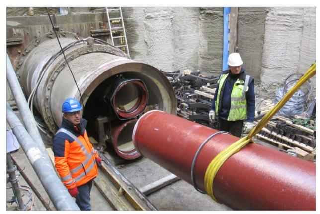
Installation of a DN 600 ductile iron pipe with a BLS® restrained push-in joint
