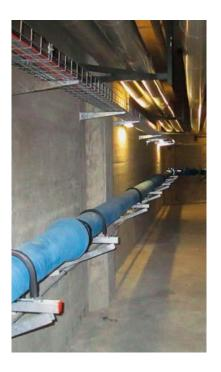
some adaptor fittings had to be produced and in each case welding beads had to be applied on the spigot ends to produce the positive locking joints. After a short running-in time, the work was carried out quickly and to a high quality standard.
