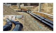
superior material properties these have a very high static load-bearing capacity. 550 m of DN 350 ECOPUR type ductile iron pipes were installed with integral lining and coating of polyurethane (PUR) to EN 545. The entire length of the pipeline is designed to be thrust resistant with the proven vonRoll HYDROTIGHT restrained joint system.
