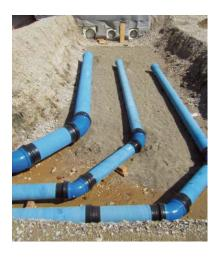
♦ In the process of the construction of a new elevated tank for the supply of drinking water to the municipality of Markt Mering in the Swabian district of Aichach-Friedberg, a few pipelines also had to be partially replaced. Because the pipelines were buried at a depth of up to 6 m, the client decided in favour of ductile iron pipes with an increased wall thickness and cement mortar coating. Re-
