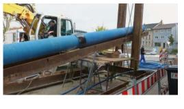
installed during the course of restructuring and reorganising the water supply were a further 288 m of DN 400, C 40, K 9 ductile iron pipes with TYTON SIT PLUS® push-in joints. The construction work commenced at the end of August 2015 and was completed by December 2015.
