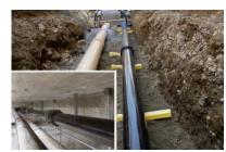
as ECOFIT fittings with integral epoxy coating to GSK/RAL-GZ 662, classified as a reinforced coating according to EN 545. The new 600 m long ECOPUR DN 200 drinking water supply pipeline was equipped with the proven HYDROTIGHT thrust resistance system along its whole length.
