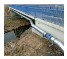
tions and because of its geographical position, the pipeline was designed with a pressure of up to PN 40; a pumping station and four water towers were included in the project. Because parts of the pipeline route run through stony ground, ductile iron pipes with a cement mortar coating and BLS® joints were selected. Bridges were used for river crossings, where pre-insulated ductile iron pipes were applied.
