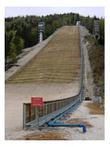
restrained push-in joints also meant that installation above ground was possible.
