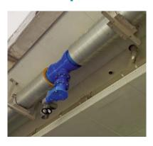
especially converted for this application the pipes were lifted up and installed. The longest thermally insulated cast iron pipeline delivered to date by the pipe manufacturer was completed with an average installation rate of 6 pipes a night.
