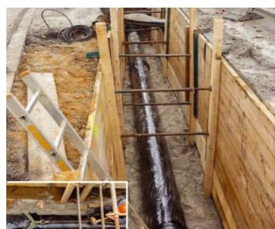
decided to install vonRoll ECOPUR full-protection pipes in ductile cast iron with a reinforced coating to EN 545 in one approximately 200 m section. The vonRoll ECOPUR push-in pipes are fully protected with a non-porous internal and external coating of polyurethane (PUR) and can therefore be used even in highly aggressive soils.
