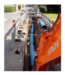
through a built-up urban area. Manual operation pits plus numerous crossings of the route were part of the work on this construction project. The replacement began in August 2014 and was completed to deadline in October 2014.
