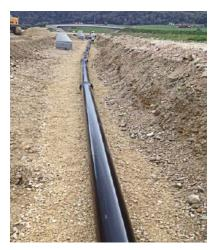
friction locking. The system is completed by vonRoll ECO-FIT fittings with integral epoxy coating to EN 14901. The high points of the transport pipeline were equipped with aeration and ventilation valves. Drainage was installed at the low points. For convenience of operation, the air valves and drainage fittings were installed in concrete shafts.
