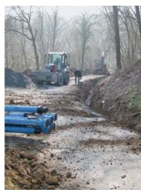
The 2,260 m long pipeline in DN 100 ductile iron pipes with cement mortar coating and TYTON SIT PLUS® pushin joints was predominantly installed outside built-up areas.
