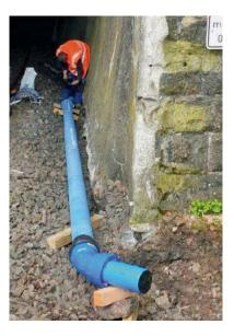
The planned delivery capacity was set at 800 l/min and the static pressure in the pipeline is 8 bar. The flow pressure when taking off extinguishing water needs to be 5 bar. 624 m of DN 125, BLS®, K 10 ductile iron pipes with cement mortar coating and FCM combisleeves were installed. FM approval has been obtained.
