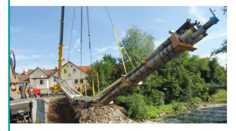
◆ For a crossing over the River Murr the utilities department at Backnang packaged one water supply pipeline in DN 200 ductile iron pipes, two DN 200 gas pipelines in steel,
