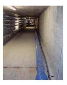
name. Here there are 2,200 m of DN 200 ductile iron pipes with PUR coating in a service gallery under the roadway, which also houses all other infrastructures. The work is in full swing; a major part of the fire-extinguishing water pipeline has already been completed under the leadership of the Atzwanger AG company from Bolzano.
