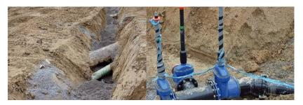
Parallel to the new road construction, a new water transport pipeline has also been laid by the water supply cooperative of Neuenkirch. The total length of the new vonRollecopur ductile pipeline is 850 m, with 580 m DN 200 and 270 m DN 150, K 9. In addition VS5000 fullprotection gate valves with integral thick epoxy resin coating to RAL GZ 662 and, for the extinguishing water requirement, 5000S vonRollhydrants with the VARIO lower part were used. The choice
