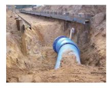
◆ The maximum operating pressure of the pipeline is 9 bar. The construction of an embankment is planned for the road in the area of the crossing, which would be built over the existing trunk main to a height of about 5.0 m. Therefore Hessenwasser has moved a length of around 145 m of its drinking water pipeline out of the danger area of the embankment. For safety reasons, Hessenwasser decided
