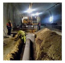
The rainwater which occurs is collected and pre-cleaned upstream of the tunnel in a settling basin for rain. The water having been cleaned in this way, a pumping station then feeds it along a 540 m long pressure pipeline of DN 200 ductile iron sewer pressure pipes with BLS® restrained push-in joints and into the river Rems, which acts as a receiving water. All the ductile iron pipes installed are coated on the outside with zinc and epoxy and are lined with cement mortar.
