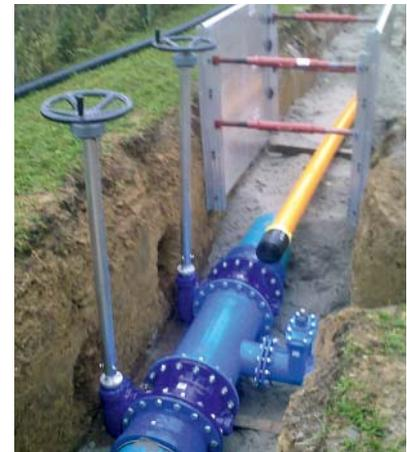
DN 100 pillar hydrants are provided every 90 m for the take-off of fire-fighting water. Given that there is an earth cover of 1.70 m, the pipeline trench is safely supported by shoring. Because there have been a number of fractures in the existing water pipeline, this is being replaced as well in the course of the installation of the pipeline for fire-fighting water. Some 200 m of DN 200 ductile iron drinking water pipes are being used for this. During
