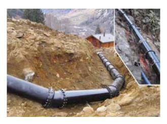
sure is 23 bars. The polyurethane coating of the ecopur pipes is classed as a reinforced coating under EN 545 and proved to be extremely rugged in this difficult terrain. The pressure pipeline system was subjected on site to a leak test at a test pressure of 32 bars for 24 hours. After a construction period of only 16 months, the small hydroelectric power station went into operation in June 2012. Its current output is 1,700 kW.
