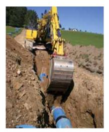
additional operations and transport work to be dispensed with. In view of the geodetic difference in height, the pipeline was designed for an operating pressure of PFA = 25 bars and it was tested at 30 bars before going into operation.
