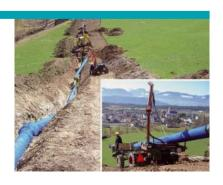
moved to the trenches by an off-road all-wheel drive agricultural vehicle which had been fitted with a crane to convert it into a special-purpose vehicle. This vehicle had to be secured by a forestry cable winch. The easy assembly of the pipes meant that only a short installation time was needed.
