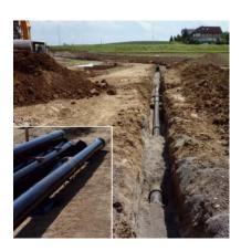
restricted space for the routeing of the trench in the area to be built on meant that large numbers of vonRollecofitfittings with an integral epoxy coating to EN 14901 and RAL GZ 662 were also needed. All in all, everyone involved in the project - the client, and pipe-layers engineers considered the vonRollecosys fully protected ductile iron system with the vonRollhydrotight push-in joints extremely easy, time-saving and safe to install and were together very pleased with how it all went.
