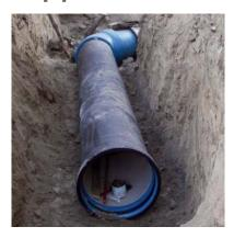
cult sections of terrain along the route,1,500 m of DN 800, PFA = 25 bar, ductile iron pipes and fittings with restrained BLS® push-in joints were supplied and installed. In spite of the difficult terrain, with its steep slopes, rocky ground and lack of space along the route, the installation of the pipeline went off without a hitch.
