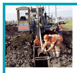
◆ The water supply utility Wasserverbund Großes Moos is laying a new transporting pipeline to connect its two water distribution networks. vonRollecopur DN 300 fully protected pipes with push-in joints have been used for this pipeline. The pipes, of wall-thickness class K 9, have a reinforced coating to EN 545, a PFA of 16 bars, and integral polyurethane internal and
