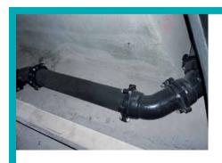
◆ As part of the "Lungern Tunnel" project a hydrant pipeline is being installed in the tunnel verge on the uphill side of the tunnel to give assured fire protection. The pipes being used are vonRoll-ducpur DN 200 K 9 ductile iron pipes with a minimum wall thickness of 4.7 mm, a polyurethane lining to EN 15655 and a zinc/bitumen coating. Thanks to the flexibility of the
