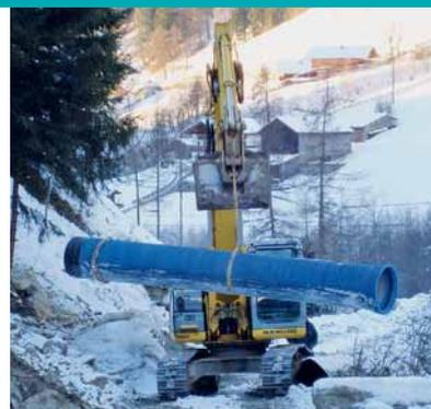
December 2009. In December the installation site was a completely wintry scene. However, ductile iron pipes can be installed in below-zero temperatures, snow, and ice. The refurbished small hydroelectric power station at Walten went back into operation in the spring of 2010.
