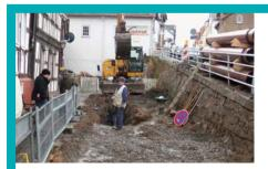
• For hydraulic and structural reasons, the existing sewer running along the Glockenstraße needed to be replaced. The sewer pipes, which were more than 50 years old, had only a shallow height of cover and contained cracks and
