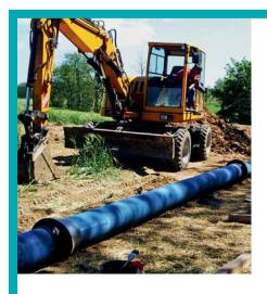
◆ On the island of Rügen in the Baltic an old DN 300 asbestos cement pipeline needed to be rehabilitated. Its route ran through marshy land and across a deep gulley along which a stream ran. The client, the water supply utility 'Zweckverband
