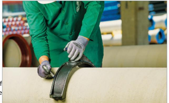
The cement mortar layer is partially removed for attaching the TRM tapping sleeve.
