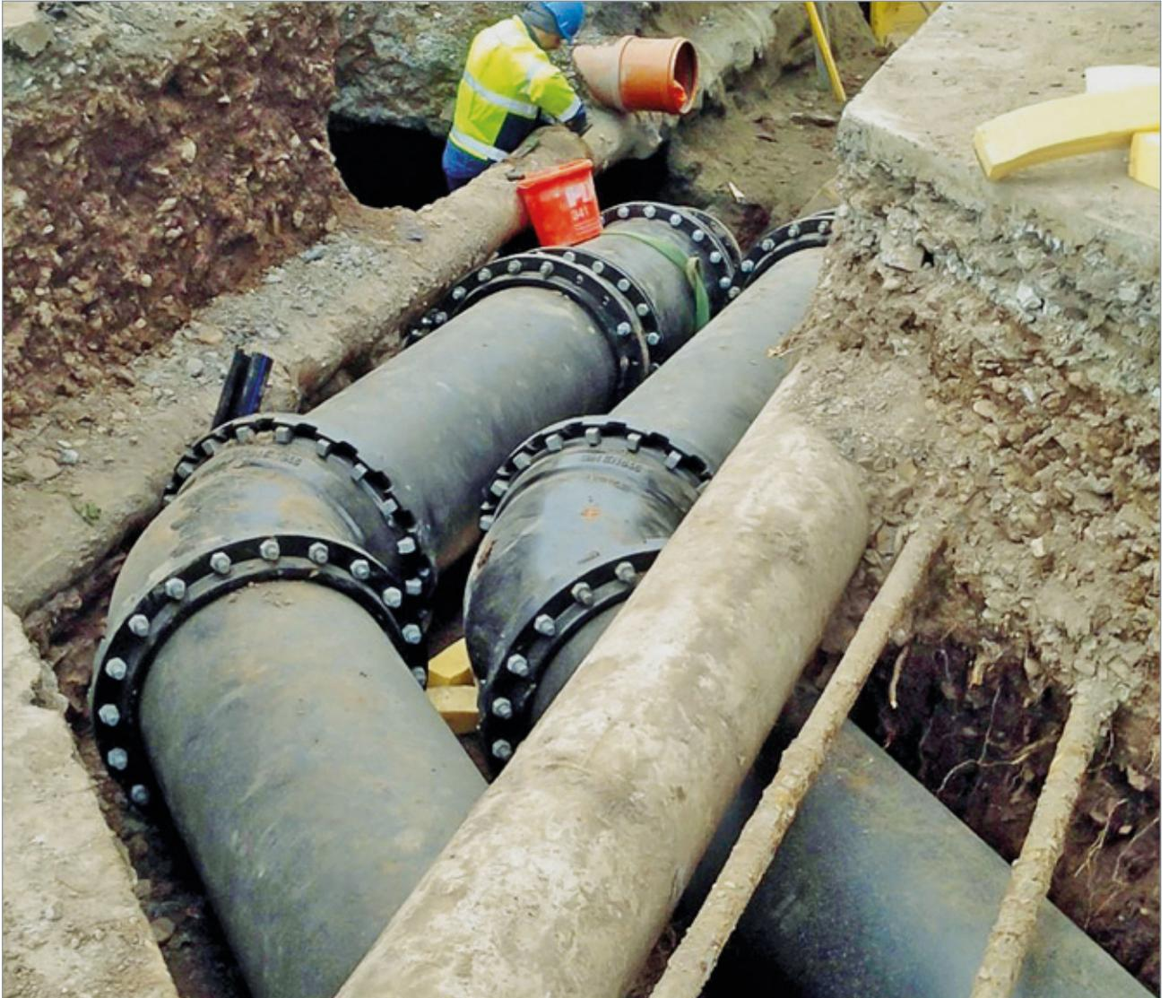
DUCPUR double DN 700 pipeline with feed and return flow.
