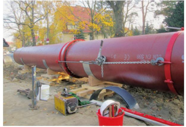
Assembled BLS® joint with pipe supports.
