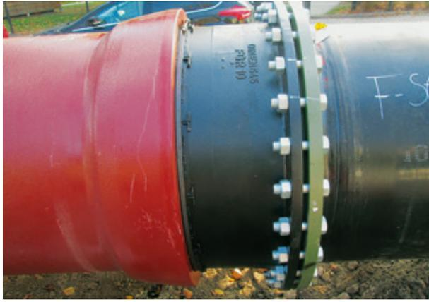
Flanged spigot assembled in the pipe socket using the BLS® system.
