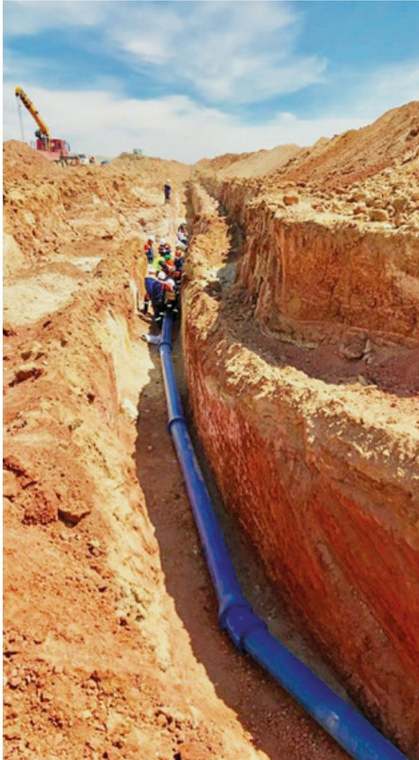
Temperatures as low as  $-40^{\circ}\text{C}$ , which prevail in the Mongolian winter and cause the ground to freeze to a depth of up to 3.5 m, make it necessary to lay the pipes 4 m deep.
